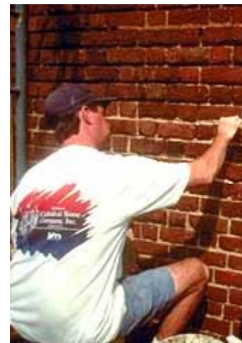
This early 19th century building is being repointed
