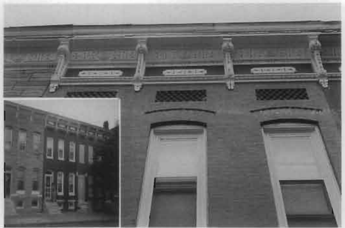
Figure 18. As part of an urban housing grant program, the exterior of this row house was successfully made lead-safe and met the Secretary of the Interior's Standards for Rehabilitation. The exterior was washed, then repainted with exterior grade alkyd paint. The decorative roof brackets and cornice were repainted; not removed or covered as is often recommended in typical abatement guidelines. The previously altered, deteriorated window sash were replaced with new sash and jamb liners set within the historic frames. Photos: Deborah Birch.
