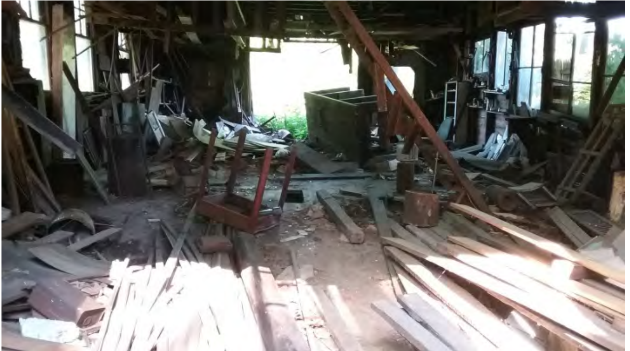
Barn Interior View
