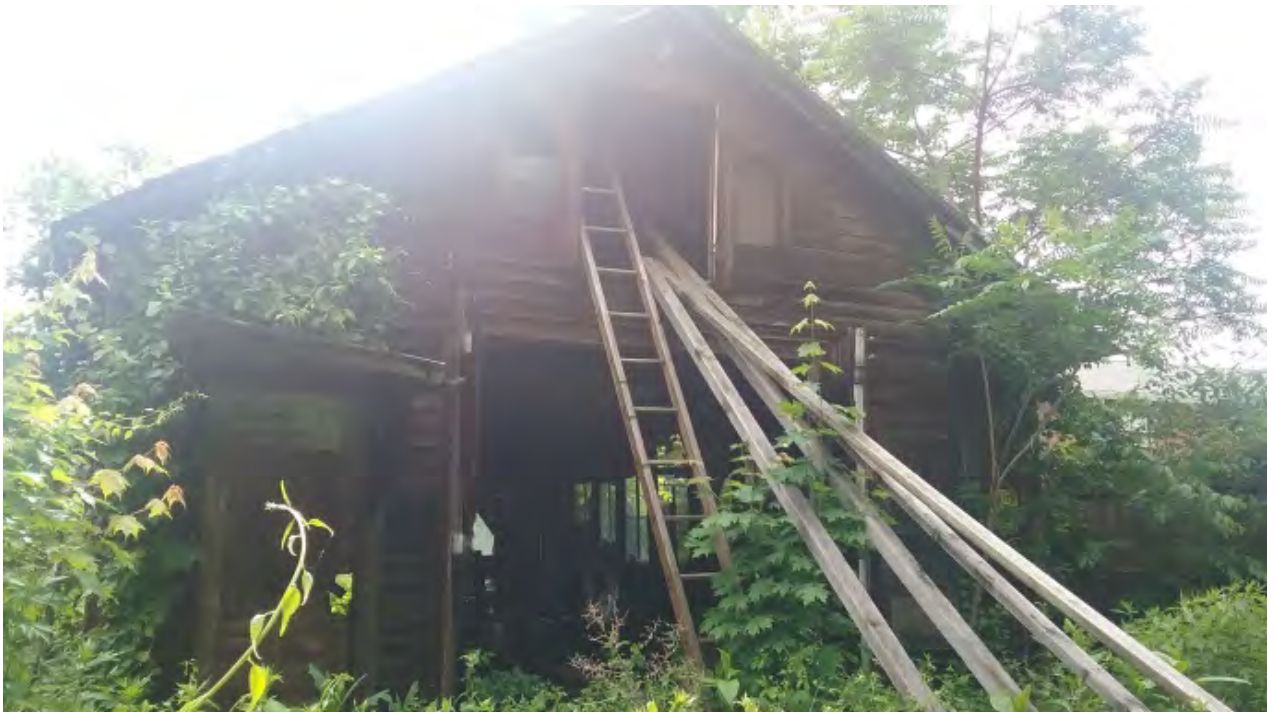
39 Chestnut Street Barn Front view
