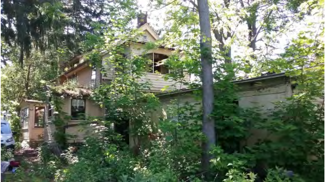
39 Chestnut Street House and Garage Back View
