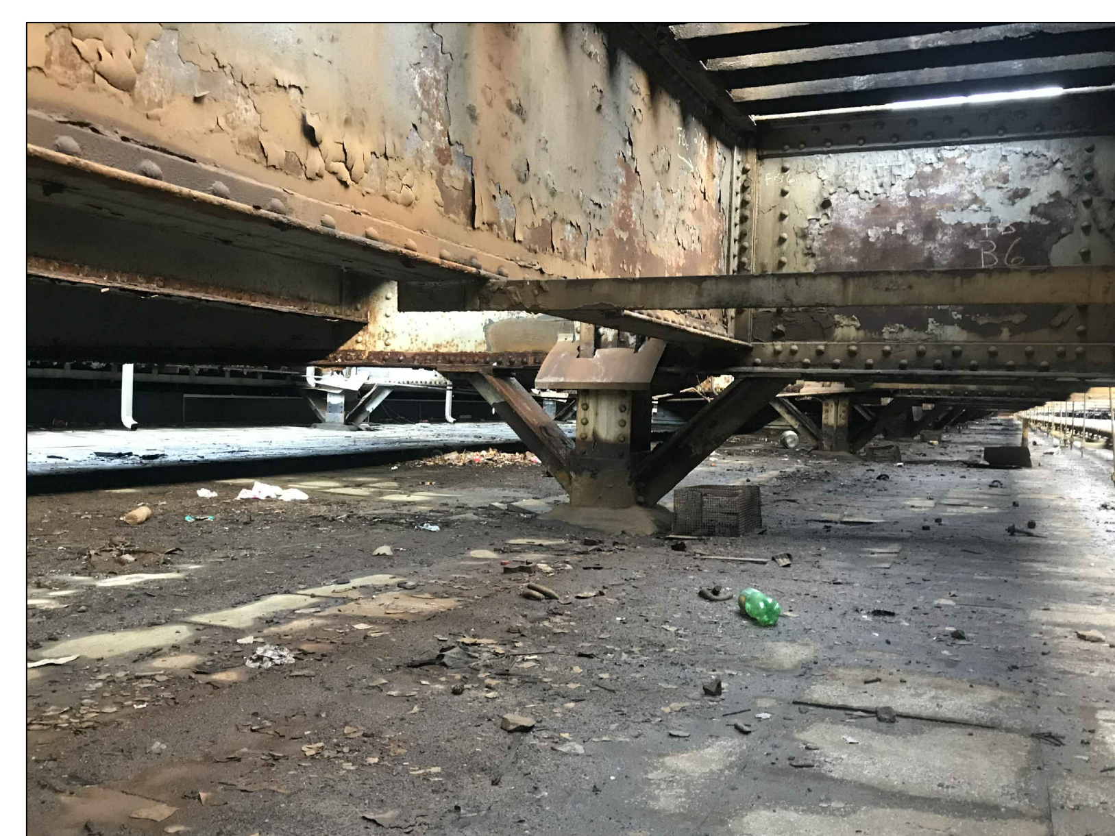
OVERVIEW OF ROOF SHOWING TYPICAL PENETRATIONS AND STRUCTURE OF TRAIN TRACKS ABOVE
