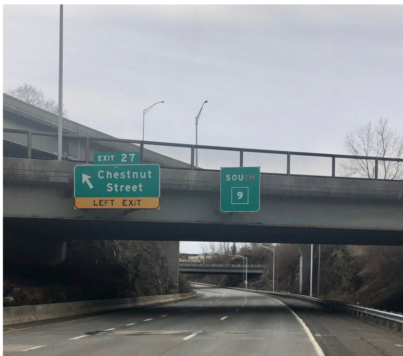
009S-088-36.08-A and 009S-088-36.08-B on 21065 (Bridge mount)
