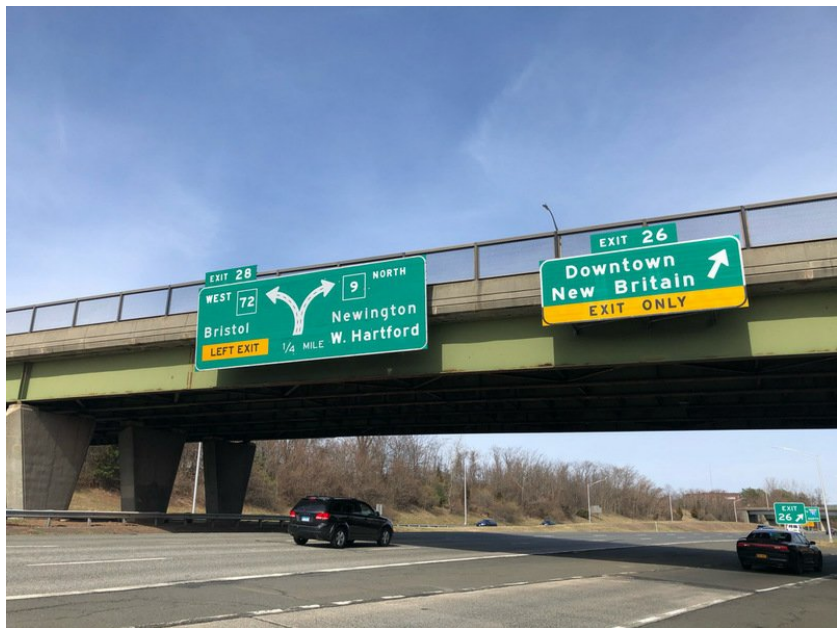
009N-088-35.35-A and 009N-088-35.35-B on bridge mount 21043
