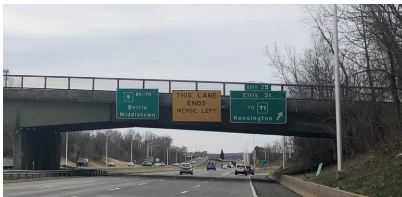
009S-088-35.14-A and 009S-088-35.14-B in 21070 (bridge mount)
