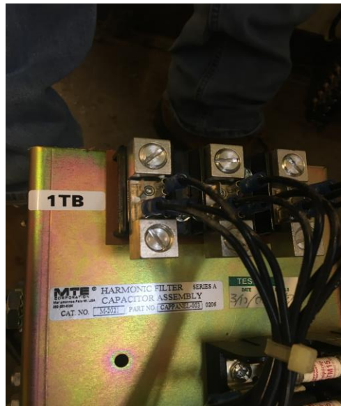
Harmonic Filter Capacitor Assembly MTE Corporation CAT. No. M-2021 Part No. CAPPANEL-003 Quantity: 3
