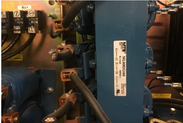
MTE Corporation No. ML0082G085 82A Max; 3 Phase Reactors; 600V Max. Part of the Filters shown above
