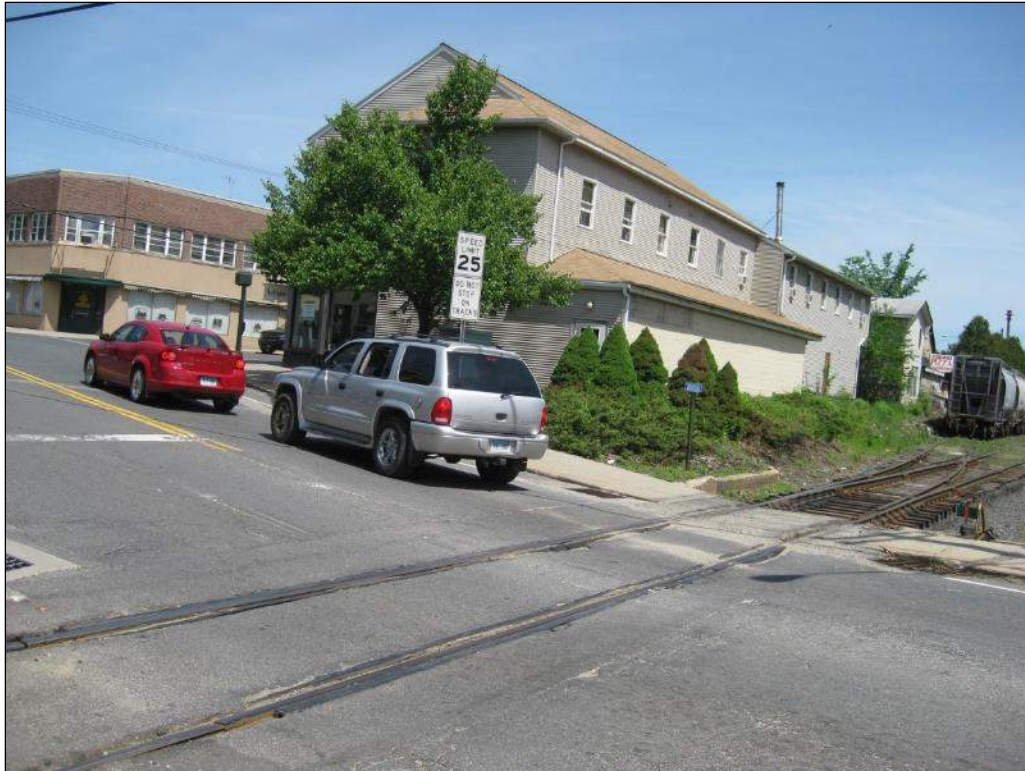
Photo No. 1 – Western crossing looking northwest
