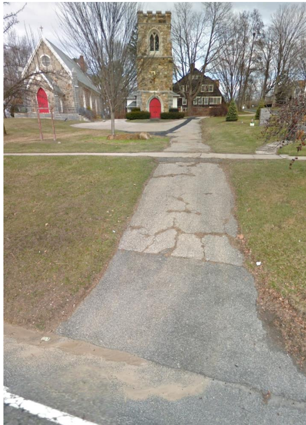
Image 4: Driveway that will be removed from 53 Main Street. In place of the existing asphalt, the path will be filled with topsoil the turf re-established. The existing concrete sidewalk will remain in place.
