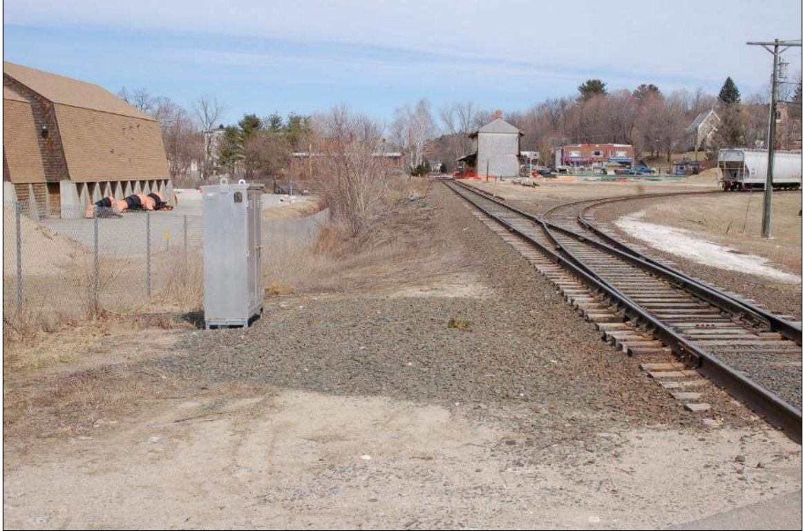
Photo No. 5 – Western drainage trunk looking north
