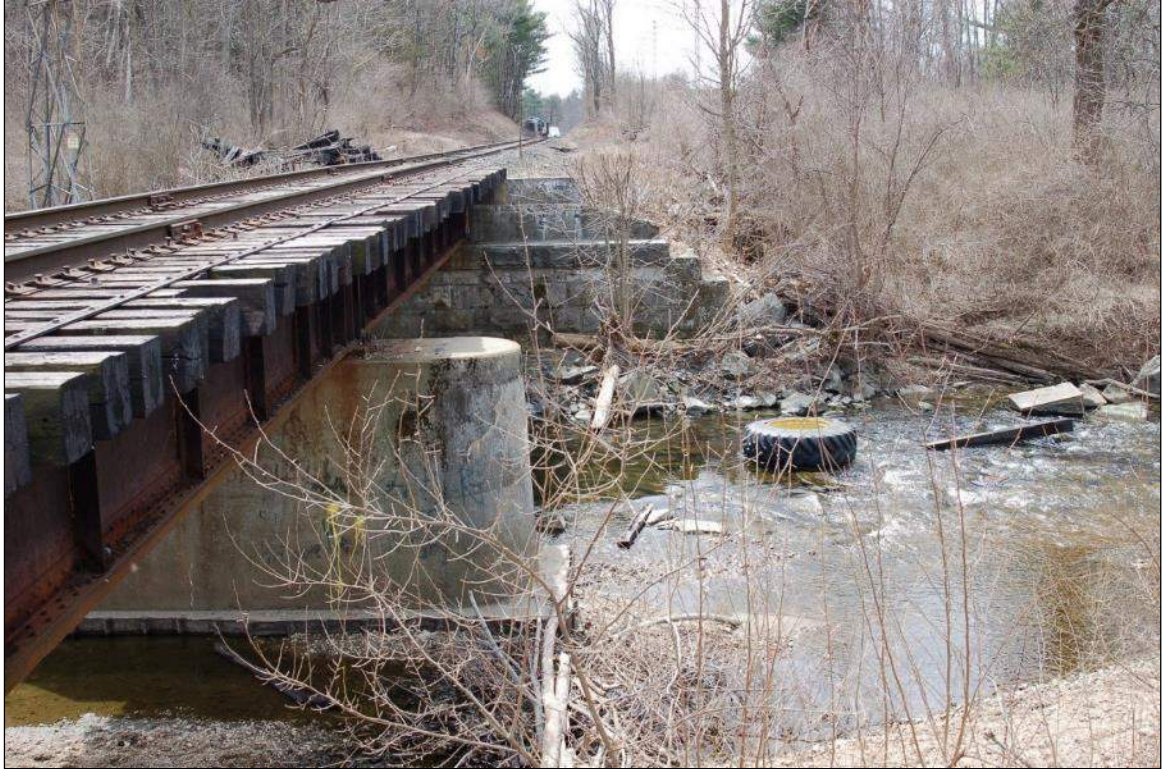
Photo No. 9 – Housatonic Railroad over Blackberry River
