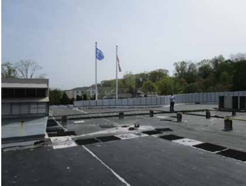
Photo 5/AD-102: Roof looking north.
