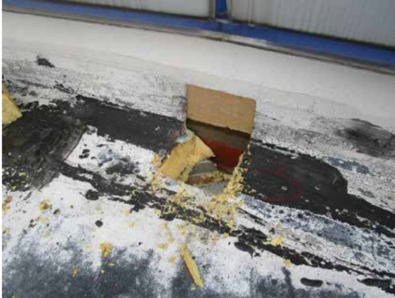
Photo 19/AD-102: Probe at north side of roof.
