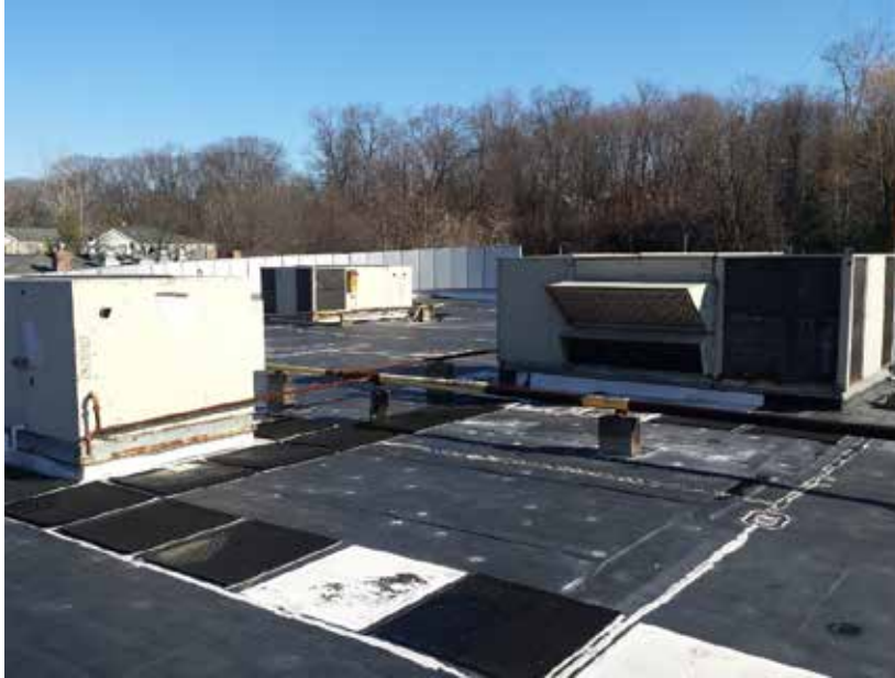
Photo 3/AD-102: Roof looking northeast.
