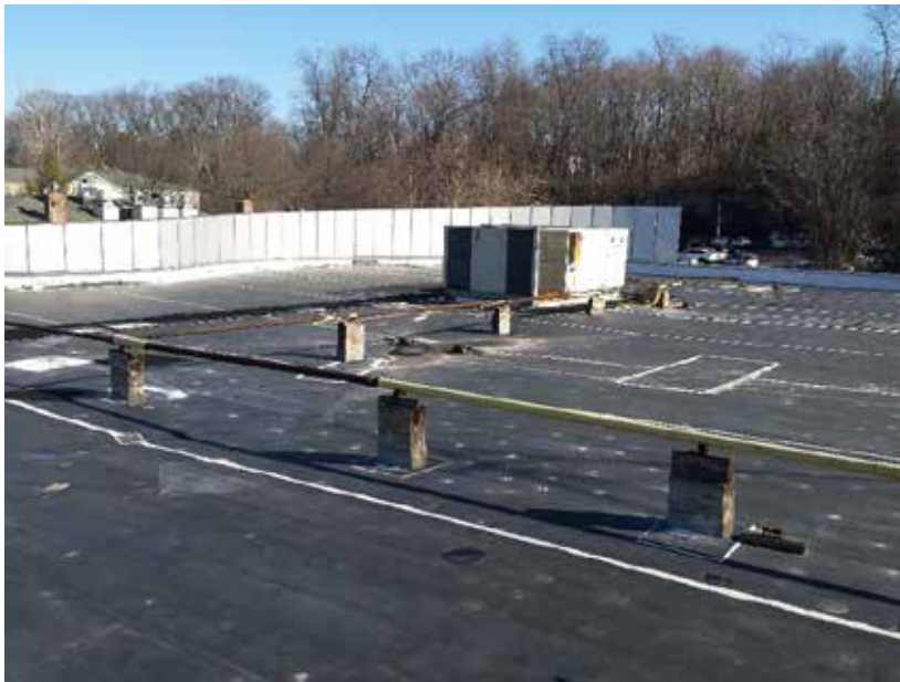
Photo 2/AD-102: Roof looking at northeast corner.
