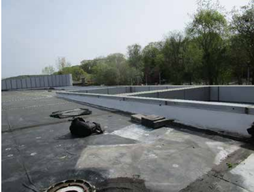
Photo 7/AD-102: Roof looking at northeast corner.
