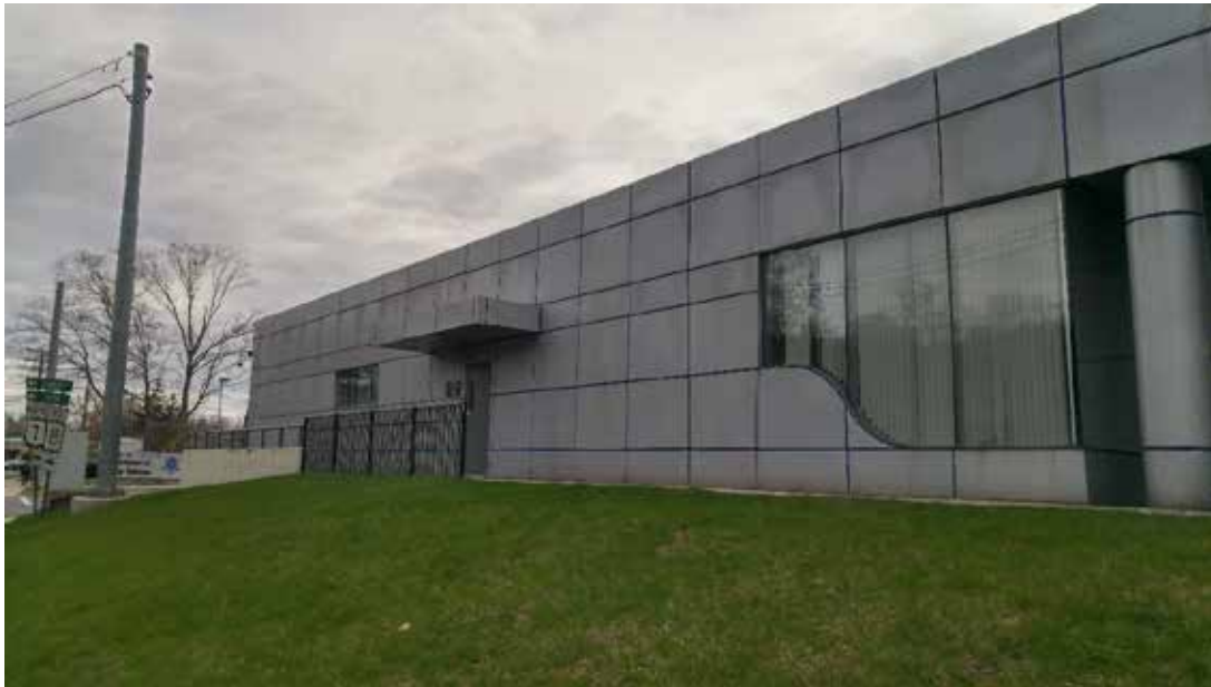
Photo 6/AD-100: West Elevation.
