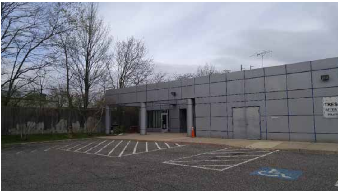
Photo 3/AD-100: Partial East Elevation.
