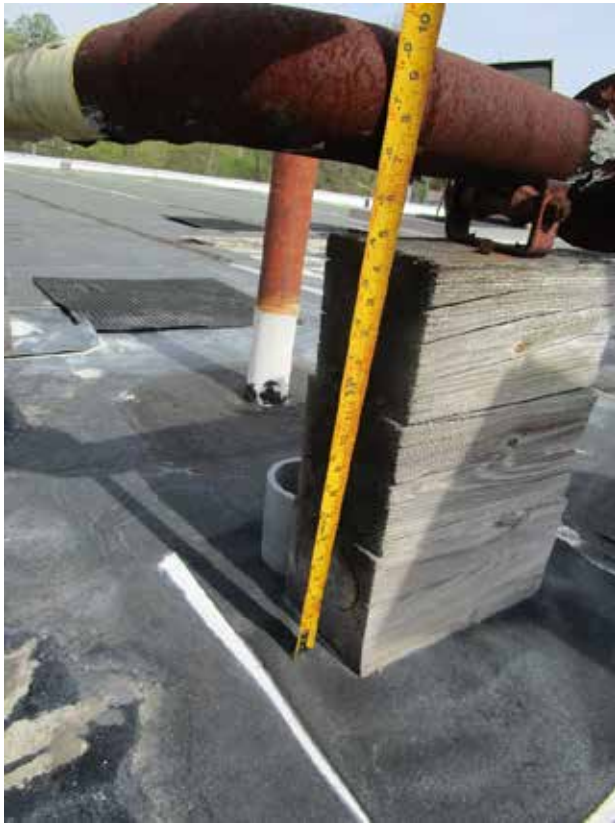
Photo 9/AD-102: Typical existing pipe support.
