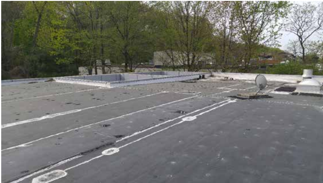
Photo 6/AD-102: Roof looking at southeast corner.
