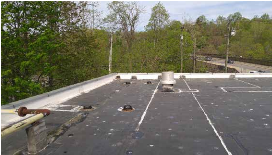
Photo 11/AD-102: Roof looking at southwest corner.
