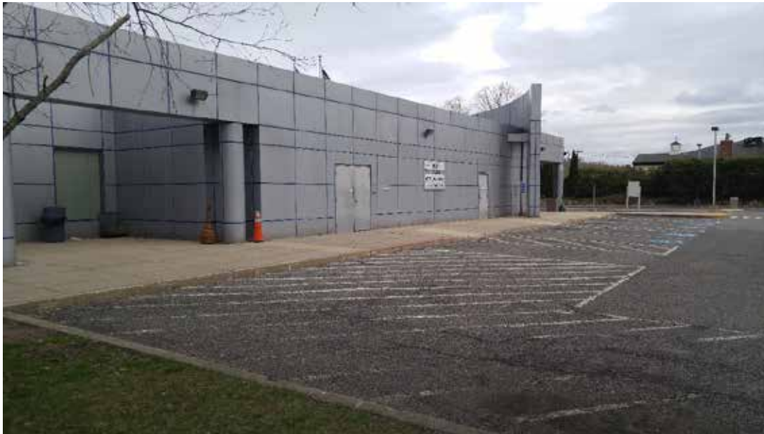
Photo 5/AD-100: Lay down and storage area at east side of building.
