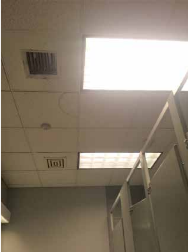
Photo 6/A-101: Public Men's Room.
