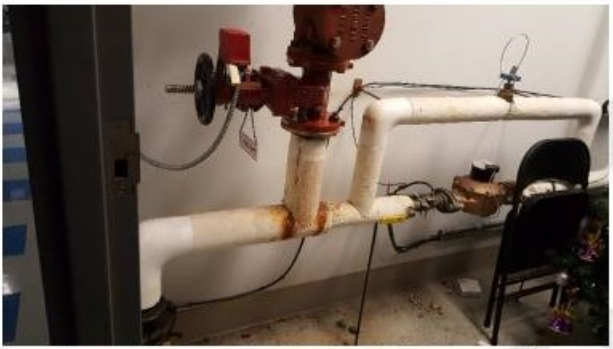
Figure 17: Incoming Domestic Water Service
