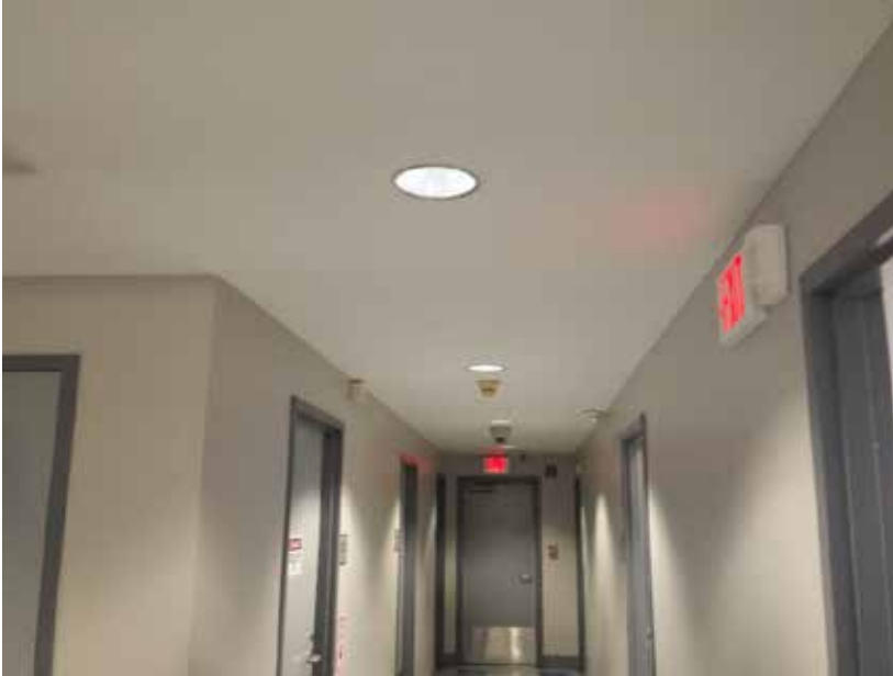
Photo 10/AD-101: Southwest exit corridor.
