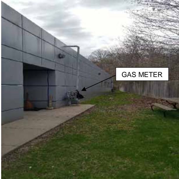
Photo 4/AD-100: South Elevation.
