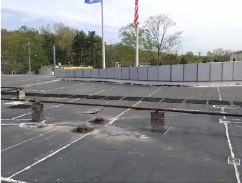
Photo 13/AD-102: Roof looking north.
