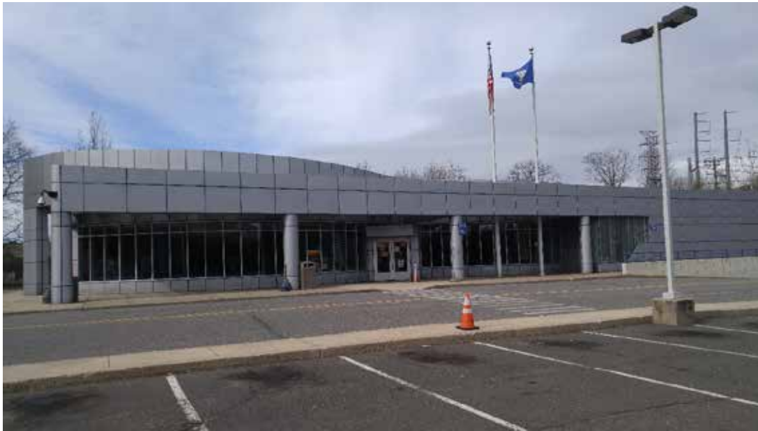
Photo 2/AD-100: North Elevation.
