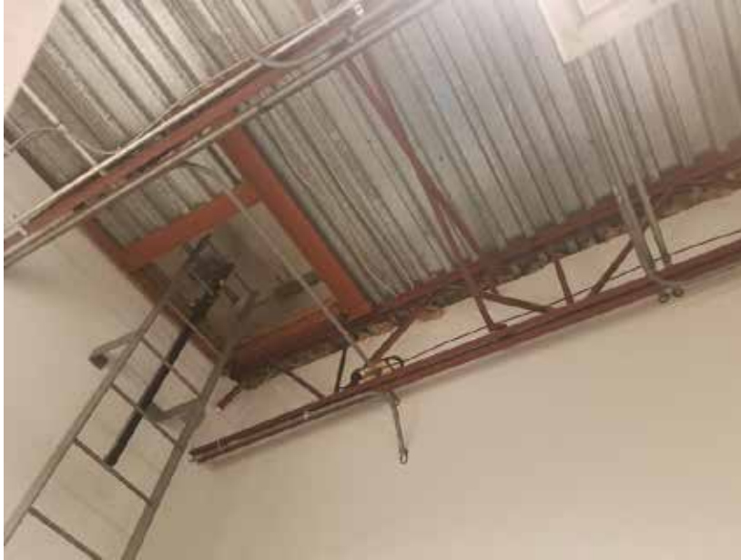
Photo 2/AD-101: Ladder to roof hatch.
