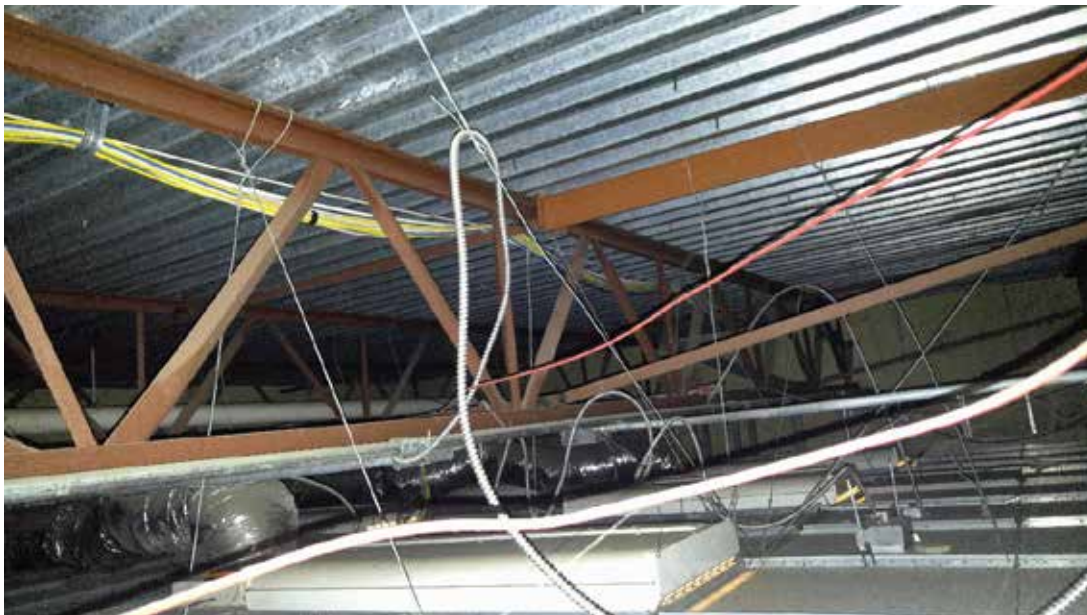
Photo 3/AD101: Typical conditions above ceiling.
