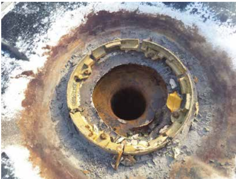
Photo 22/AD-102: Existing roof drain clamping ring.
