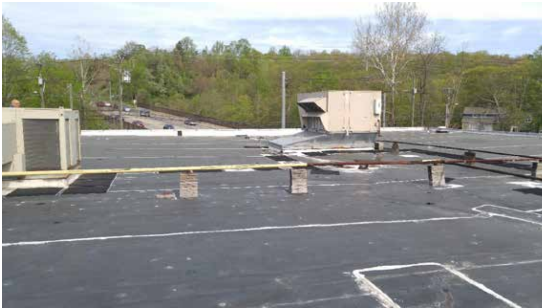
Photo 18/AD-102: Roof looking west.
