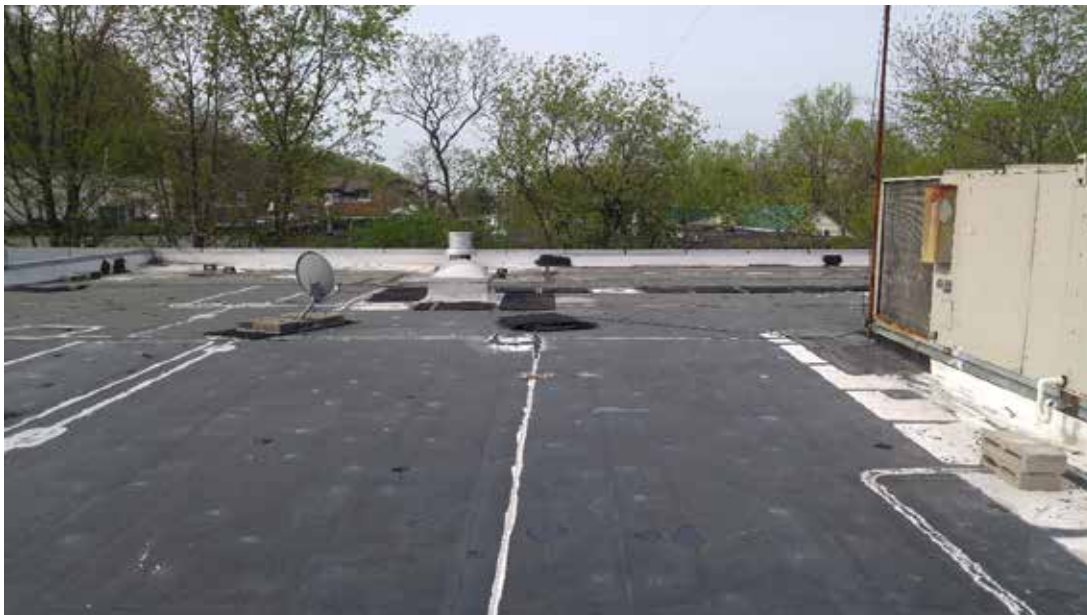
Photo 12/AD-102: Roof looking south.
