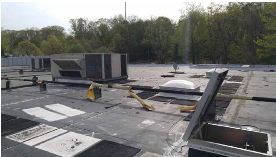
Photo 10/AD-102: Roof looking east.
