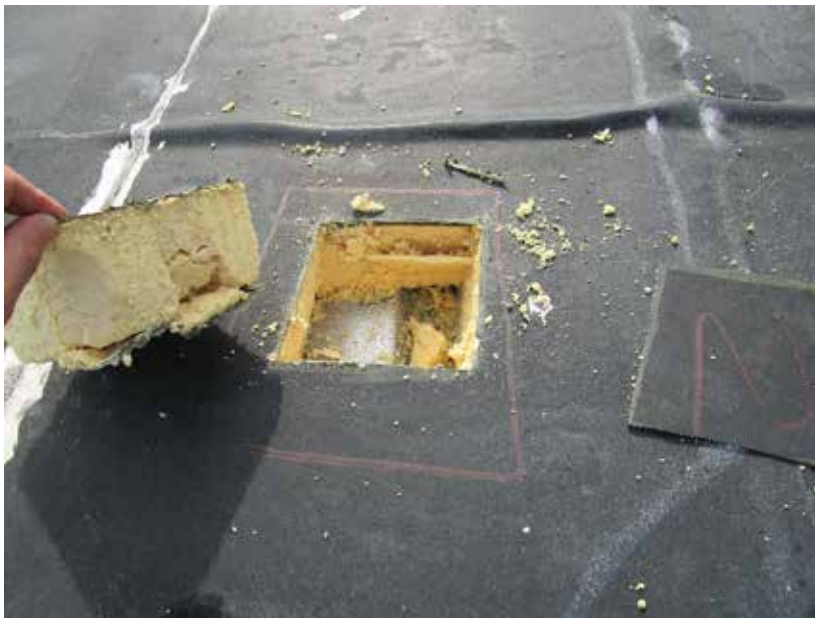
Photo 20/AD-102: Probe at field of roof.
