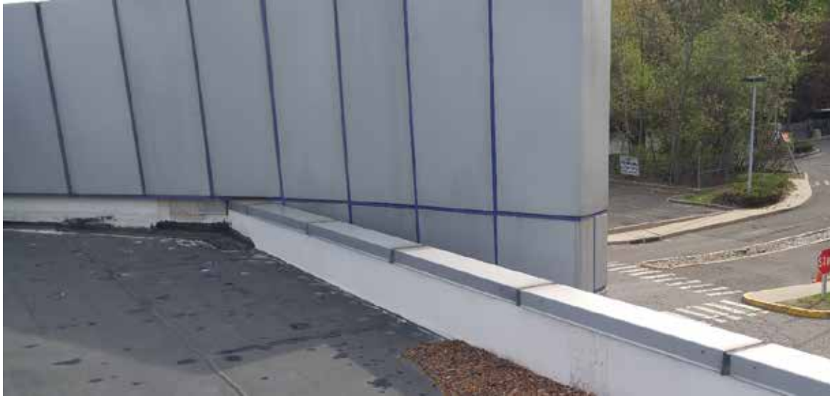
Photo 17/AD-102: East end of metal panel parapet.
