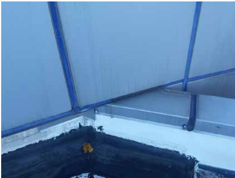
Photo 16/AD-102: Roof edge at east side of parapet.
