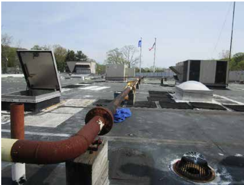
Photo 8/AD-102: Roof looking north.
