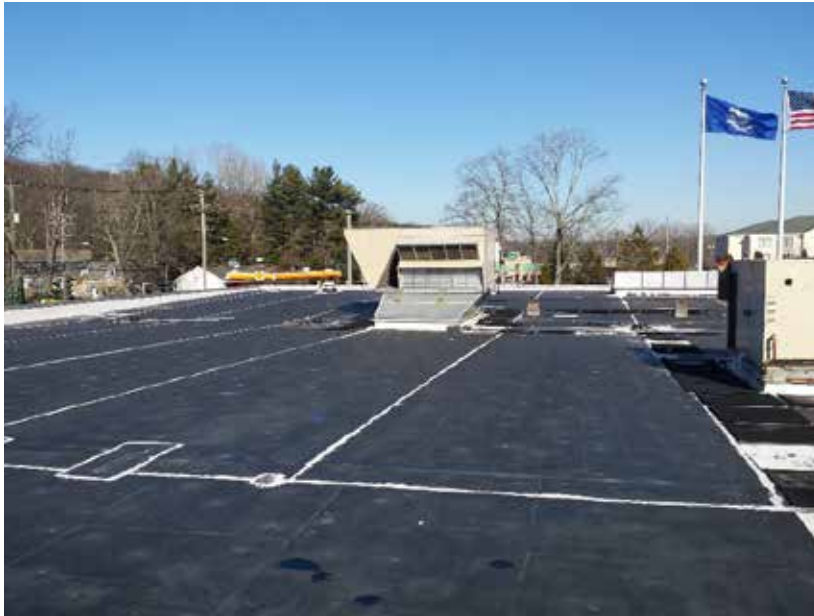
Photo 1/AD-102: Roof looking at northeast corner.
