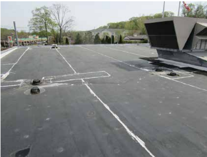
Photo 14/AD-102: Roof looking at northwest corner.
