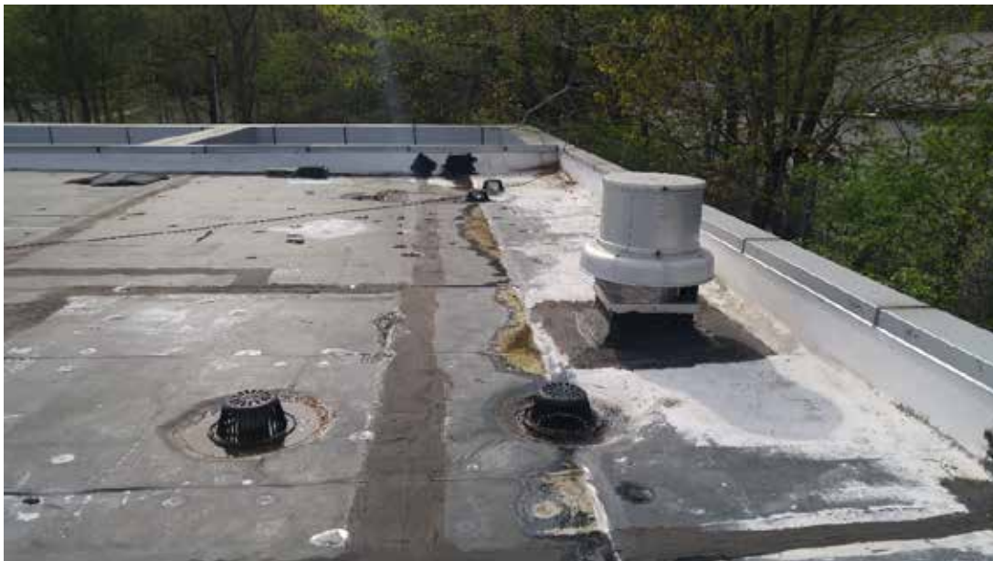
Photo 4/AD-102: Roof looking at southeast corner.
