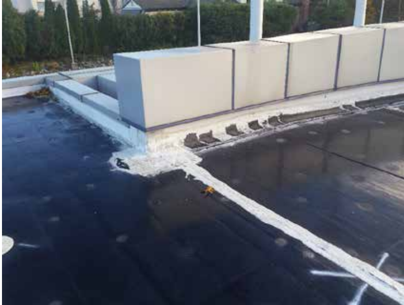
Photo 15/AD-102: West end of metal panel parapet.
