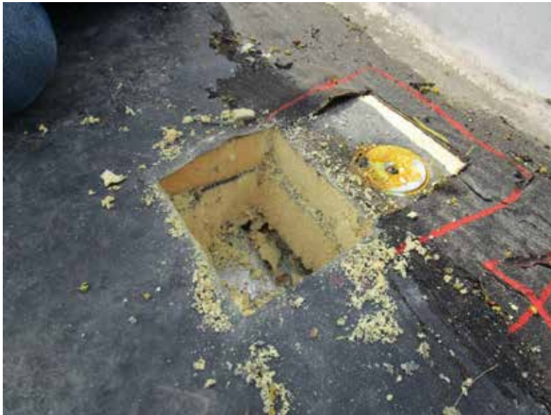
Photo 21/AD-102: Probe at south side of roof.
