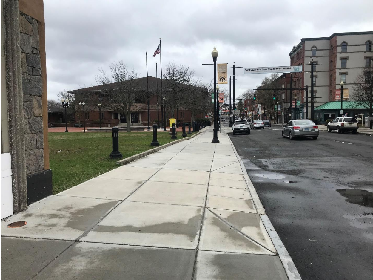
On Street Parking View #1, before bump-out
