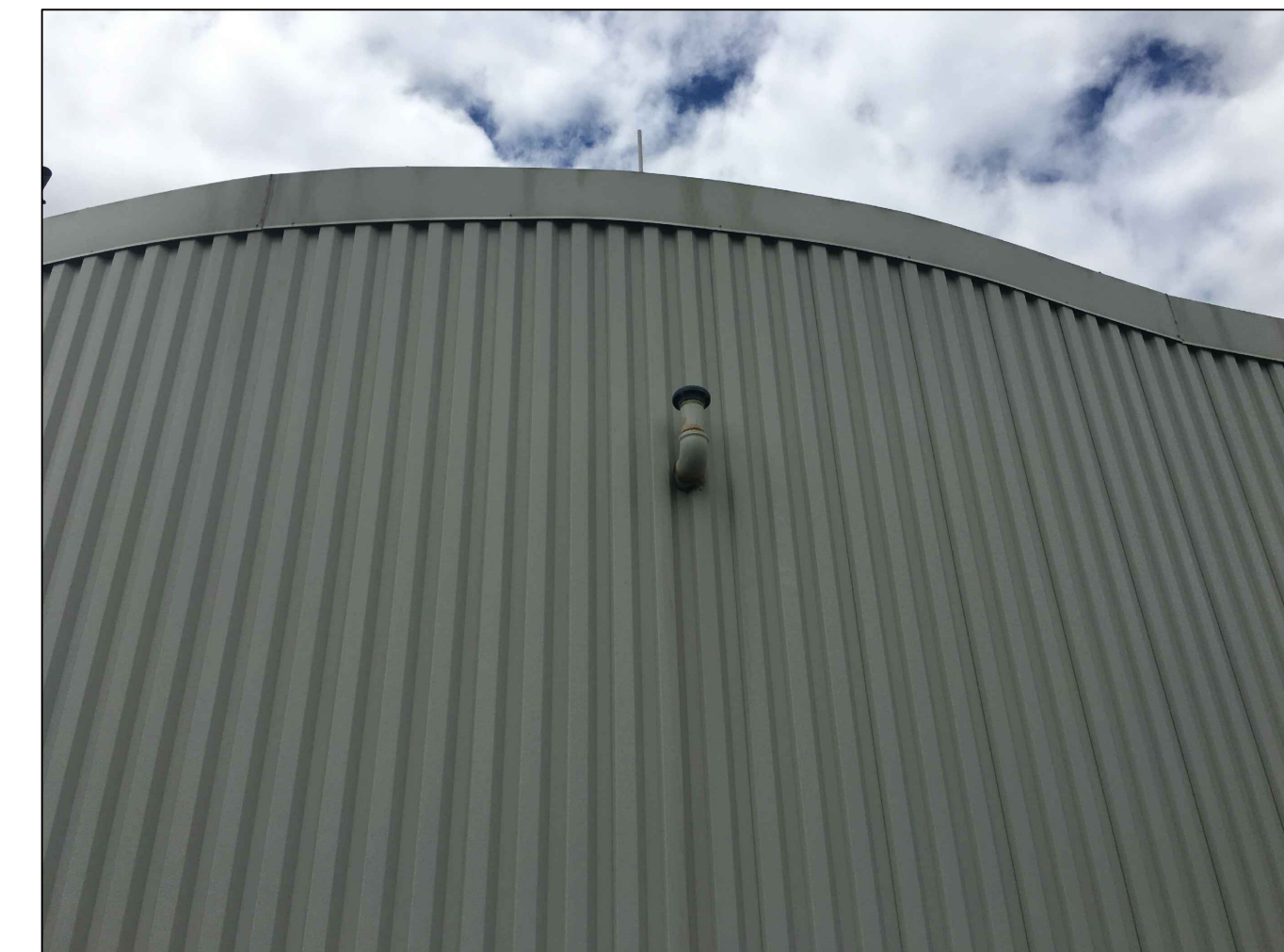
8 PENTHOUSE: REMOVE VENT AND PERMANENTLY CAP
