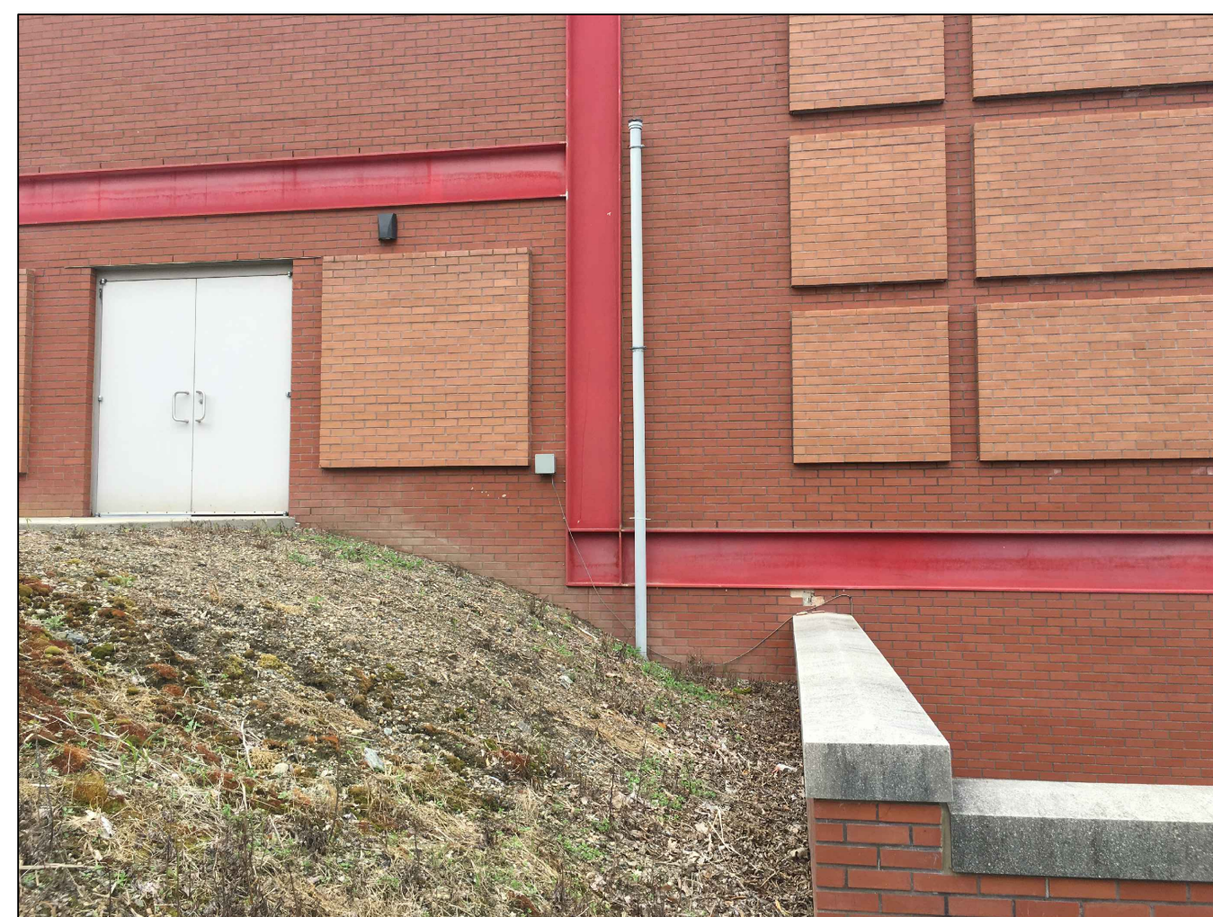
7 REMOVE VENT & CAP BELOW GRADE
