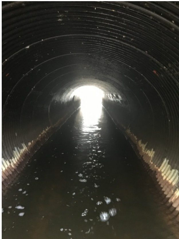
East side looking westward
