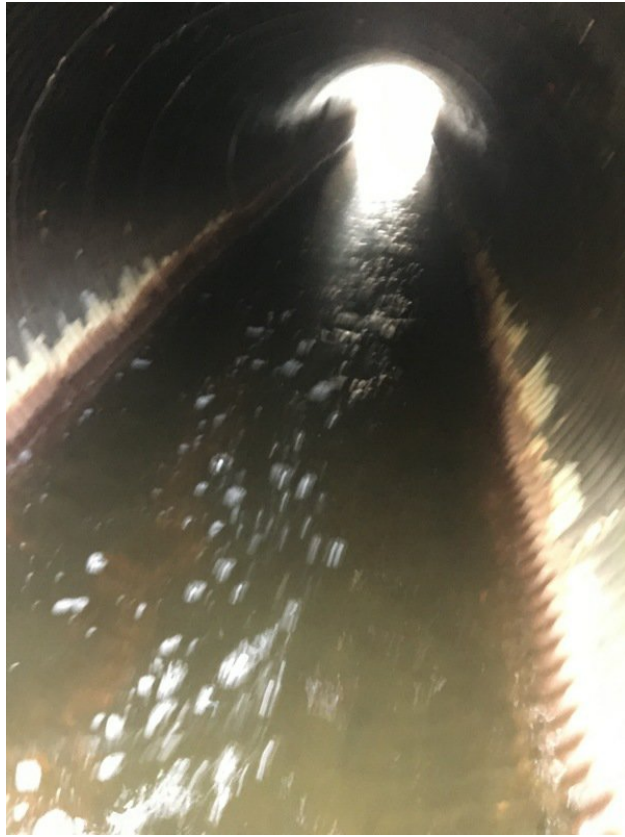
East side looking westward
