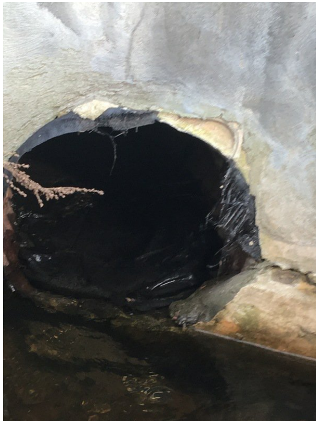
18 inch pipe on west side with fiber lining
