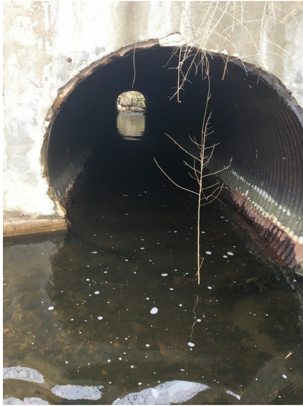
West side of culvert
