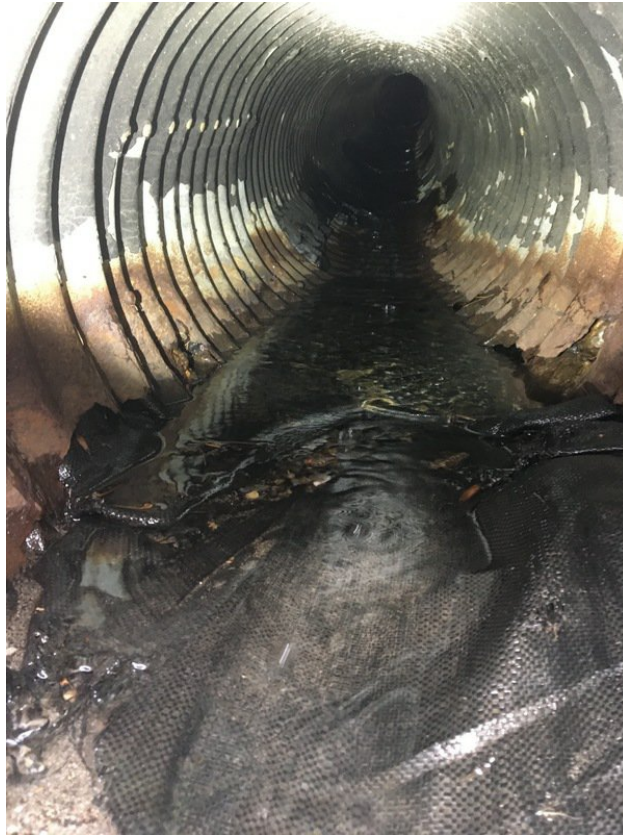
18 inch pipe on west side
