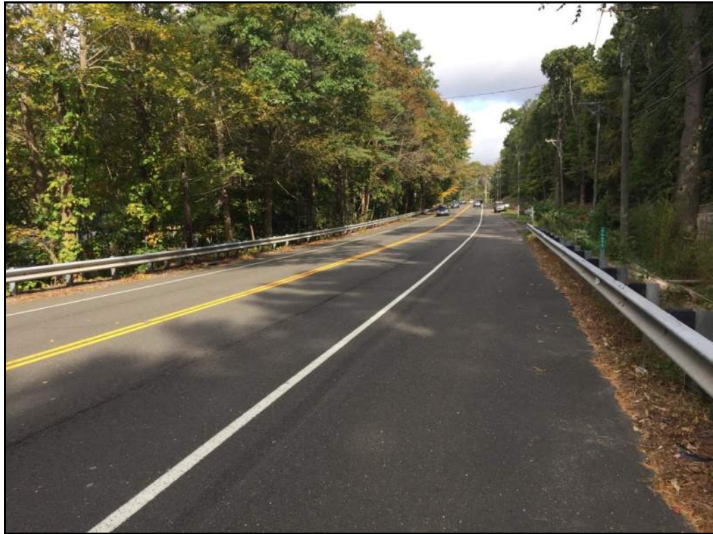
Photo No. 5 – Bridge from South Approach
