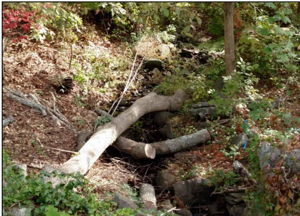
Photo No. 6 – Upstream from Bridge (Overflow Spillway)
