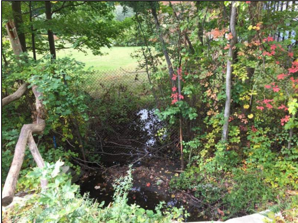
Photo No. 7 – Downstream from Bridge
