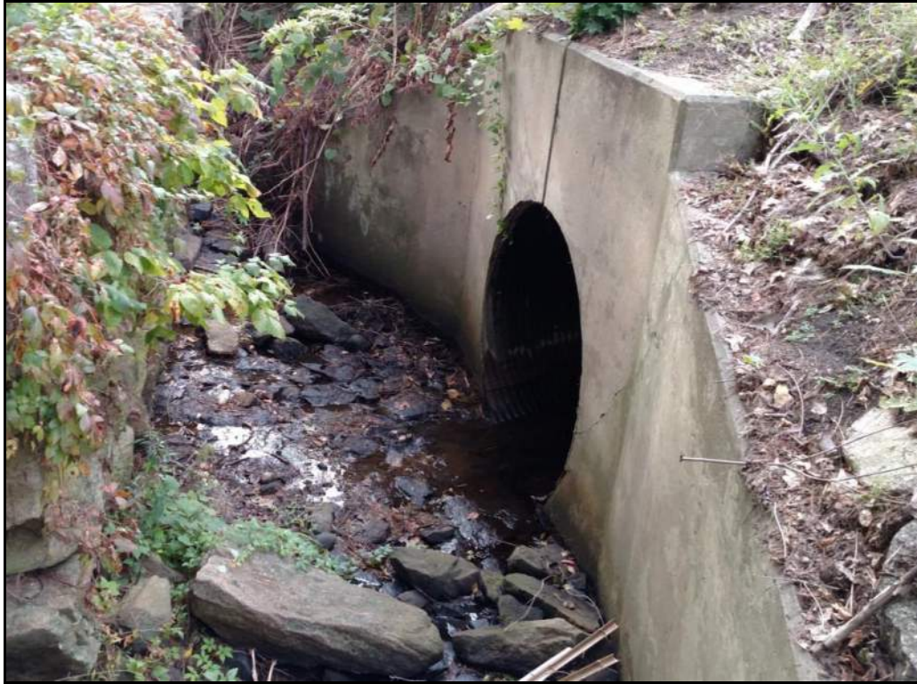
Photo No. 11 – South East Wingwall
