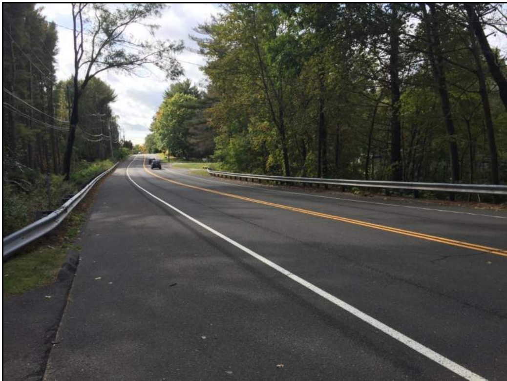
Photo No. 4 – Bridge from North Approach
