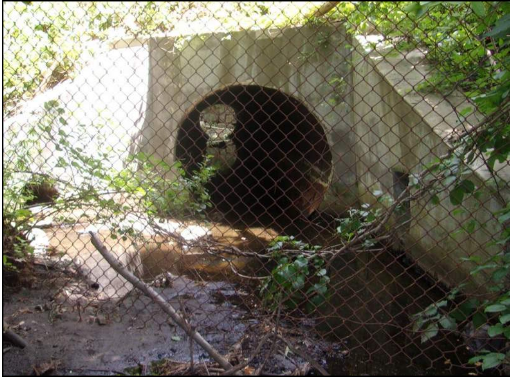
Photo No. 3 – West Elevation
