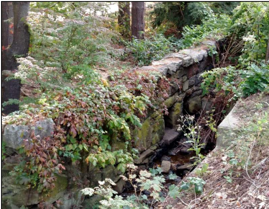
Photo No. 12 – Masonry Wall opposite East Elevation
