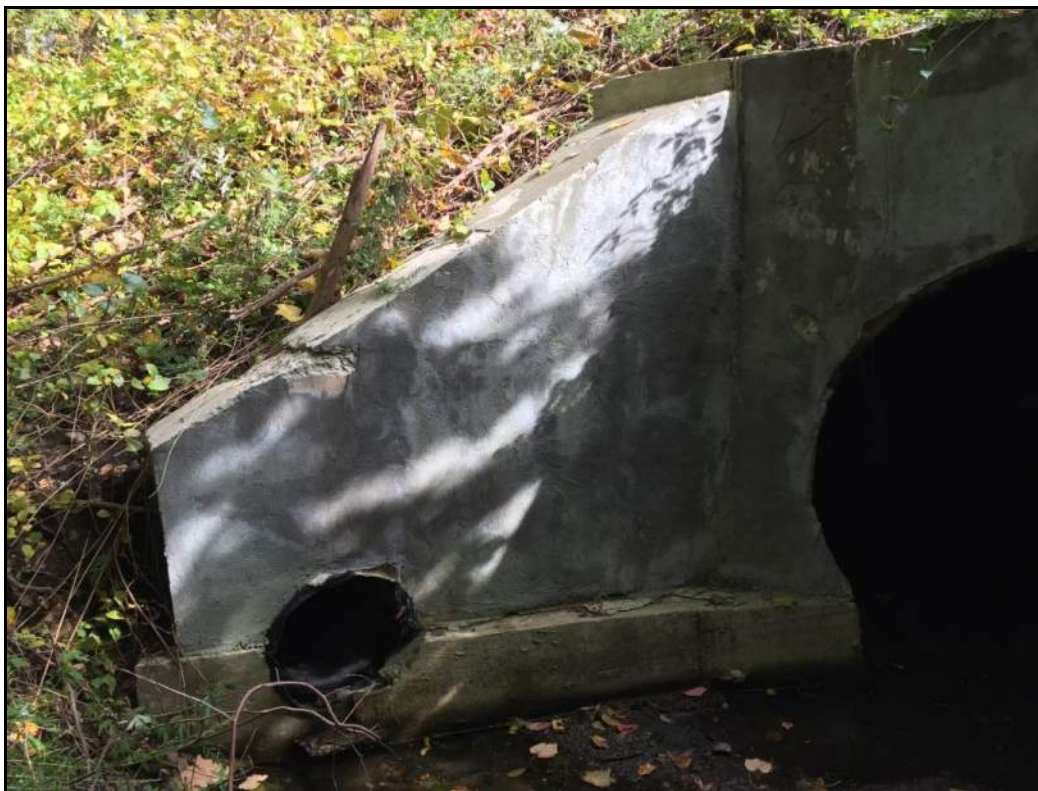
Photo No. 8 – North West Wingwall
