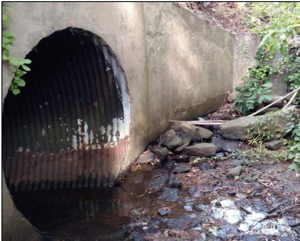
Photo No. 10 – North East Wingwall
