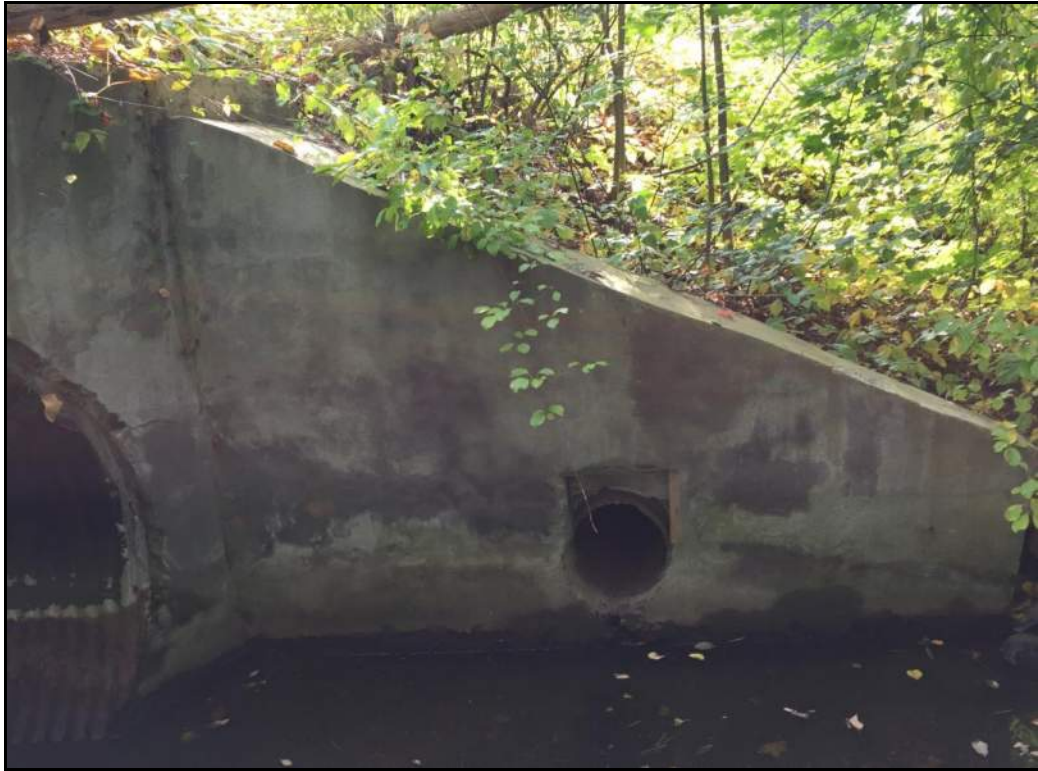
Photo No. 9 – South West Wingwall
