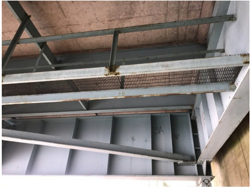
Westbound bridge facing east
