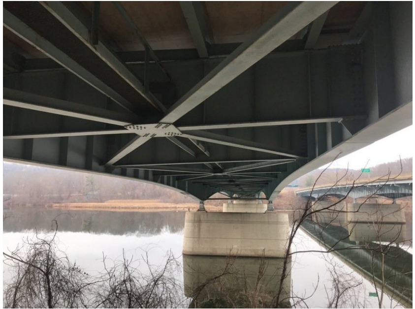
Westbound bridge facing north
