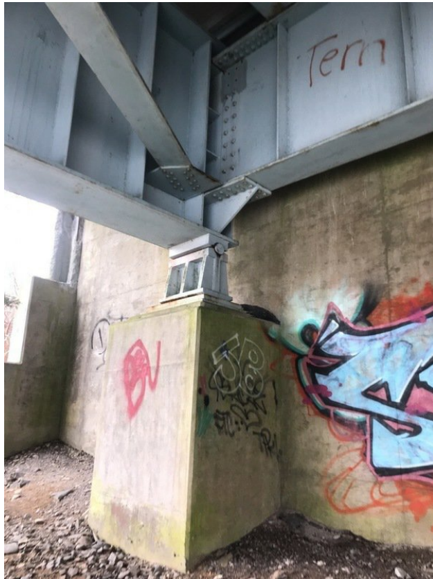
Westbound bridge facing east
