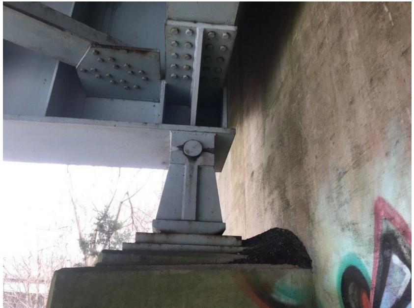
Westbound bridge facing east
