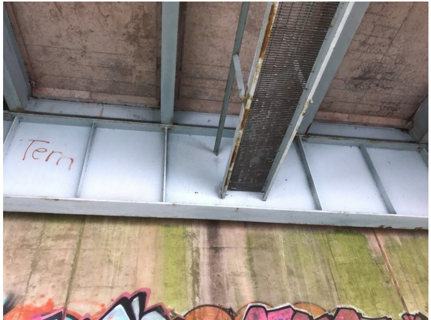
Westbound bridge facing south
