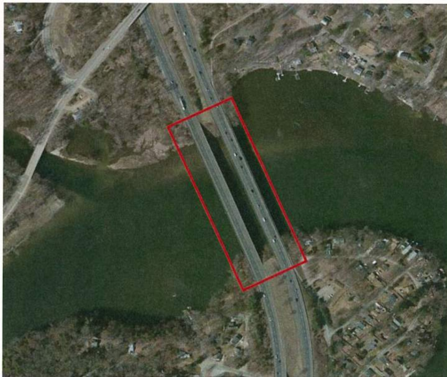
Aerial photo of Bridge Nos. 01218 & 04180 and immediate surroundings
