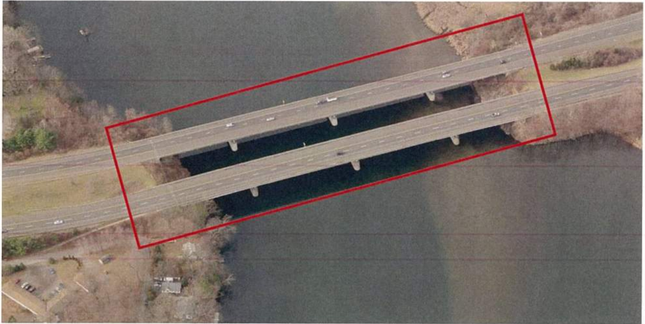
Birdseye aerial of Bridge Nos. 01218 & 04180 I-84 EB and I-84 WB over the Housatonic River looking westward (BingMaps)
