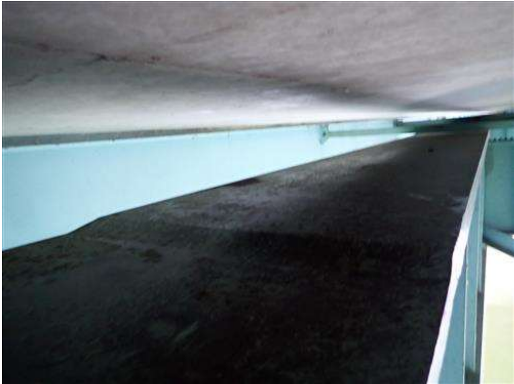
Girder 1 Top Flange Transition at Floor Beam 2 (Typical)
