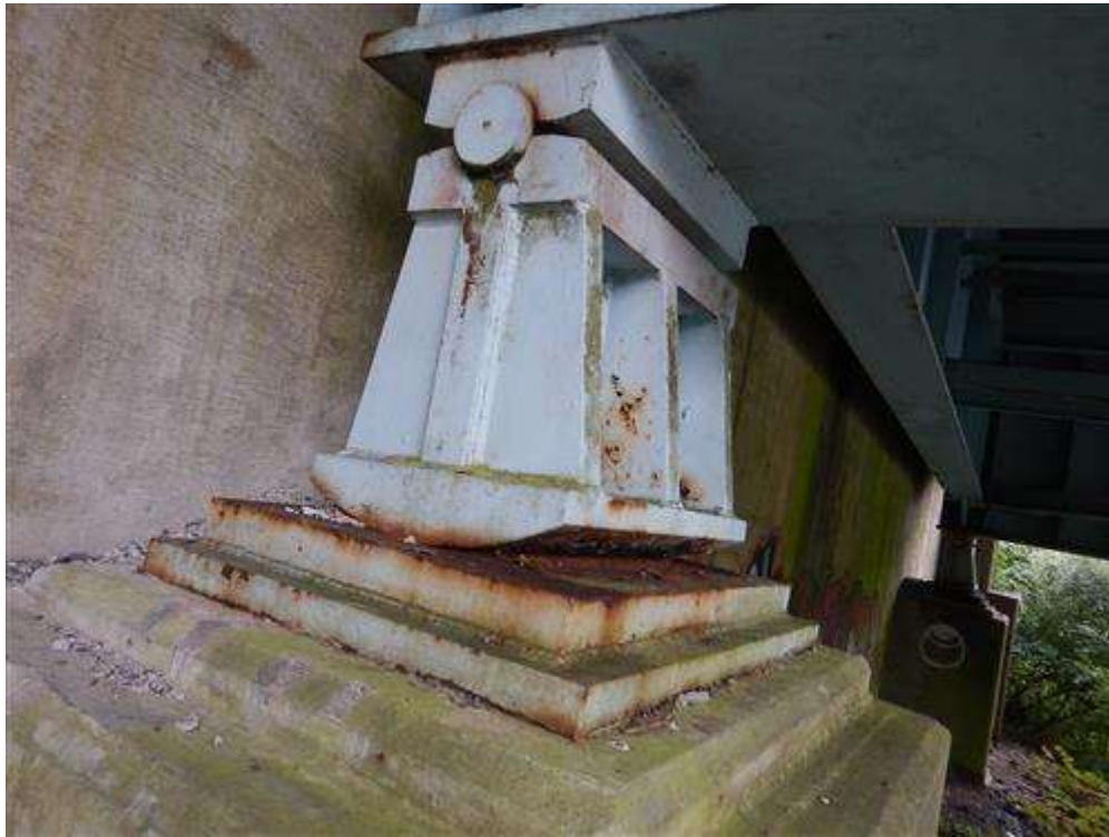
Girder 1 Rocker Bearing at Abutment 1
