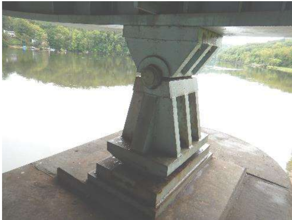
Girder 1 Bearing at Pier 3
