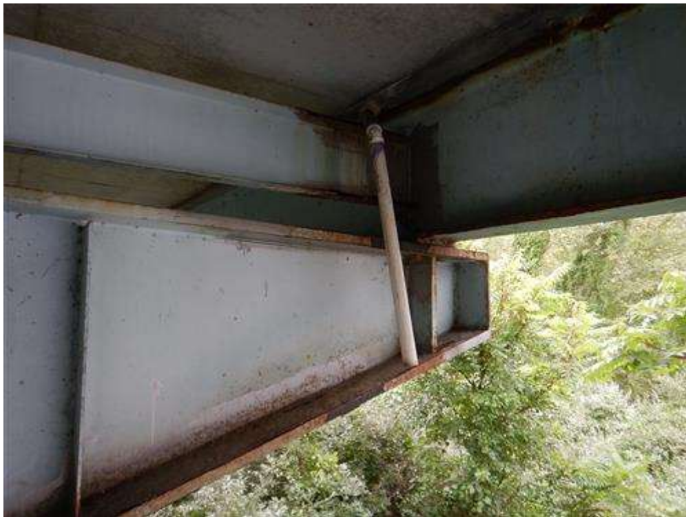
Weep Drain Adjacent to Floor Beam 2 and Stringer 1
