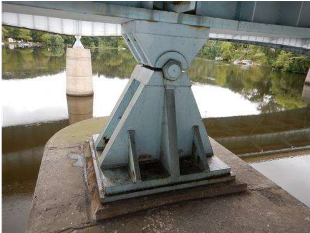
Girder 2 Fixed Bearing at Pier 2
