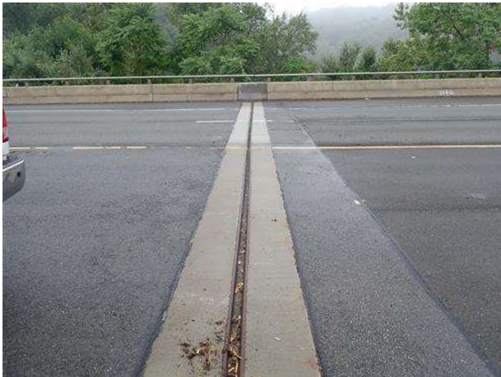
Abutment 1 Strip Seal Joint
