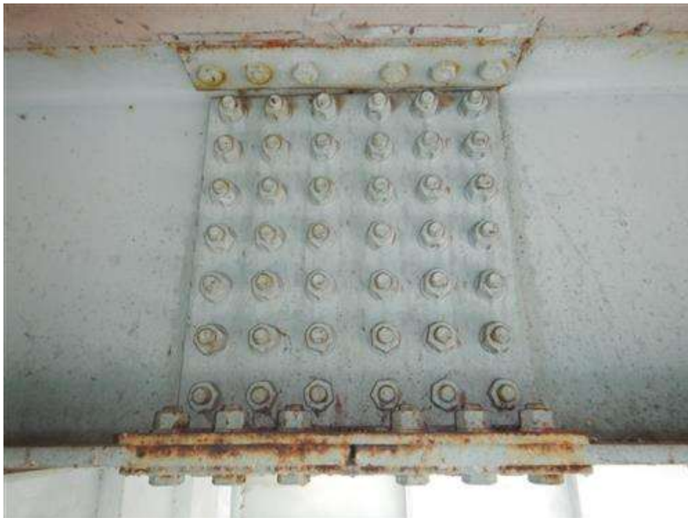
Stringer Field Splice (Typical)
