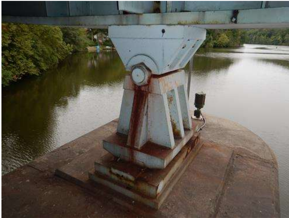
Girder 1 Rocker Bearing at Pier 1
