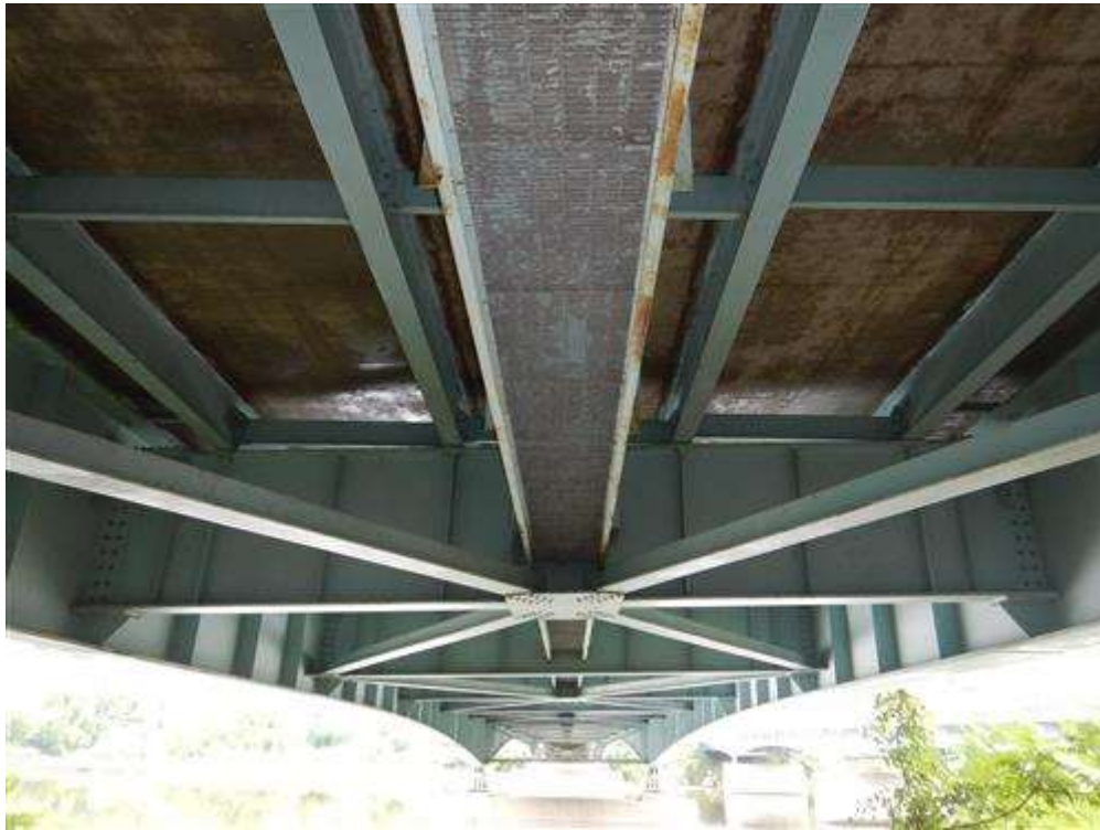
Floor Beam (Typical)
