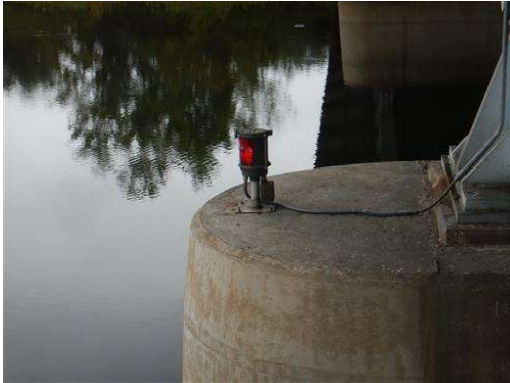
Pier 2 Navigation Light (Typical)
