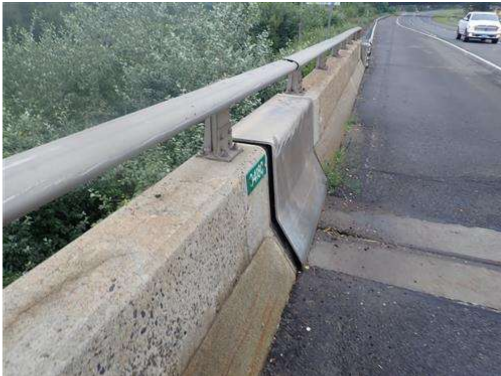
Left Parapet Sliding Metal Plate at Abutment 2
