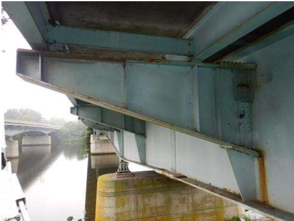
Floor Beam 25 Cantilever at Girder 2 (Typical)
