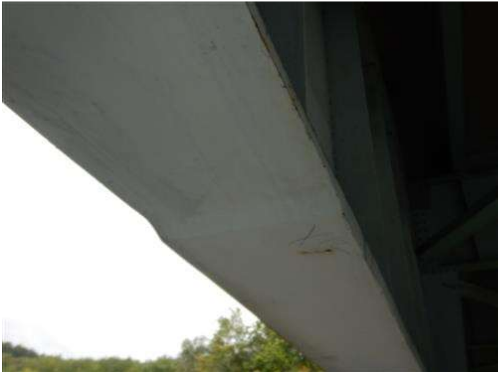
Girder Bottom Flange Transition (Typical)
