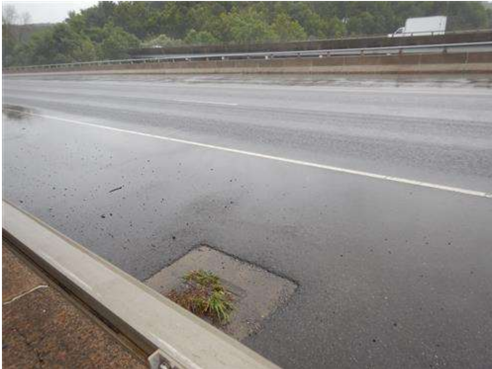
Span 1 Bituminous Concrete Overlay, Looking Southwest
