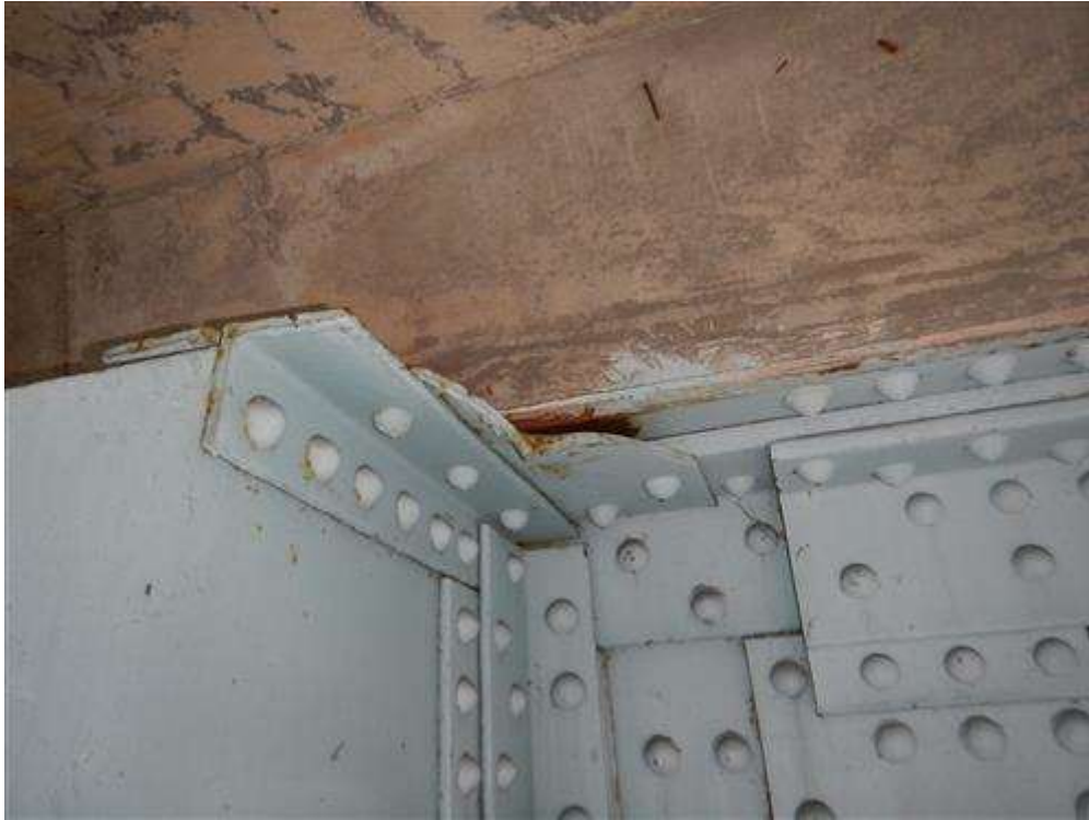
Floor Beam 6 Connection to Girder 2
