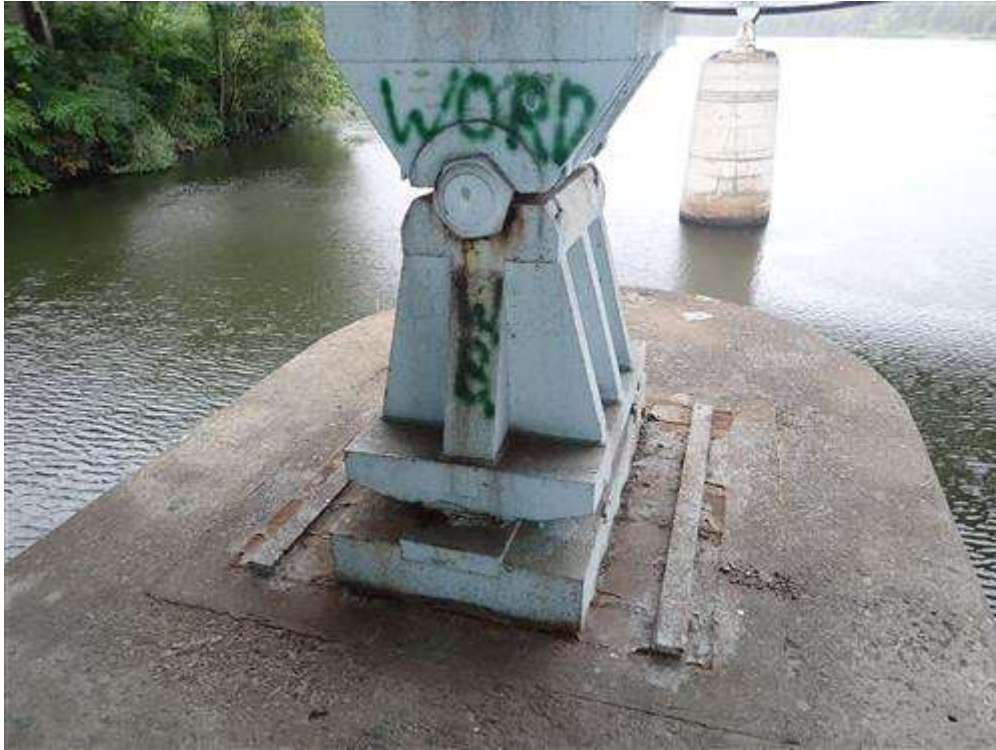
Girder 1 Rocker Bearing at Pier 1
