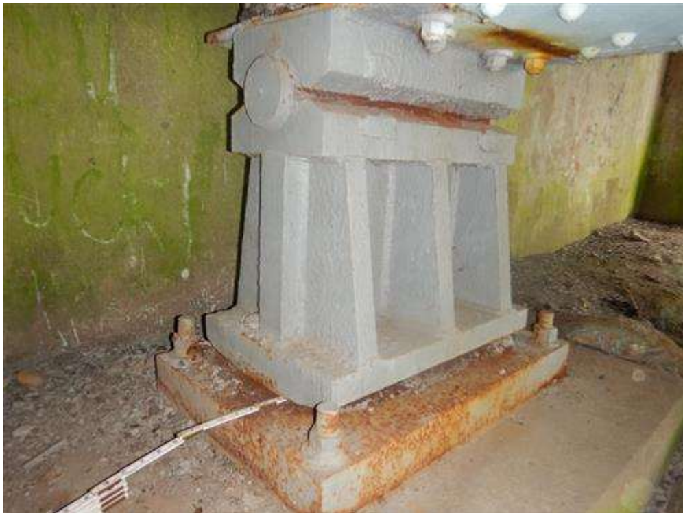
Girder 1 Rocker Bearing at Abutment 1
