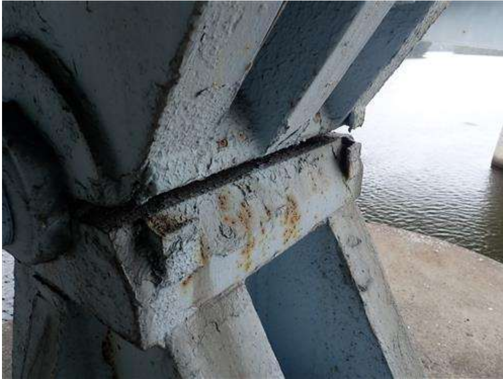
Brackets Torch Cut Off Bearings
