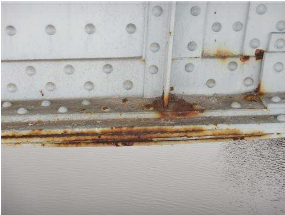
Girder 1 West Face at Floor Beam 6
