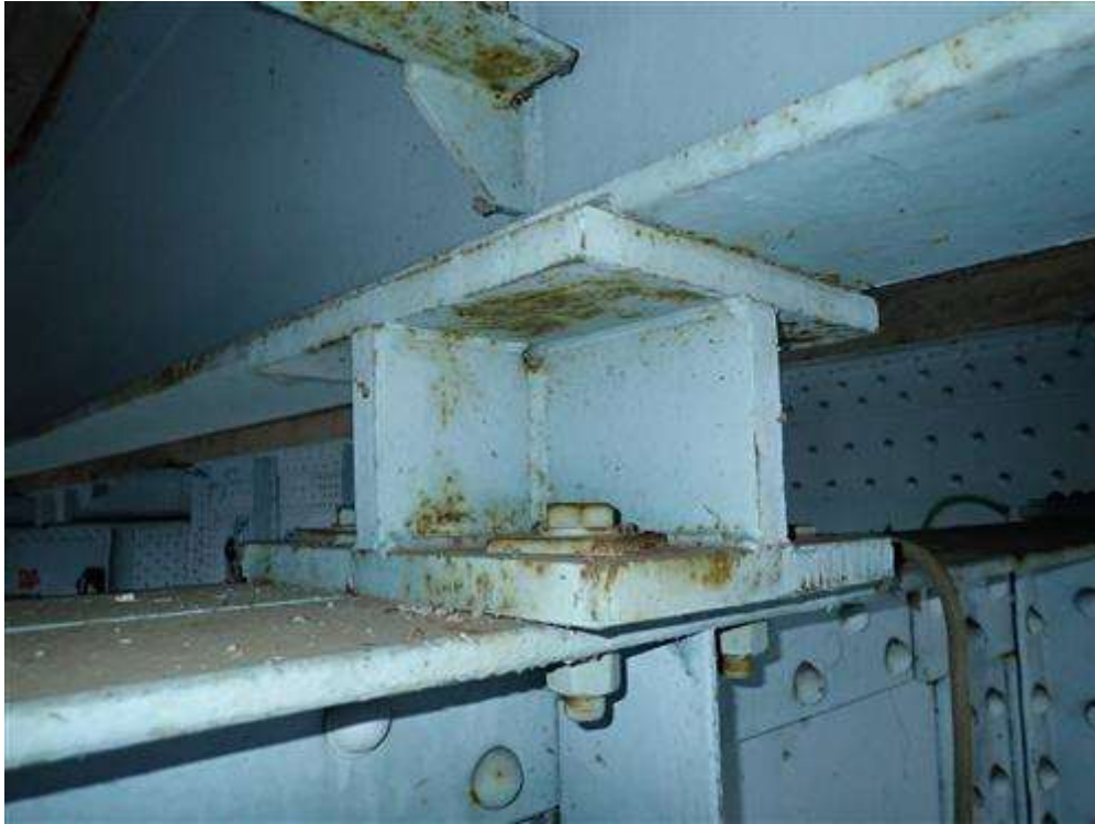
Span 2, Typical Stringer "Bearing" on Floor Beam
