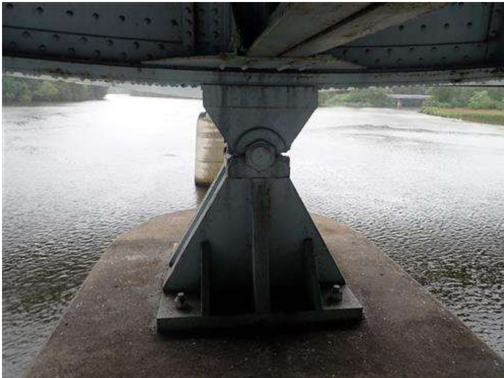
Girder 1 Fixed Bearing at Pier 2
