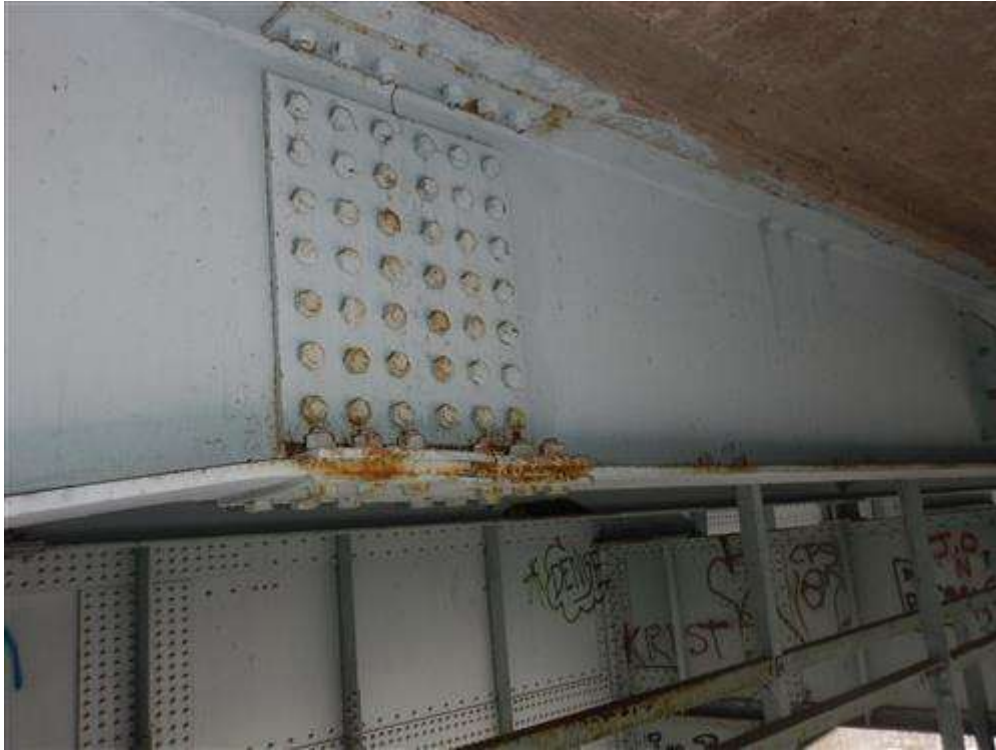
Stringer 5 Field Splice Between Floor Beam 7 and Floor Beam 8
