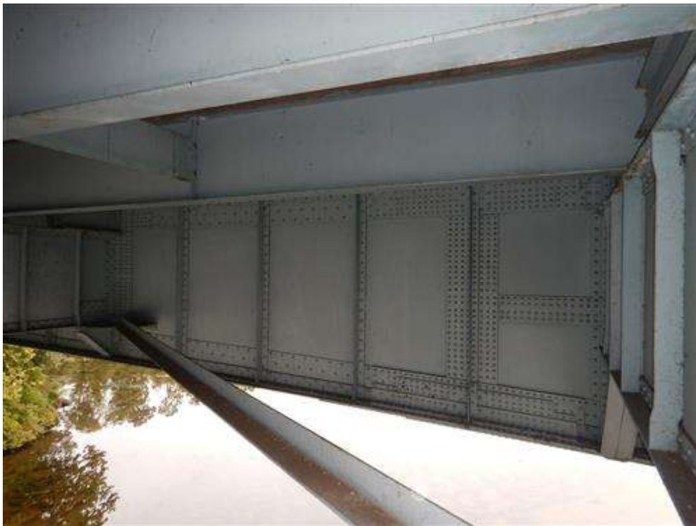
Inside Face of Girder (Typical)
