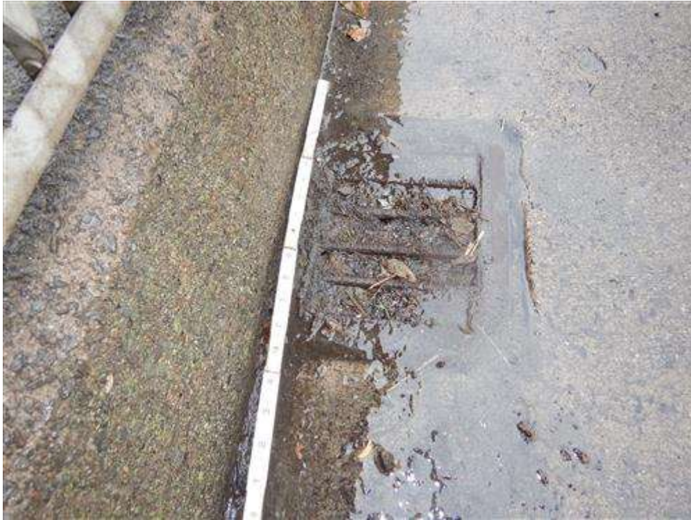
Sidewalk Scupper Grate in Span 4
