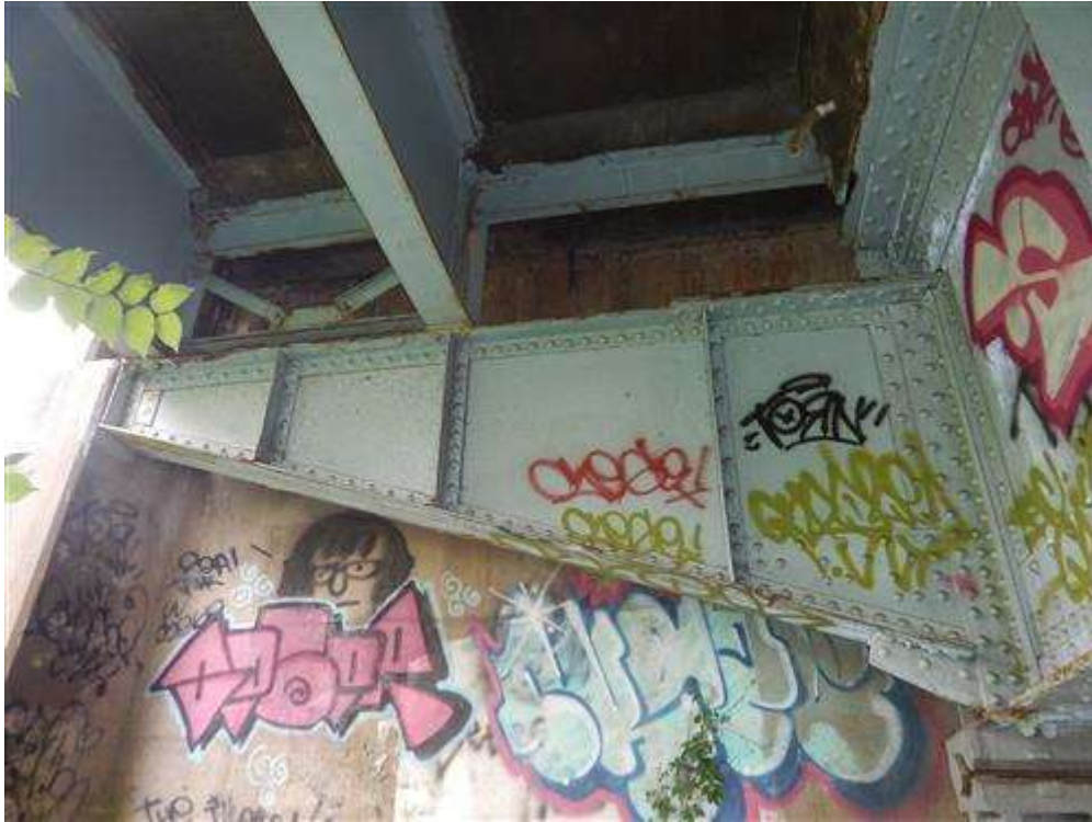
Left Cantilever at Floor Beam 29 (Typical)
