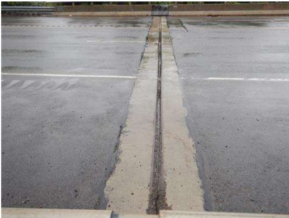
Abutment 1 Compression Joint Seal with Concrete Headers, Looking West
