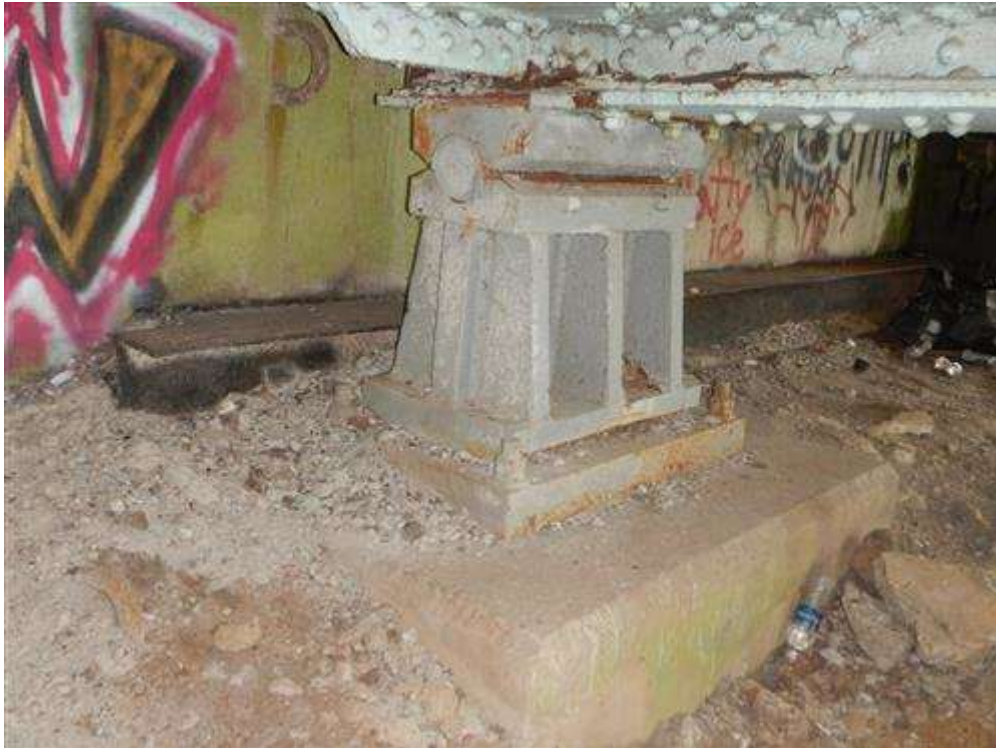
Girder 2 Expansion Bearing at Abutment 2
