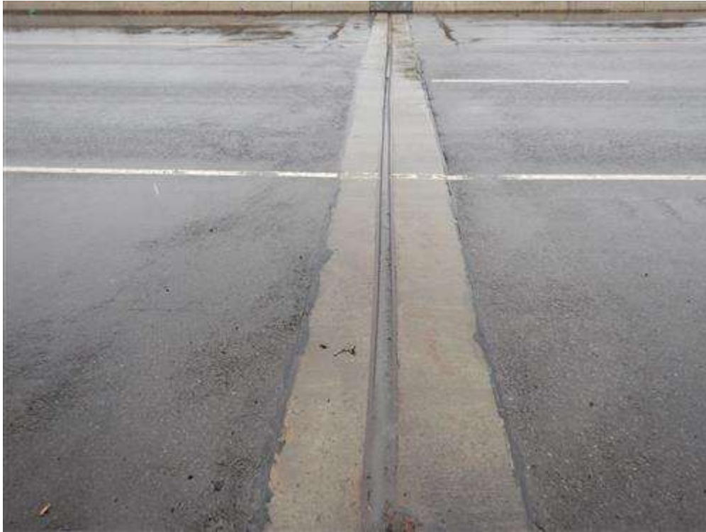
Abutment 2 Compression Joint Seal with Concrete Headers, Looking West
