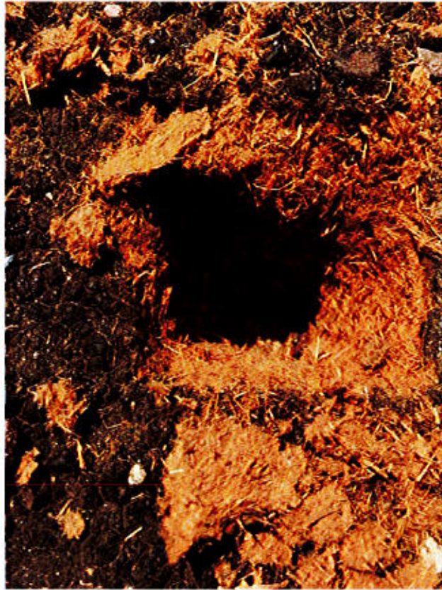
Partical board layers with a tar coating over concrete roof
