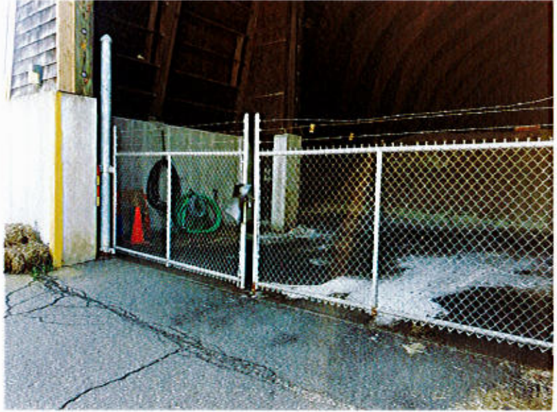
Stafford Salt Shed interior locked
