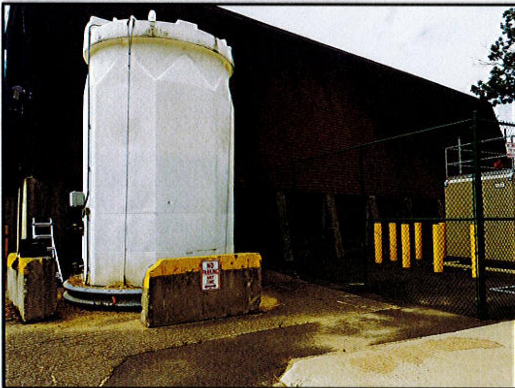
PHOTO 4. Union Salt Shed B-side.
