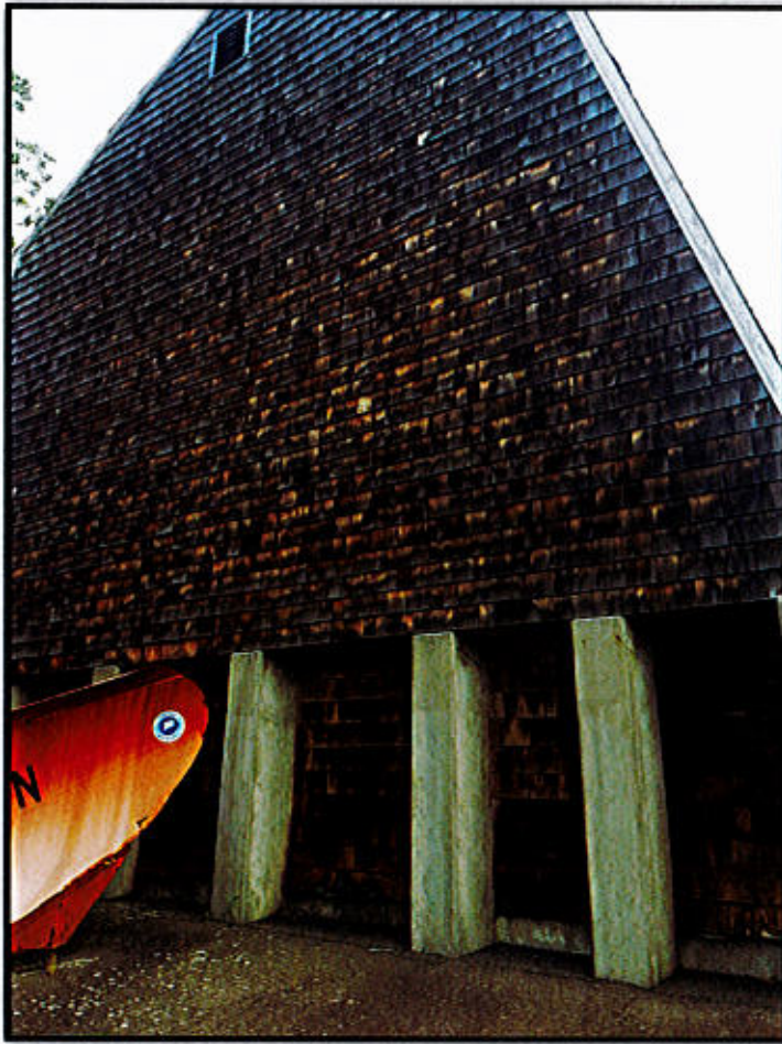
PHOTO 3. Union Salt Shed A-side.
