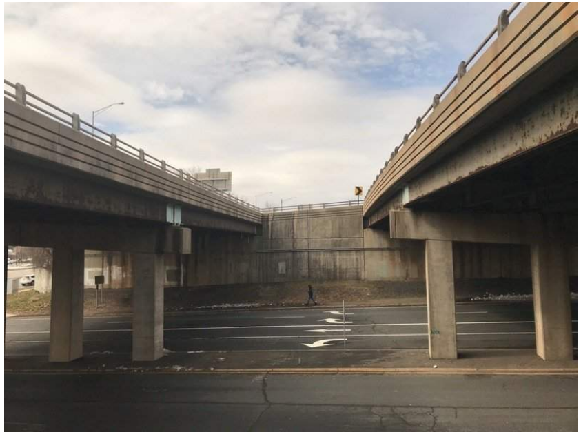
Bridges 01743 A and B
