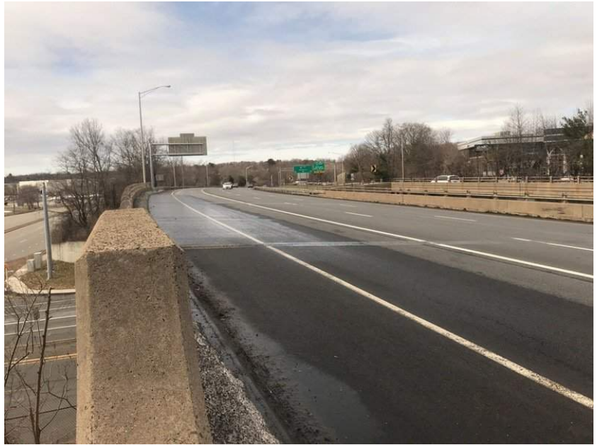
Topside Bridge 01743A
