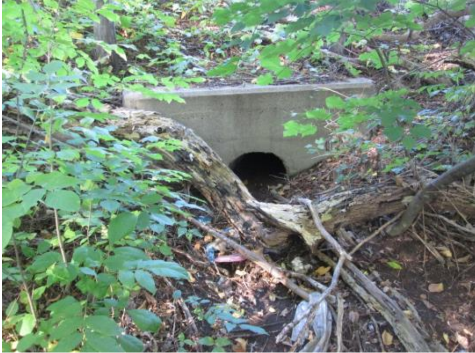
Impact Area 9 (Ramp C 39+25 RT)
