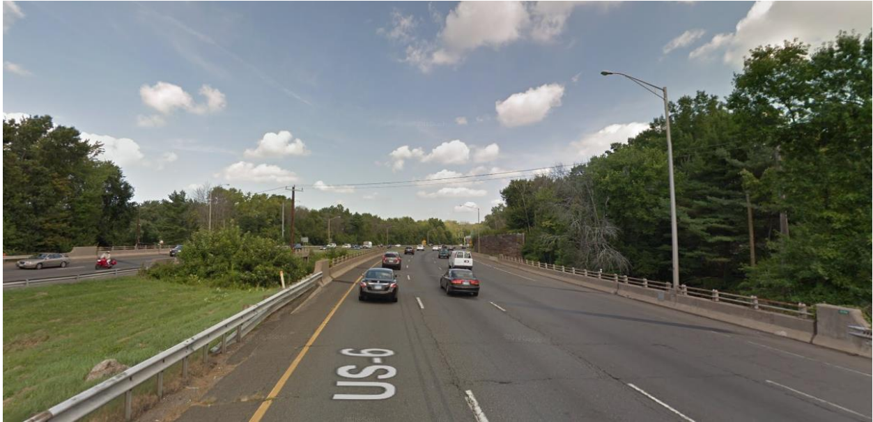
Bridge Nos. 01744 and 01745
