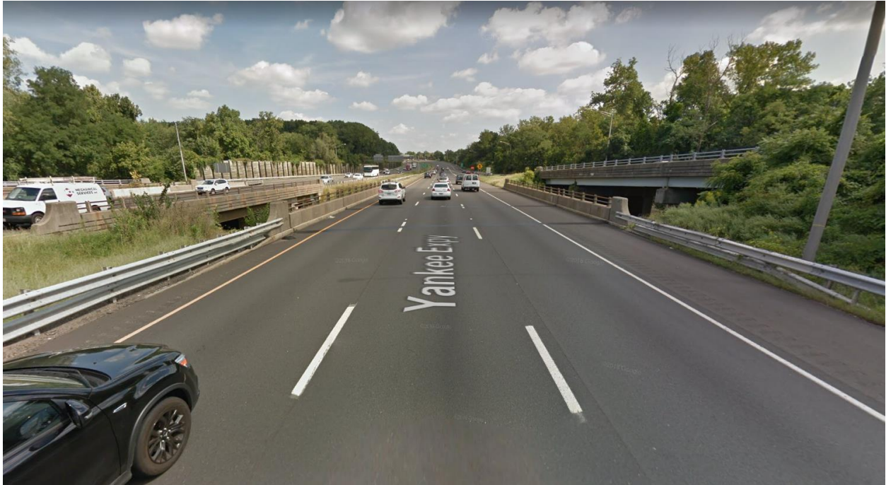
Bridge Nos. 03486, 03489 & 03490 I-84 Eastbound over Woodruff Lane (Exit 39A)
