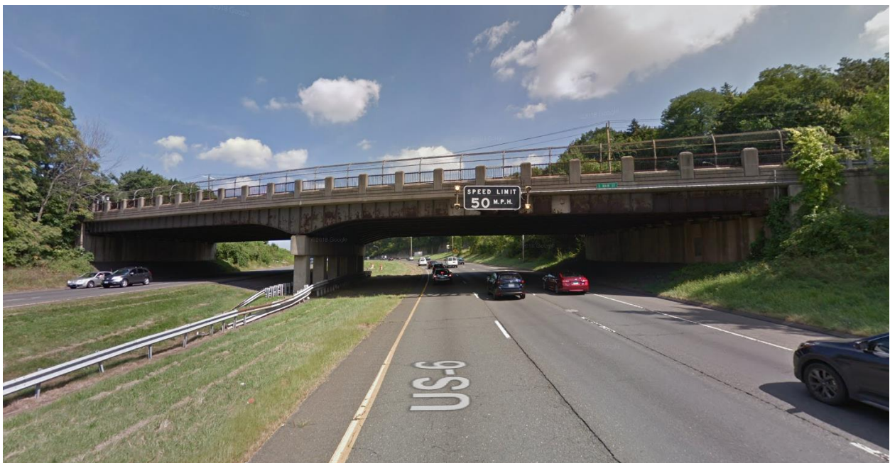
Bridge No. 01747 South Main Street over I-84 Eastbound (Exit 41)
