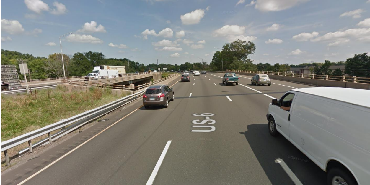
Bridge Nos. 01743A & 01743B I-84 Eastbound over Ridgewood Drive (Exit 40)
