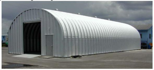
Arches: Twenty-five (25) grade 80 AZM 180/AZ 60 Galvalume Plus coating, double bolt 9" lap seams.
