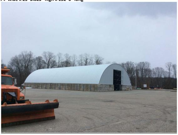
Arches: Seventy-four (74) grade 50 AZM 180/AZ 60 Galvalume Plus coating, double bolt 9" lap seams.
