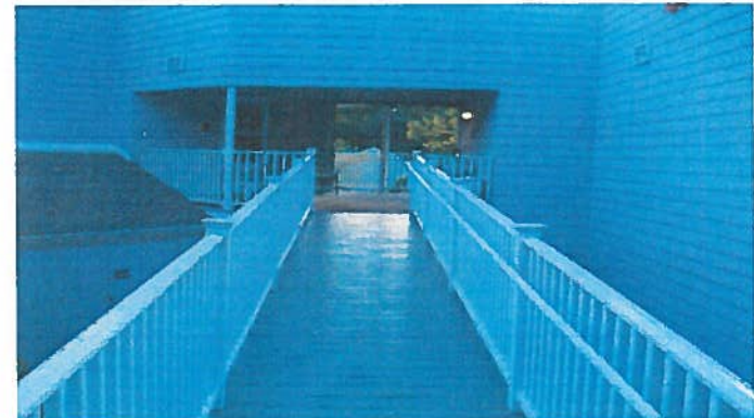
BLDG 215/225 REAR OF BREEZEWAY (FACING RAMP)
