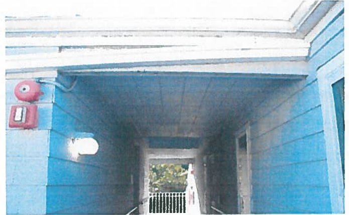
BLDG 165 REAR OF BREEZEWAY (FACING RAMP) 94" HI
