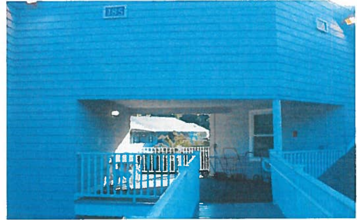
BLDG 185/195 REAR OF BREEZEWAY (FACING RAMP)
