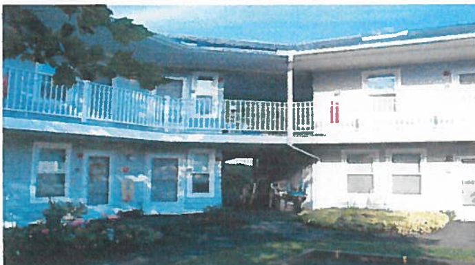
BLDG 215/225 FRONT OF BREEZEWAY (FACING COURTYARD)
