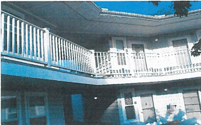
BLDG 185/195 FRONT OF BREEZEWAY (FACING COURTYARD)
