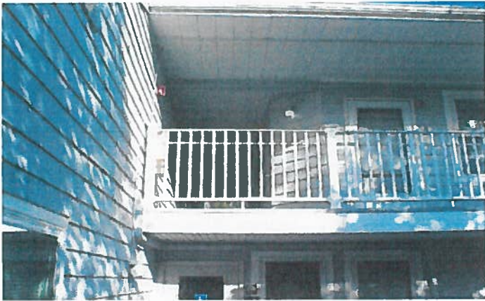
BLDG 165 FRONT OF BREEZEWAY (FACING COURTYARD)
