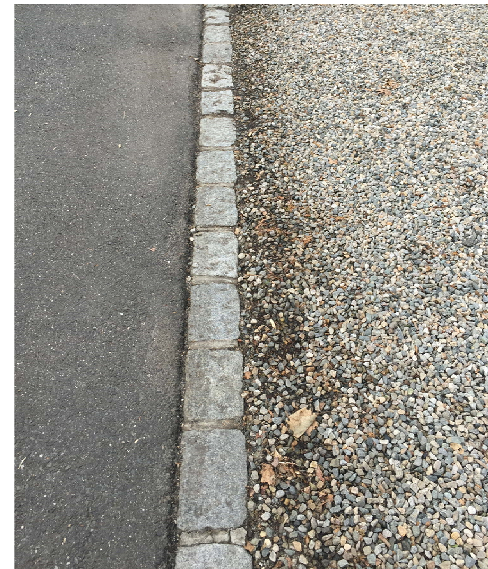
FLUSH BELGIAN BOCK CURB (BETWEEN POROUS ASPHALT AND CRUSHED STONE PARKING) N.T.S.
