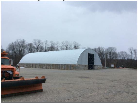
Arches: Seventy-four (74) grade 50 AZM 180/AZ 60 Galvalume Plus coating, double bolt 9" lap seams.
