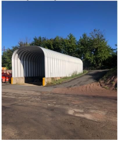
Arches: Twenty-five (25) grade 80 AZM 180/AZ 60 Galvalume Plus coating, double bolt 9" lap seams.
