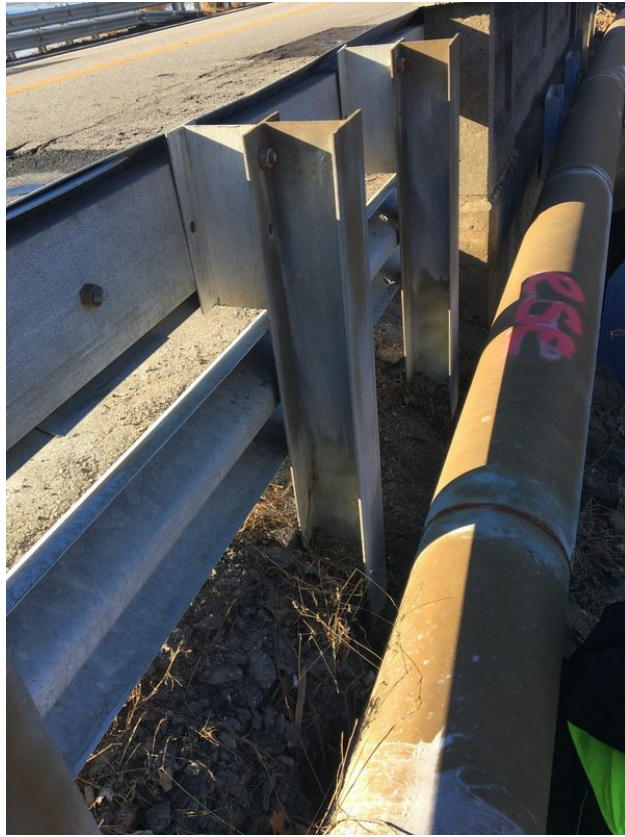
North side of bridge
