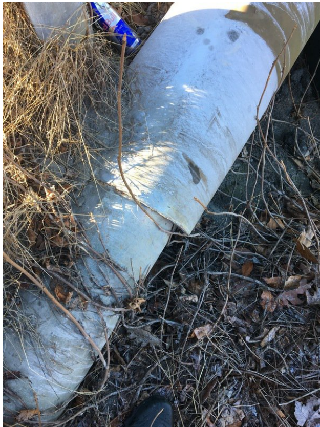
North side of bridge
