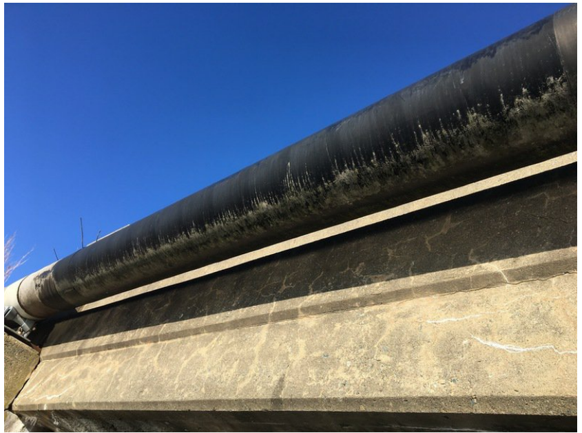
South side of bridge
