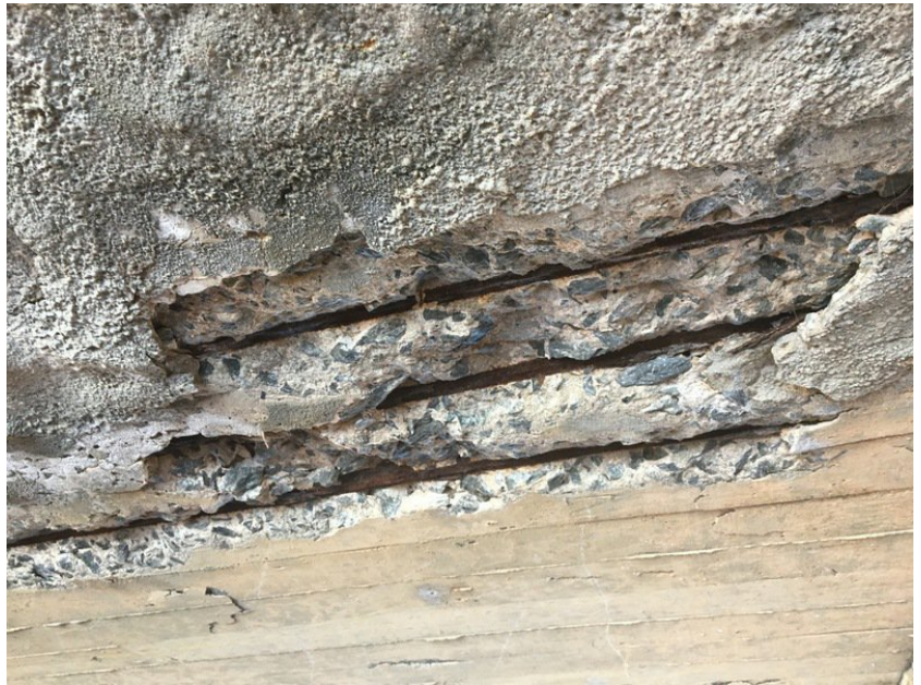
Under side of bridge
