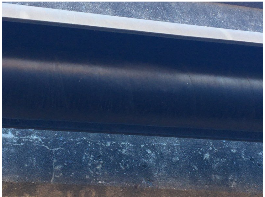
Pipe on North side of bridge
