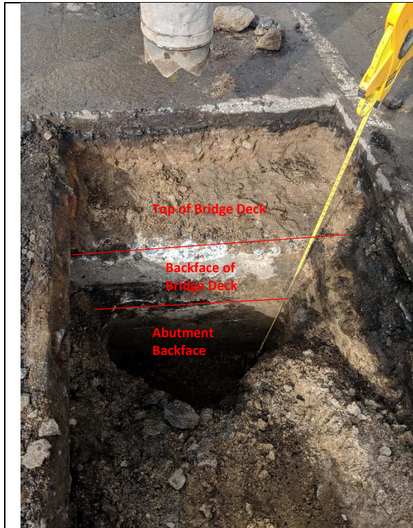
Bridge 02931, Test Pit T-2-2, facing west, looking down. Depth of test pit.
