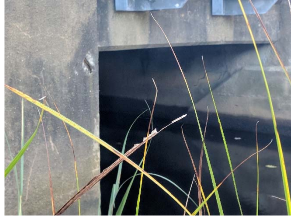
Bridge 02932, facing west, beneath bridge Abutment face
