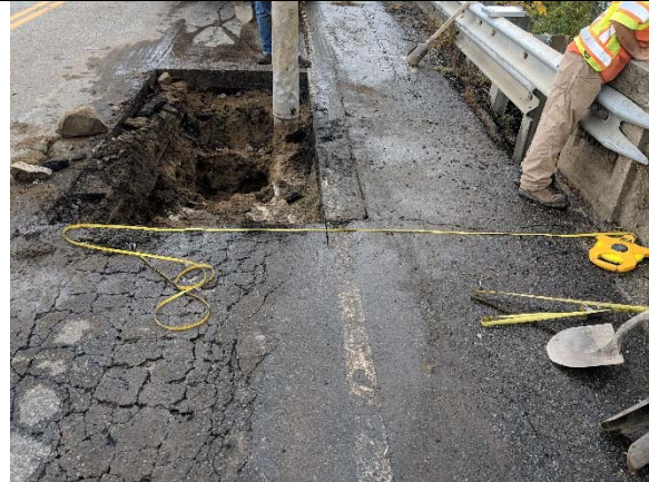
Bridge 02931, Test Pit T-2-1, facing west, looking down. Test pit during vacuum excavation.
