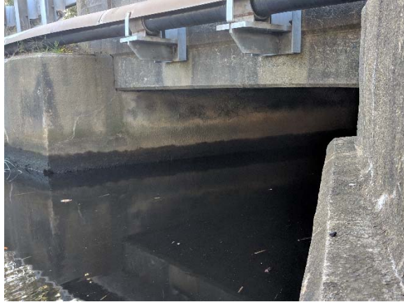
Bridge 02932, facing east, beneath bridge Abutment face
