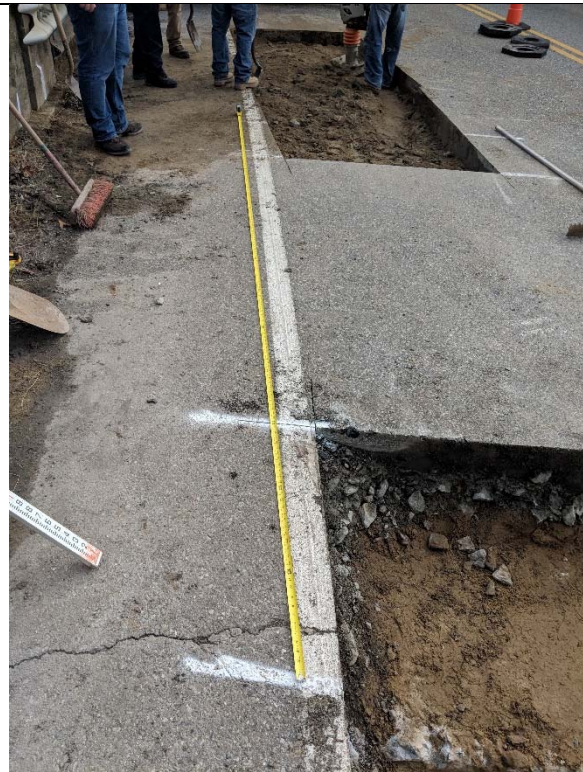
Bridge 02932, facing east Length of bridge deck
