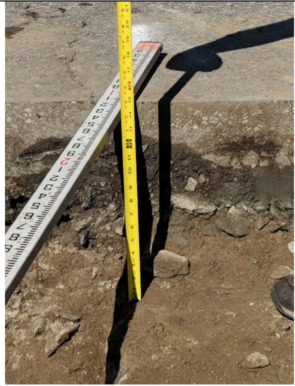
Bridge 02931, T-2-3, facing north Thickness of existing asphalt and soil above bridge deck
