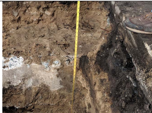
Bridge 02931, Test Pit T-2-2, facing west. Looking across test pit.
