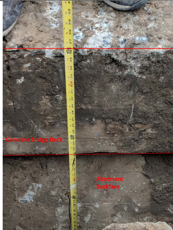
Bridge 02931, Test Pit T-2-4, facing west. Depth from bottom of test pit to the top of the concrete deck.
