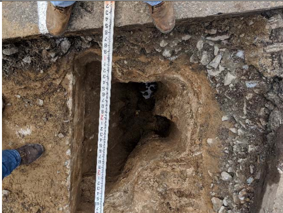
Bridge 02932, T-1-1, facing down Water at bottom of Test Pit
