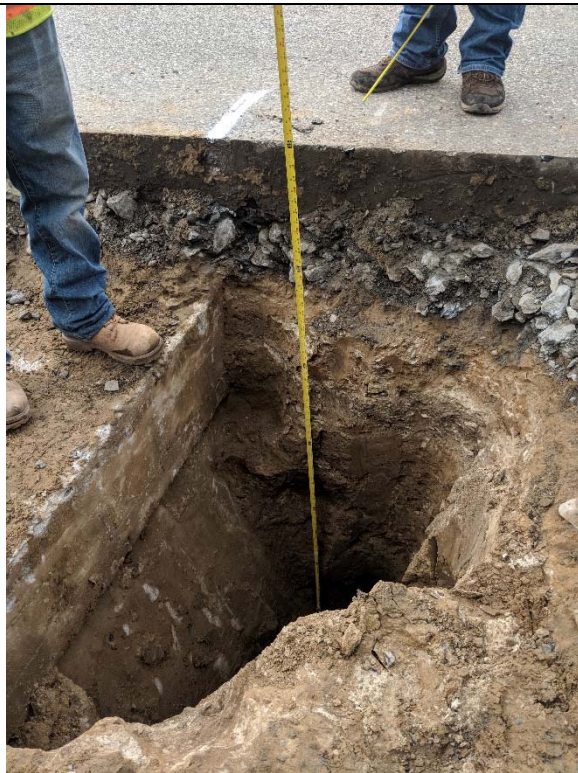
Bridge 02932, T-1-1, facing south General view of depth of test pit
