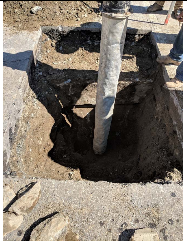
Bridge 02931, T-2-3, facing east Vacuum excavating the test pit
