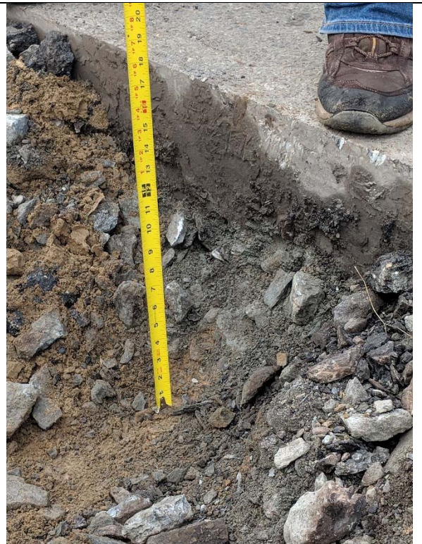
Bridge 02932, T-1-2, facing southeast Thickness of existing asphalt and soil above bridge deck
