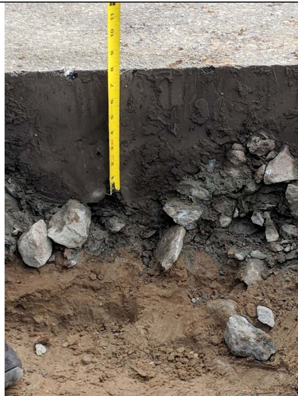
Bridge 02932, T-1-1, facing east Thickness of existing asphalt above bridge deck
