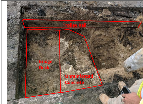
Bridge 02931, Test Pit T-2-1, facing south, looking down. Top of exposed bridge deck, unreinforced concrete behind bridge deck, trolley rail exposed.
