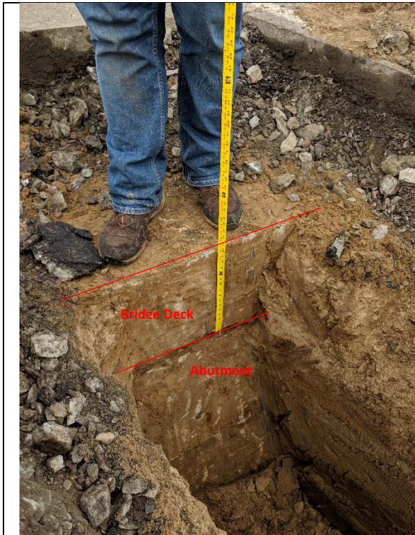
Bridge 02932, T-1-2, facing northwest Thickness of bridge deck
