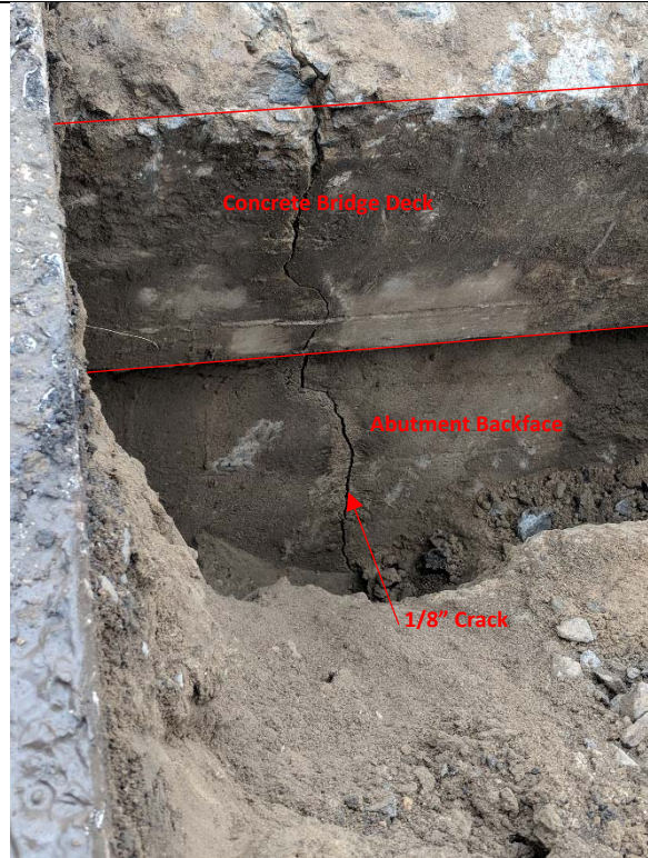
Bridge 02931, Test Pit T-2-4, facing west, looking down. Crack running from bridge deck and through abutment.
