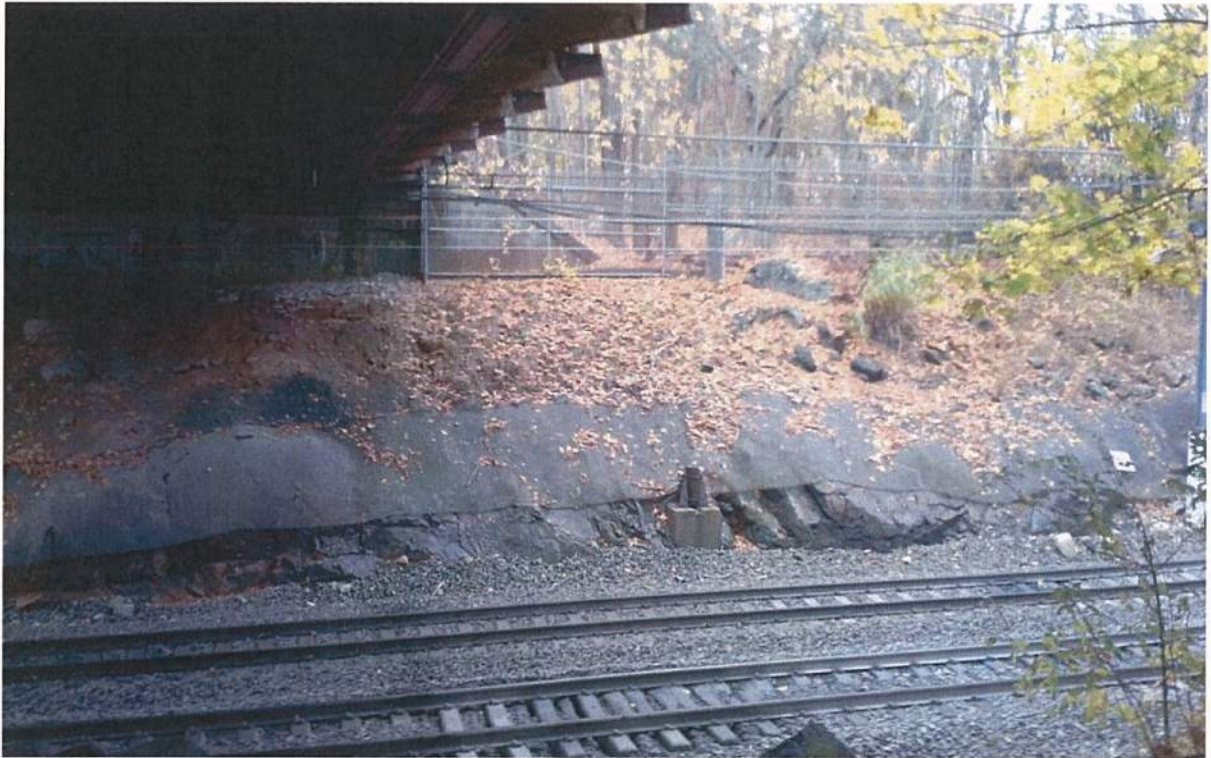
Amtrak railroad under Bridge No. 03903 looking at west abutment
