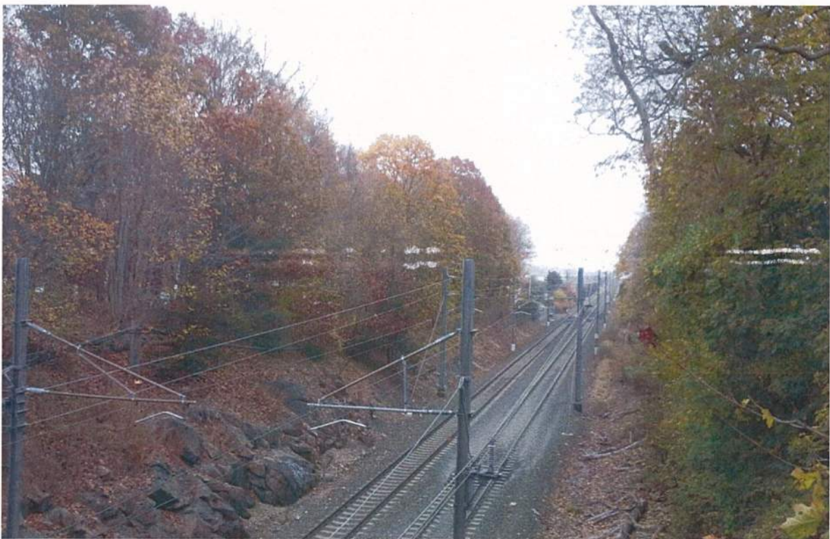
Looking northeast along Amtrak rail from Bridge No. 03903
