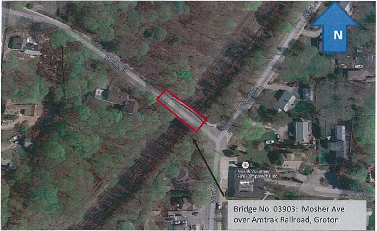
Aerial photo of Bridge 03903 (Google)
