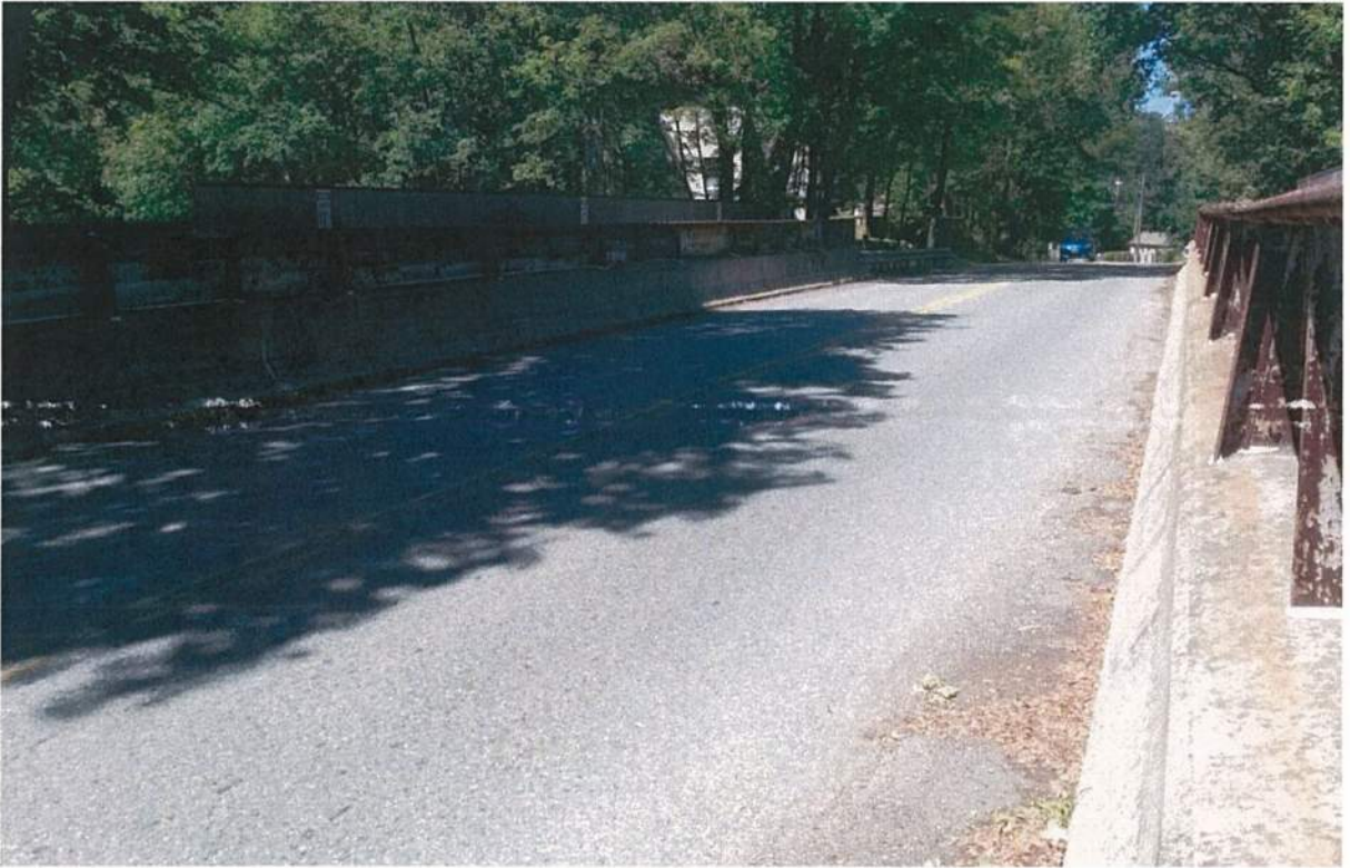
Bridge No. 03903 looking approximately northwest
