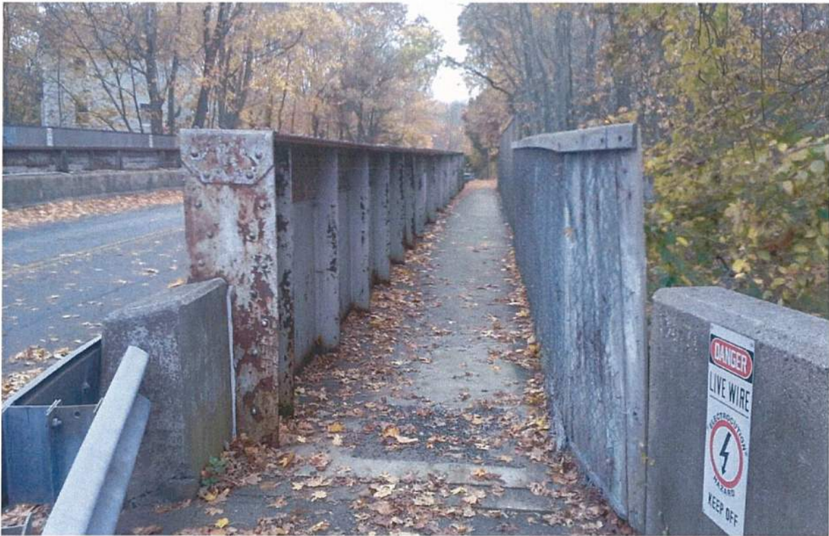
Sidewalk at north side of Bridge No. 03903
