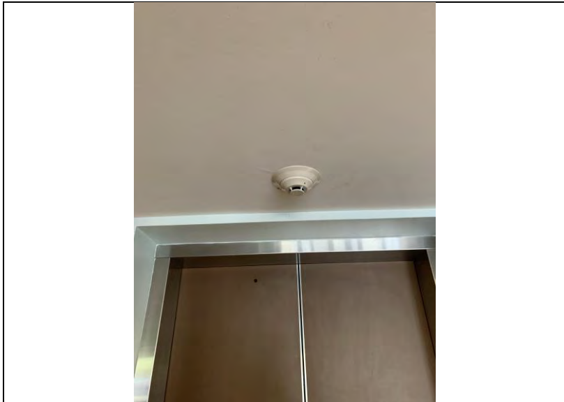
Vestibule Fire Detection Smoke Head
