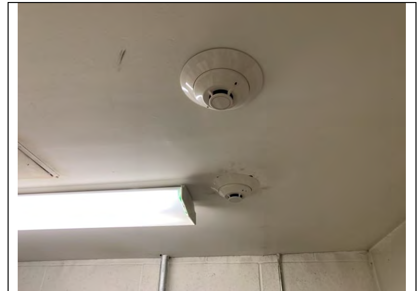
Machine Room Fire Detection Smoke Heads
