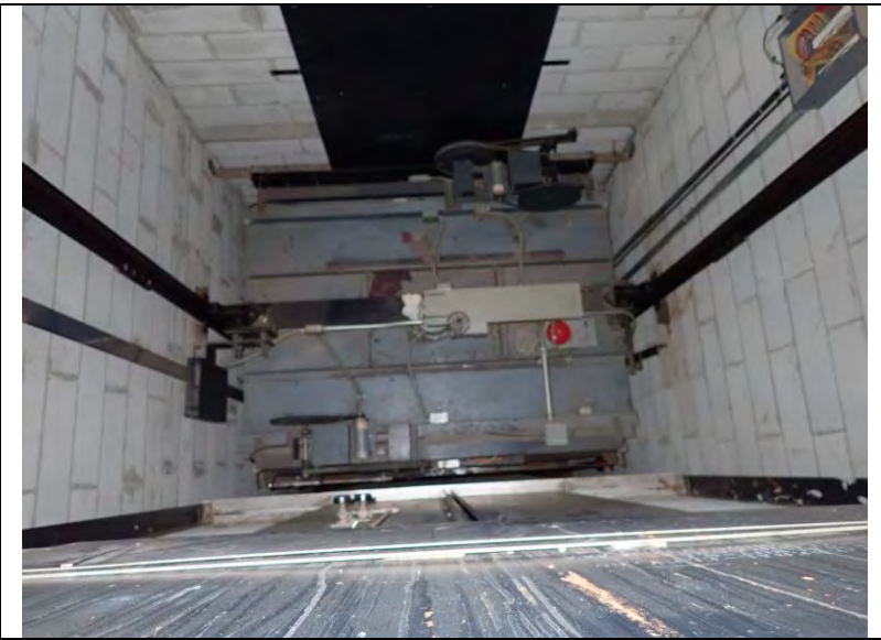
17 Elevator Hoistway and Top of Cab
