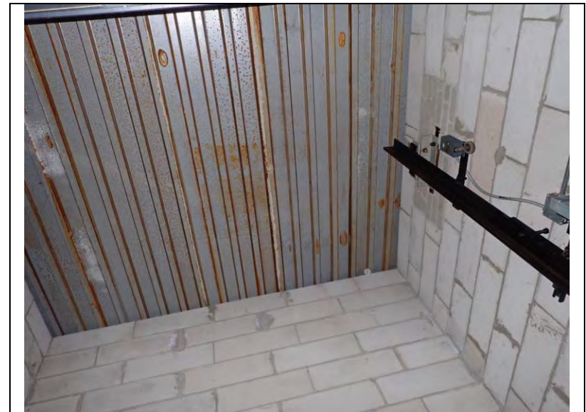
20 Top of Elevator Hoistway
