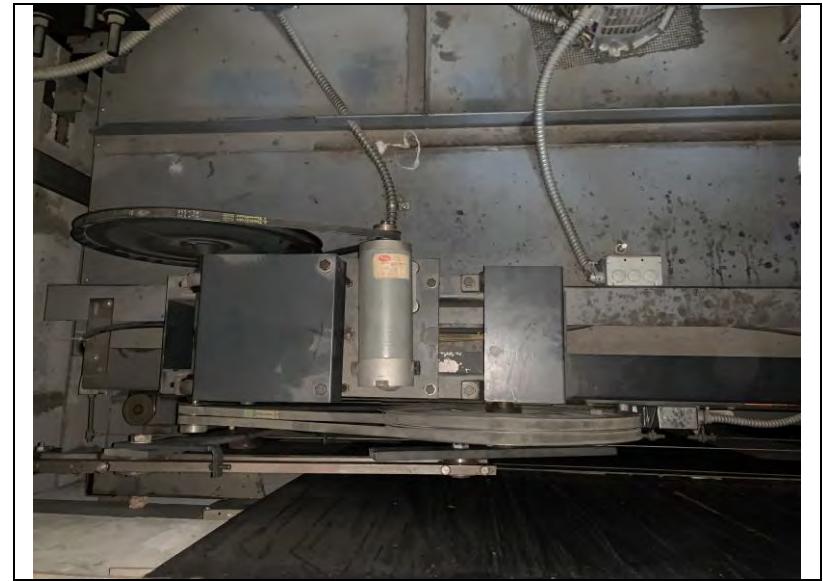
18 Original Moline Door Operator
