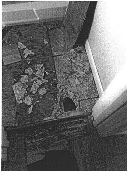
Multiple layers of flooring in bathroom
