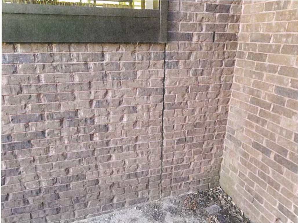
1977 Addition Dark Gray Expansion Caulk
