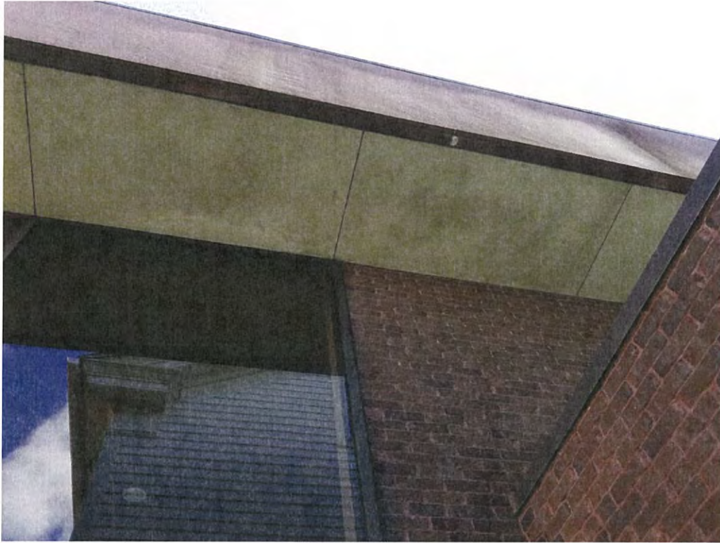
1977 Addition Concrete Panels
