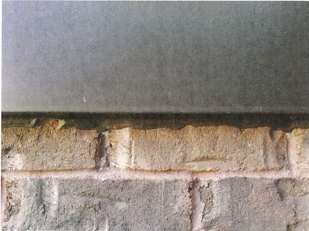
1977 Addition Window Caulk Tar
