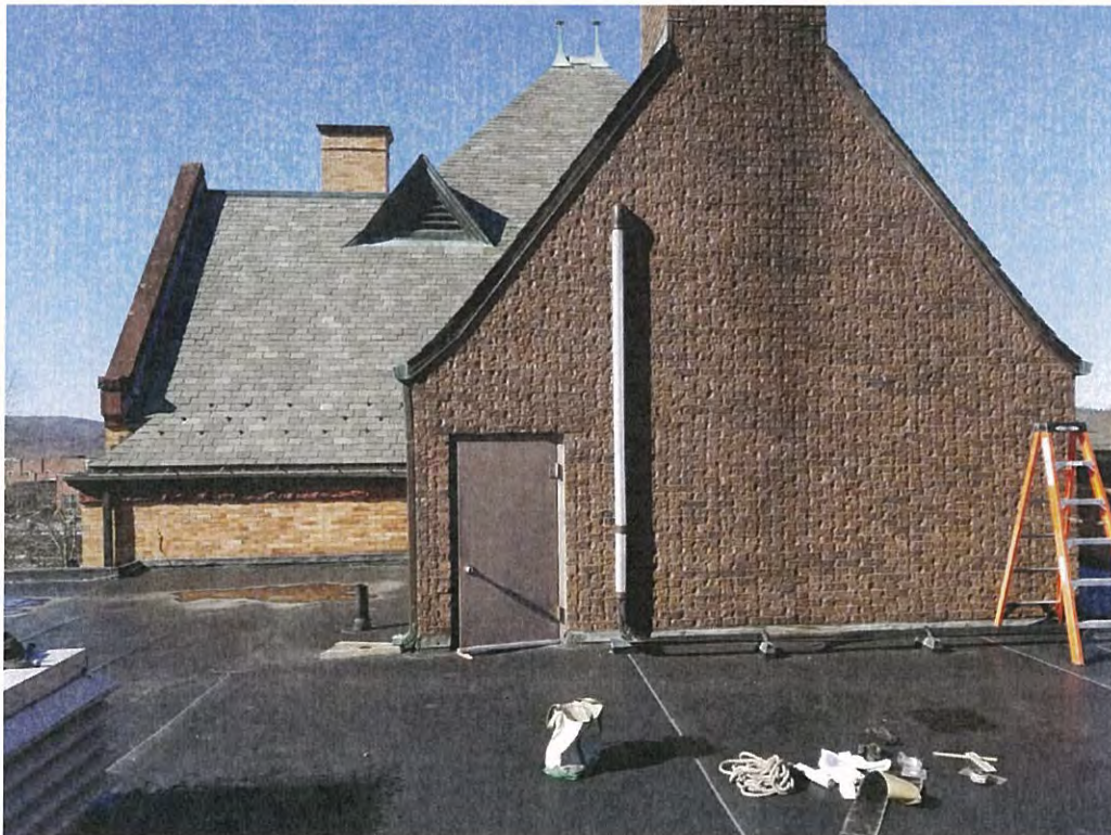
1977 Addition Roof Overall
