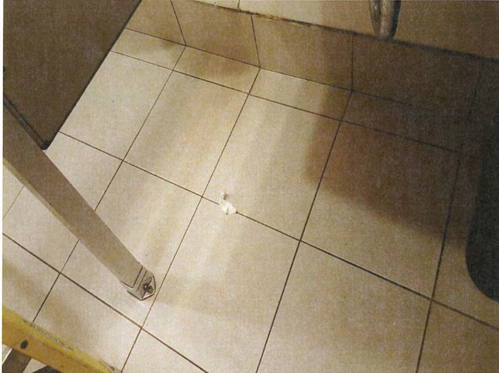
1977 Addition Men's Bathroom Floor
