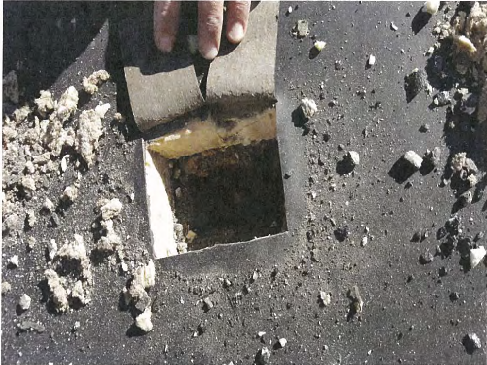
1977 Addition Roof Field
