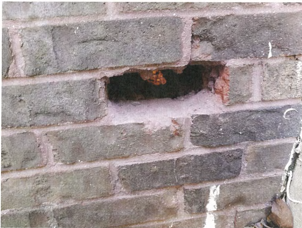
1977 Addition Dampproofing behind Brick
