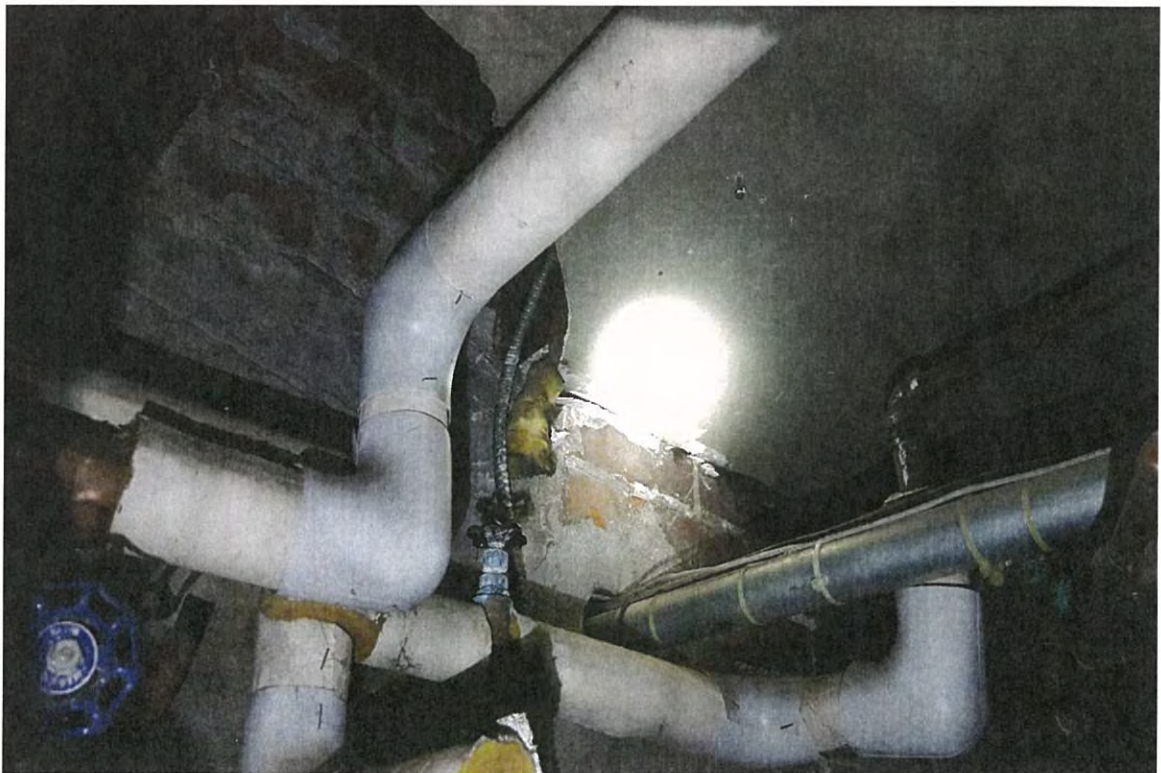
1897 Section Basement Storage 003 Transite Ceiling
