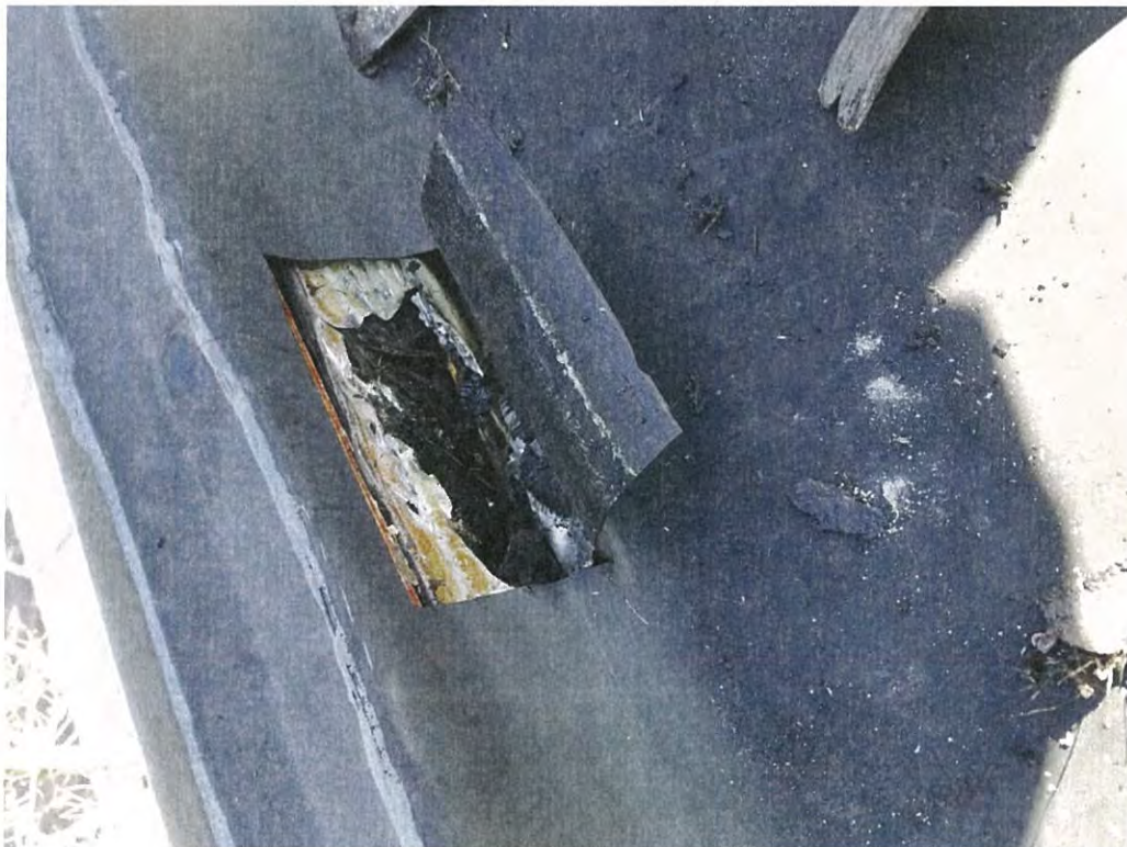
1977 Addition Roof Perimeter
