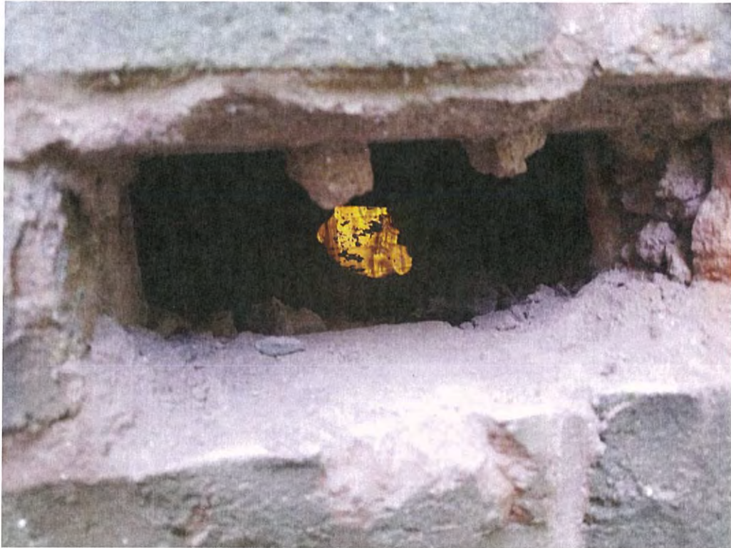
1977 Addition Dampproofing behind Brick
