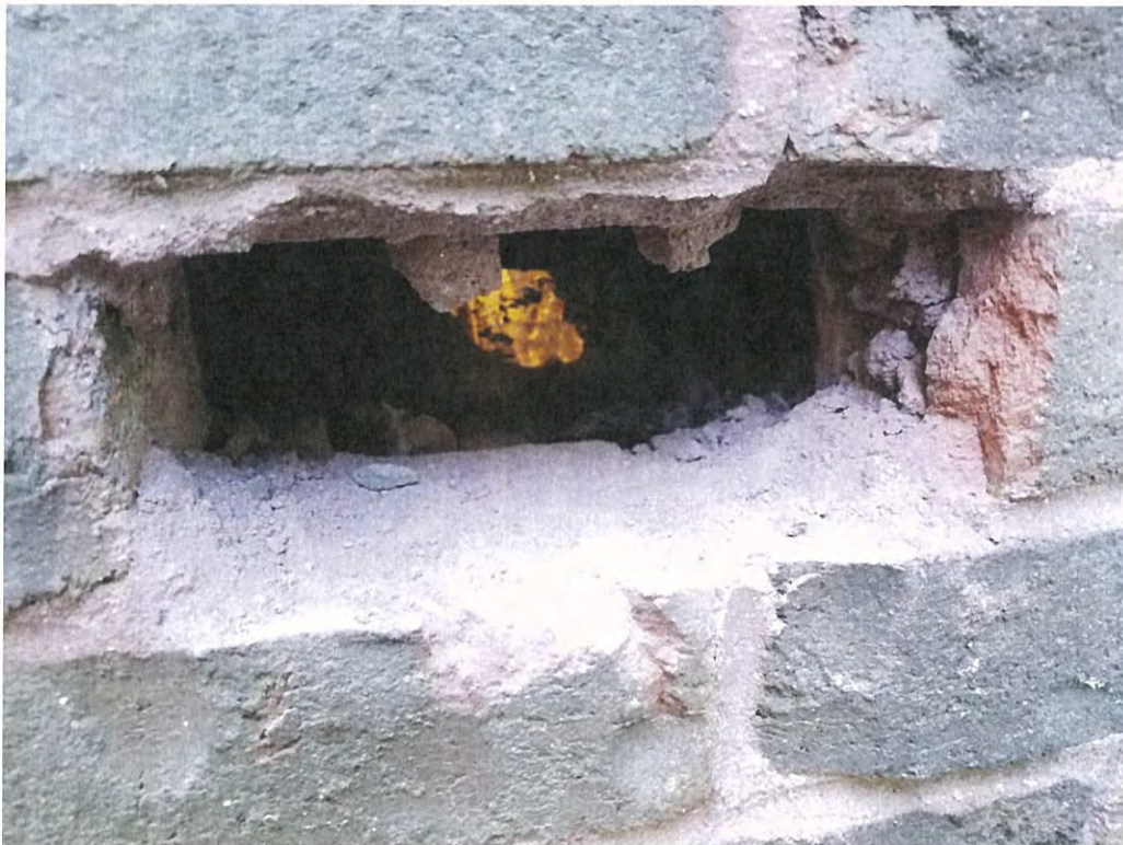
1977 Addition Dampproofing behind Brick
