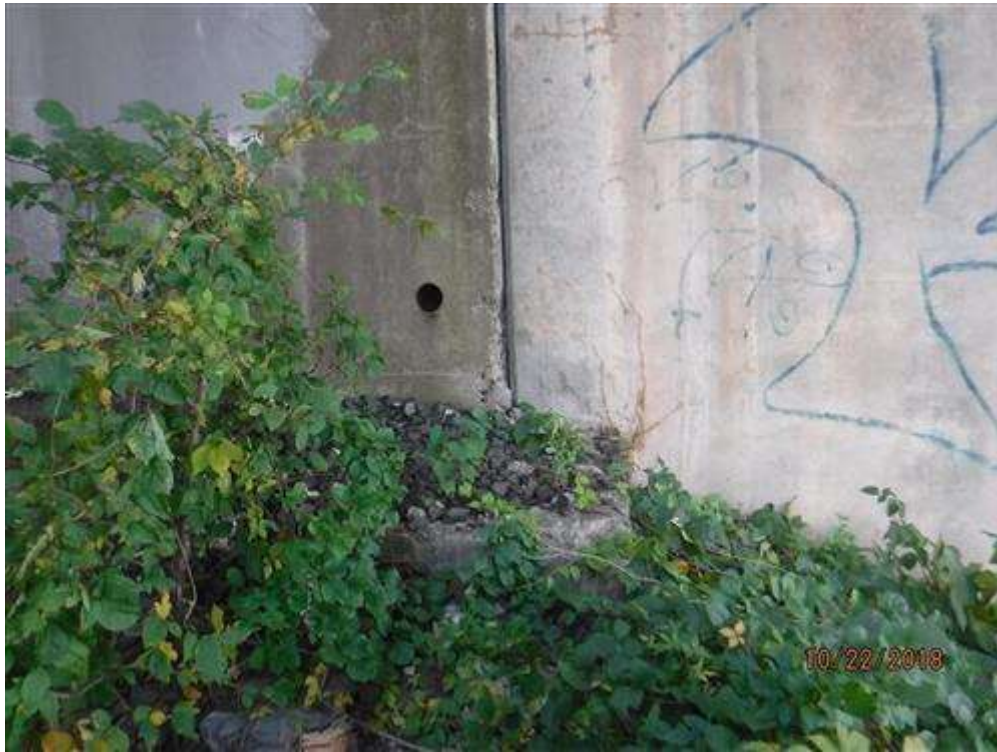
Exposed footing at west end of abutment 1 with a corner spall.
