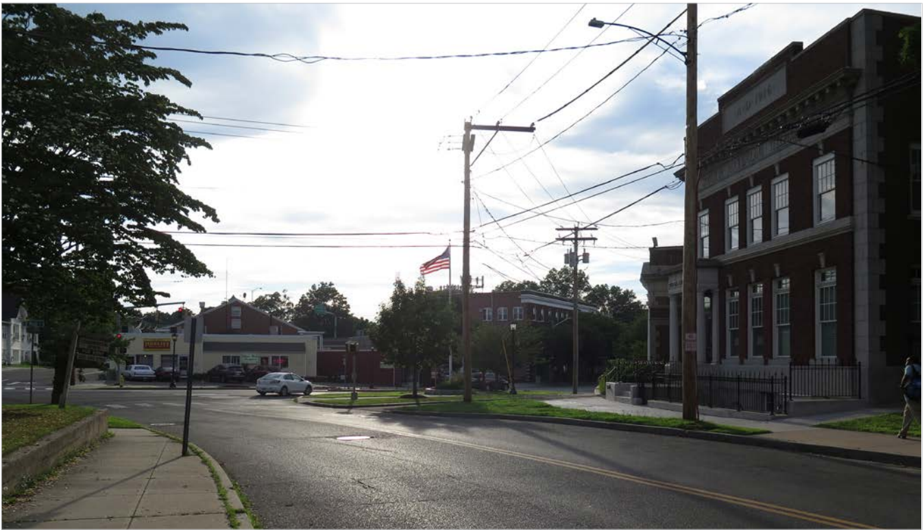
Main St. in Stratford Center is home to a mix of residential units, retail establishments, civic institutions, and professional uses. The view of Main St. from East Broadway is shown above. On the right is The Center Lofts on Main, which is a historical brick building that was recently converted into 5 upscale loft apartments
