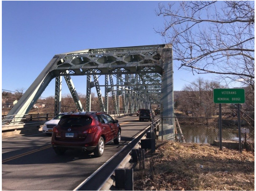
View from west side of bridge
