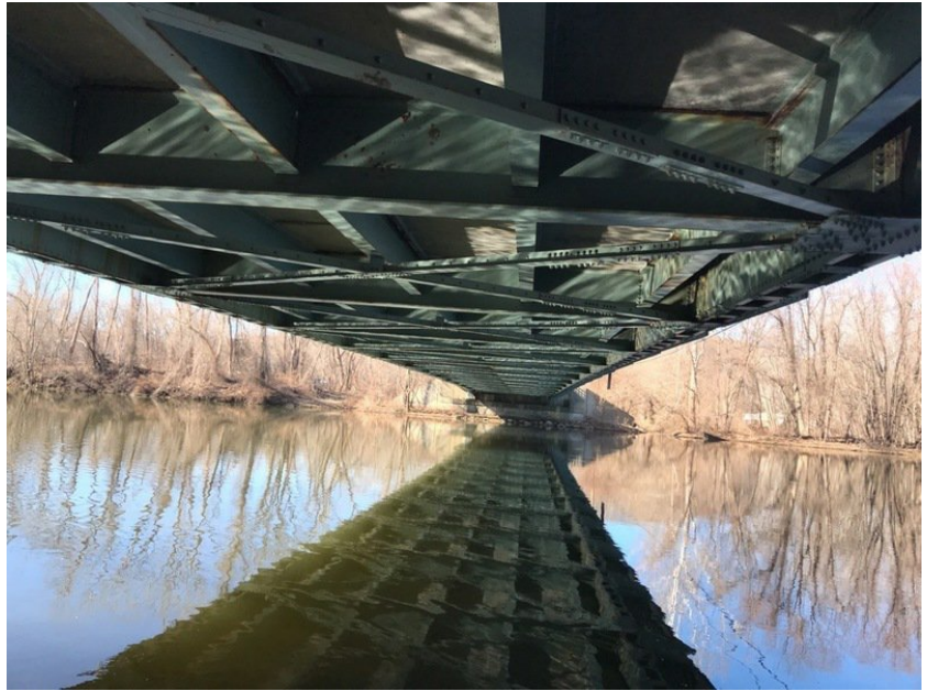
Underside of bridge from east
