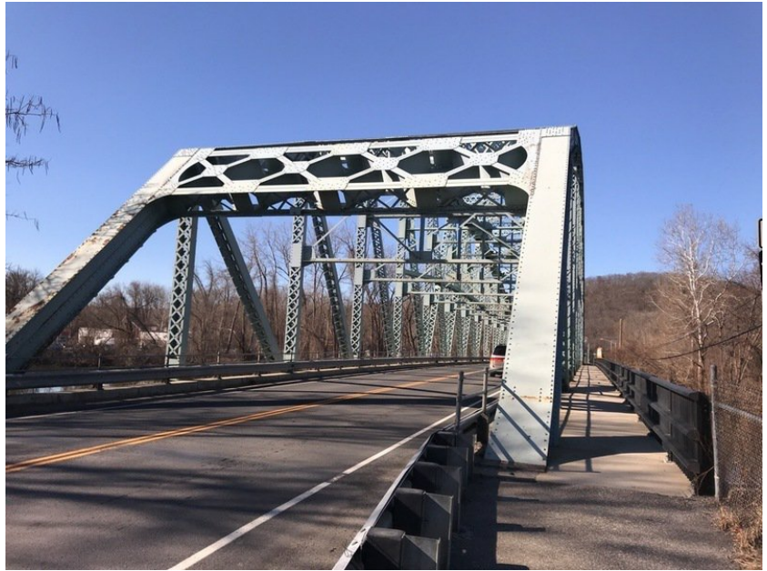
View from east side
