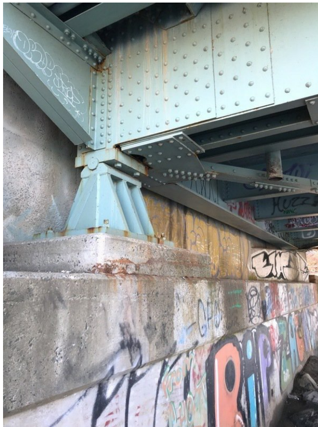
East underside support pad
