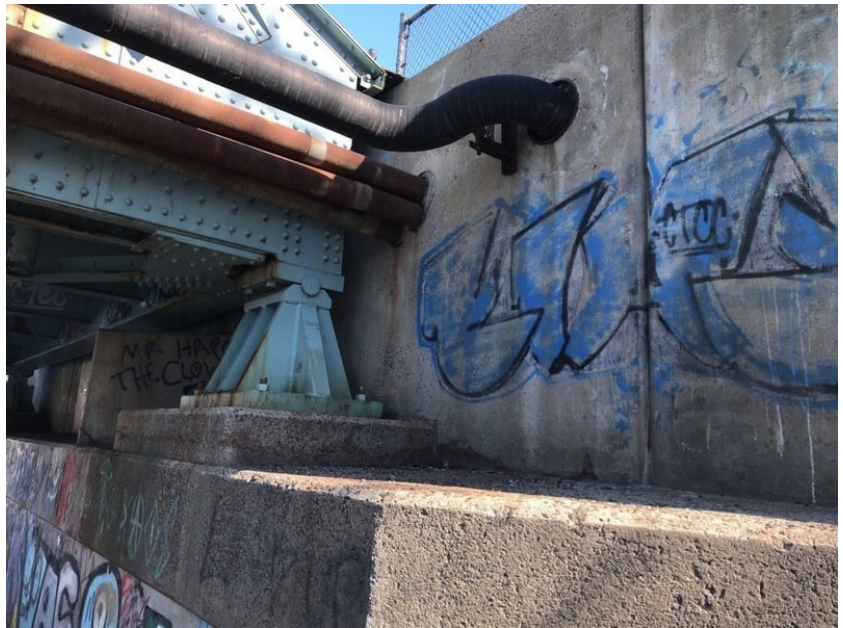
Southeast underside of bridge
