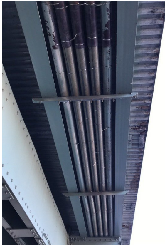
Additional piping on north side
