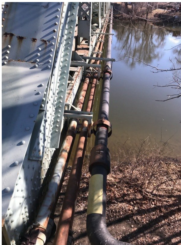
Pipeline running alongside bridge on south side
