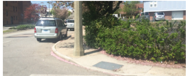
A pole blocks ADA and pedestrian access at the intersection of Governor Winthrop Blvd. at Meridian St.
