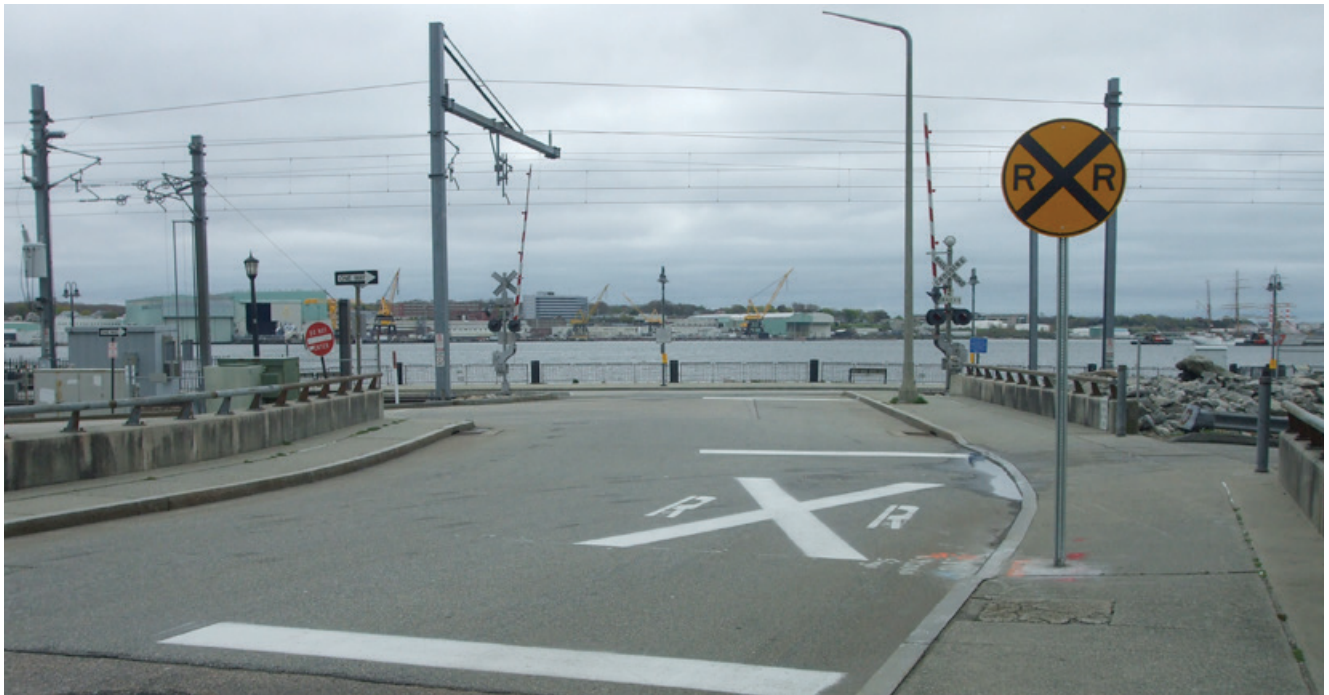
At-Grade Railroad Street Crossing at Bank St. Connector east of South Water St.
