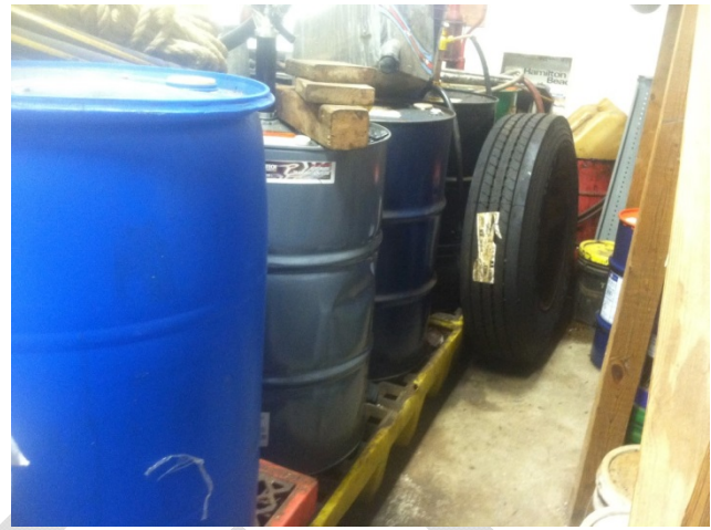
Photo Description: 55-gallon drums in secondary containment in Oil Storage Room
