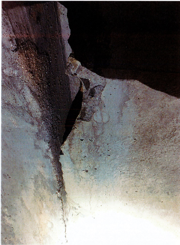
6' concrete pipe interior seam
