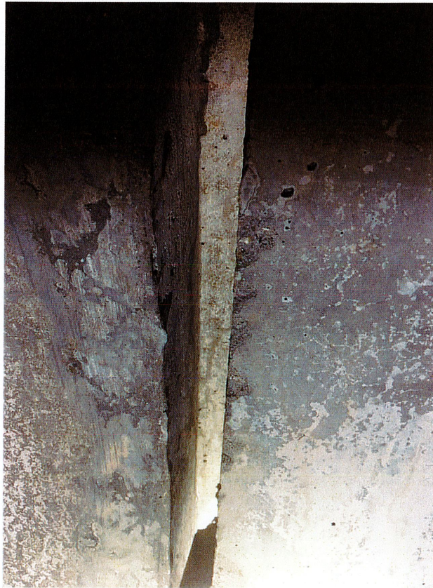
Interior of 6' concrete pipe seam
