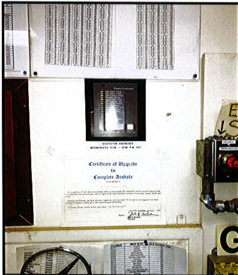
Photo 36. East Windsor Maintenance Facility – Prospect Hill Road, East Windsor, CT. Tank Monitoring System.
