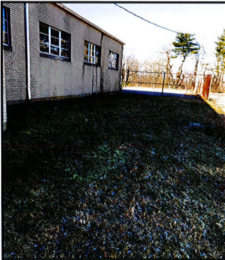
Photo 17. East Lyme Property & Facilities Region 2 Facility – Rt. 156, East Lyme, CT. Proposed Generator Location.
