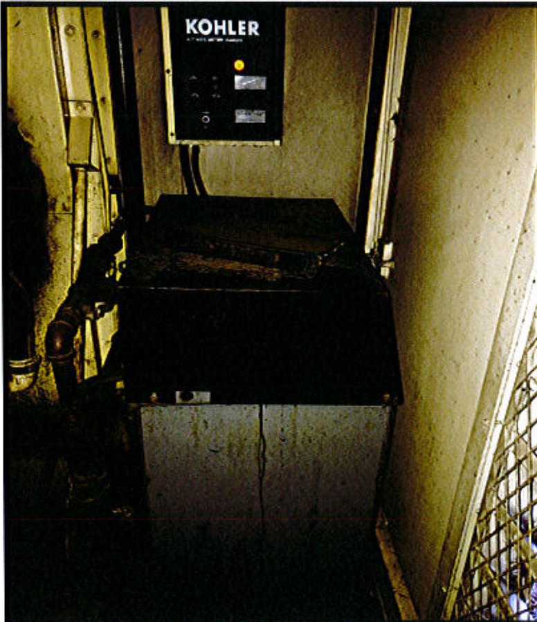
Photo 76. Mansfield Maintenance Facility – 100 N. Frontage Road, Mansfield, CT. Inside Geo.
