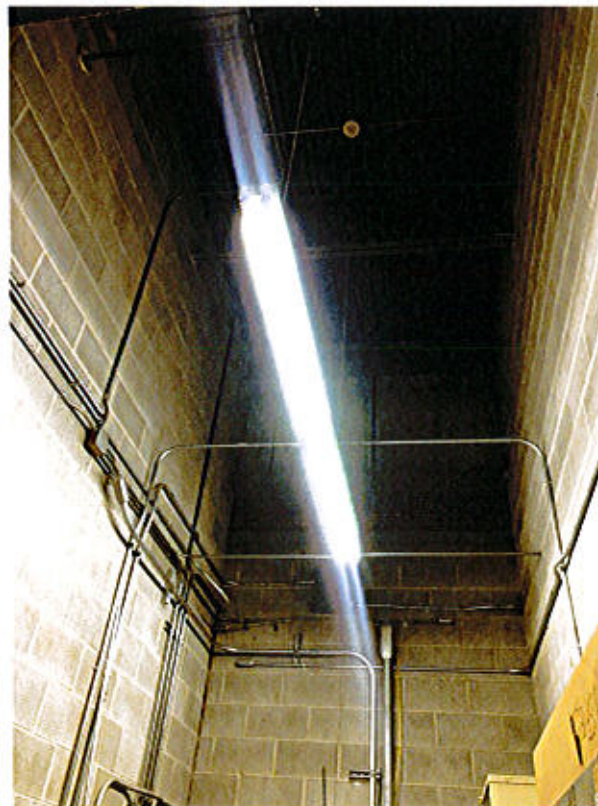
Generator room ceiling
