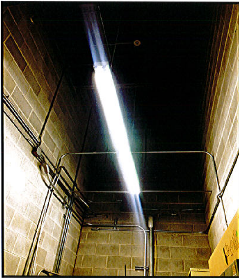
Photo 67. Mansfield Maintenance Facility – 100 N. Frontage Road, Mansfield, CT. Generator Room Ceiling.
