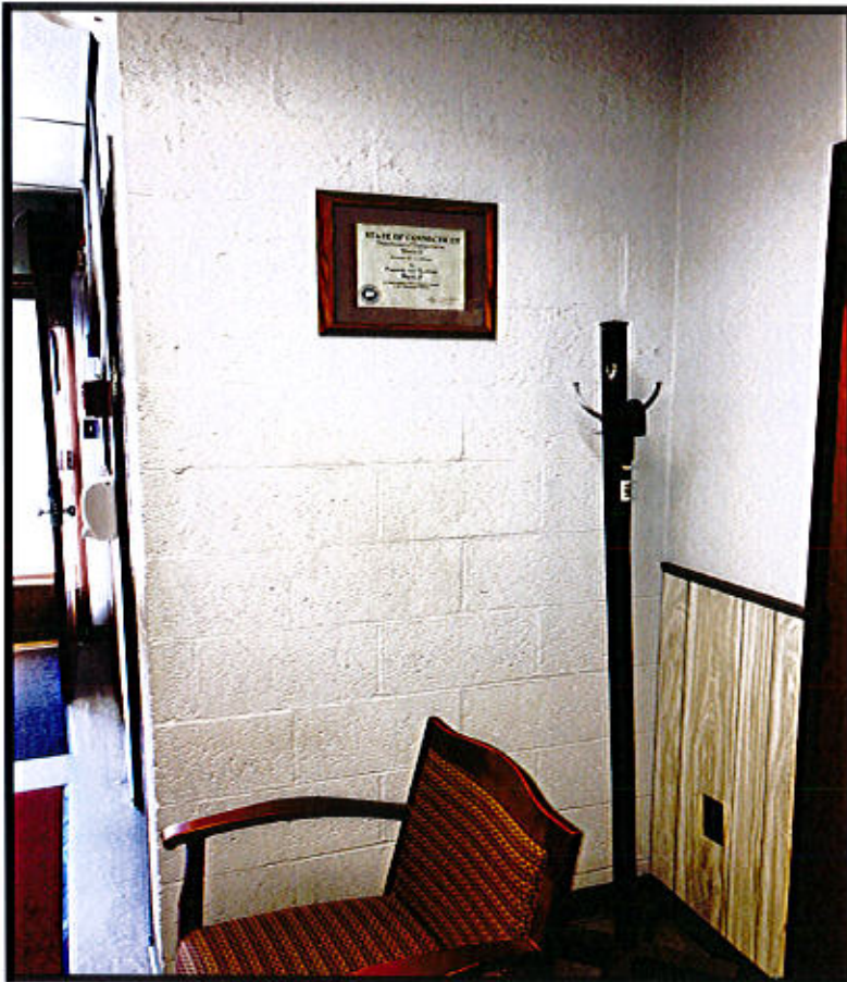
Photo 19. East Lyme Property & Facilities Region 2 Facility – Rt. 156, East Lyme, CT. Possible Annunciator Location.
