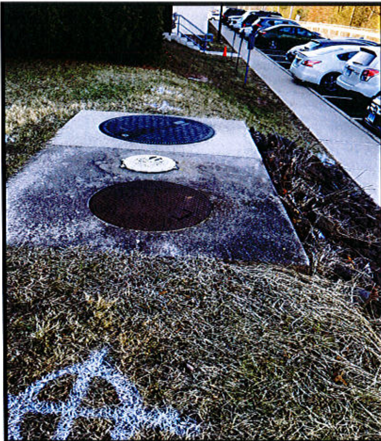
Photo 72. Mansfield Maintenance Facility – 100 N. Frontage Road, Mansfield, CT. UST Covers.
