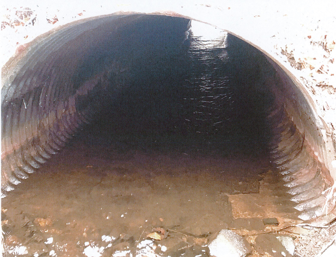
Photo 2 Bridge No. 06676 Inside of Culvert
