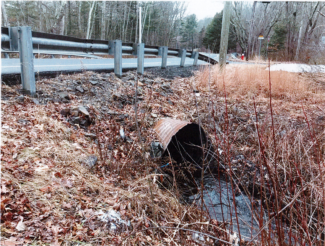
Photo 3 Bridge No. 06676 Outlet of Culvert
