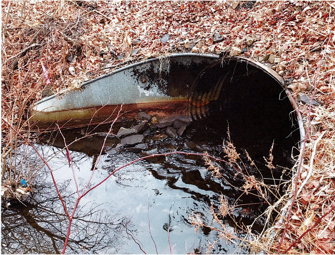
Photo 1 Bridge No. 06676 Culvert Inlet
