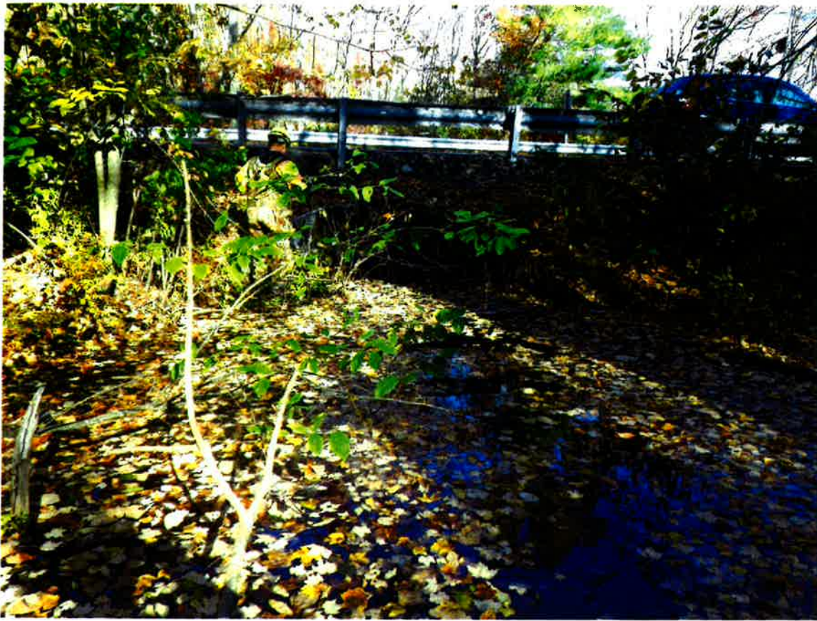
3. Upstream Elevation of Bridge No. 06676
