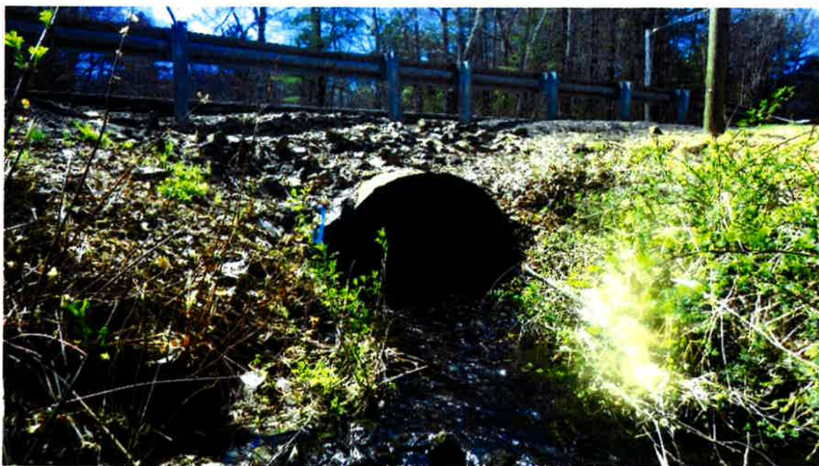
Image 1: Outlet of Structure #06676.
