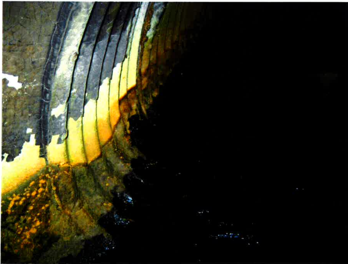
8. Typical Condition of Pipe
