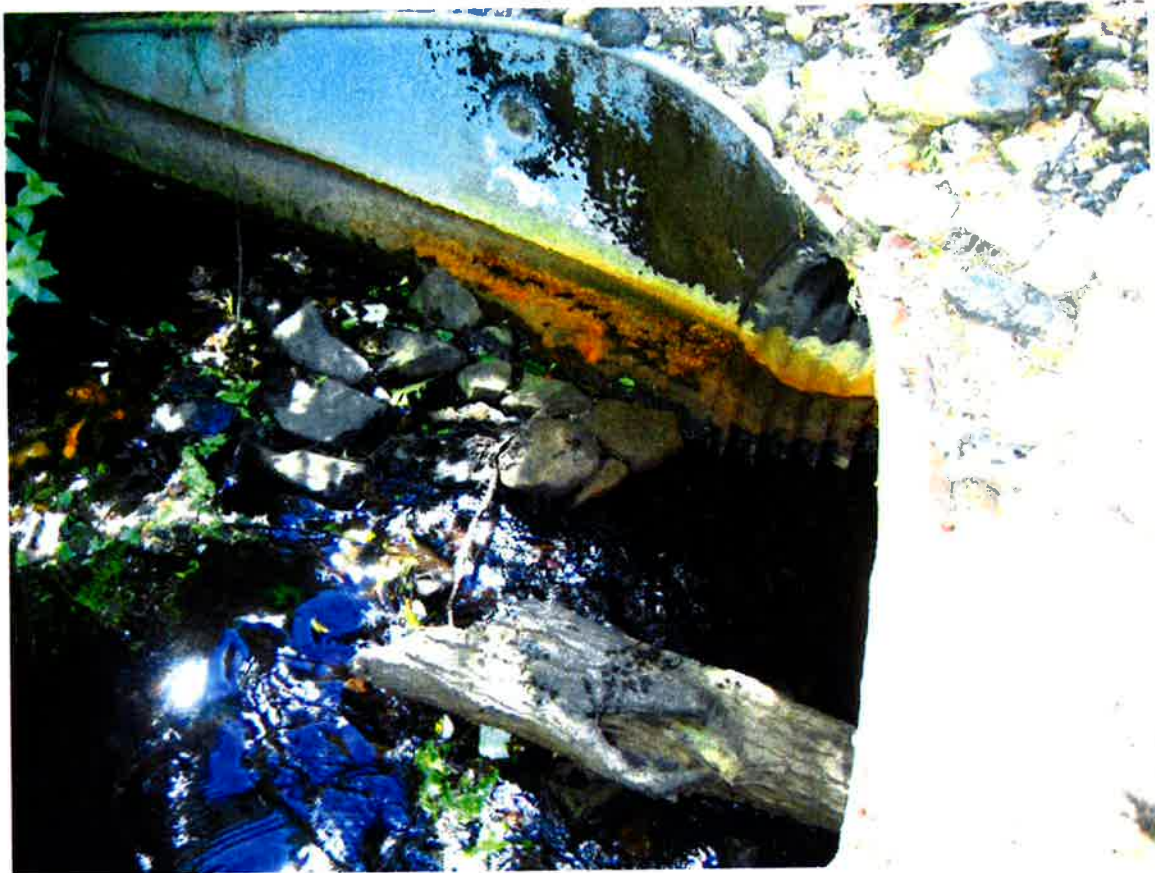
9. Typical Pipe and End Treatment Condition at Inlet
