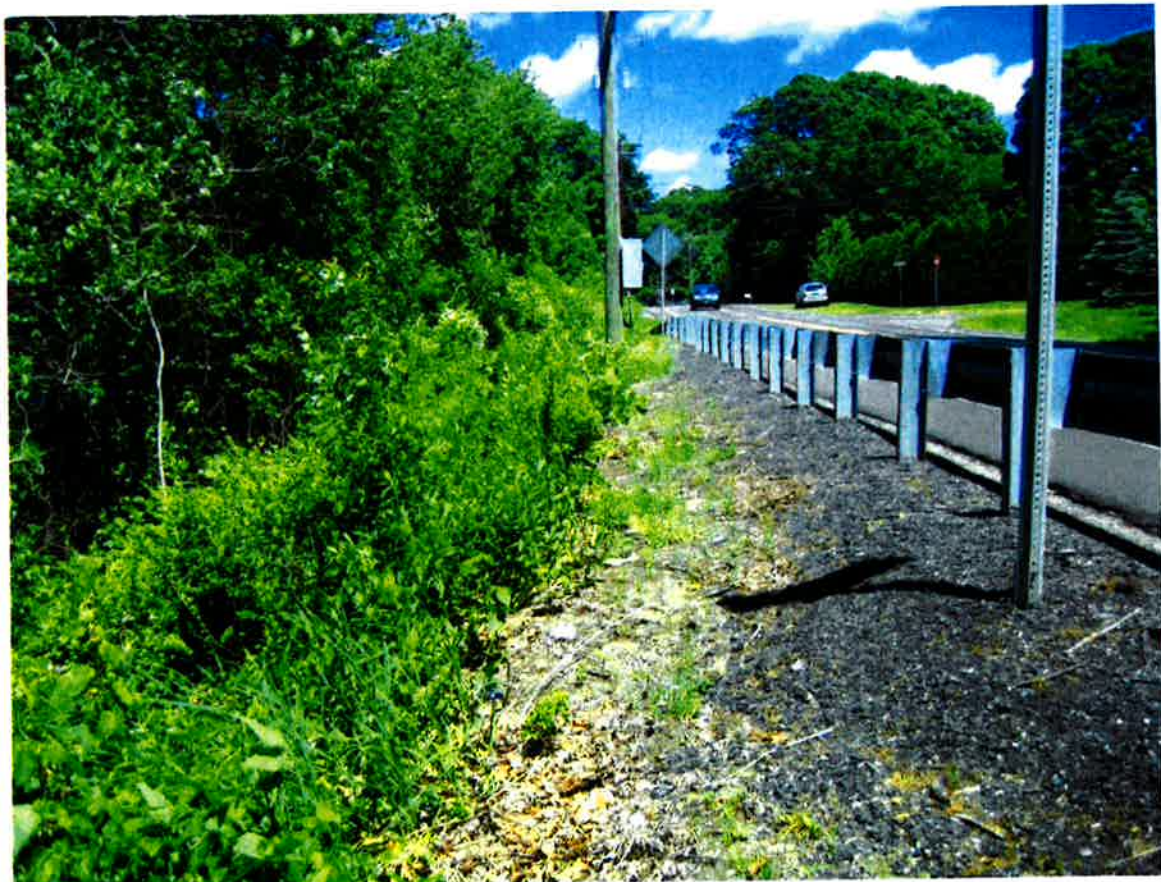
10. Typical Embankment Condition
