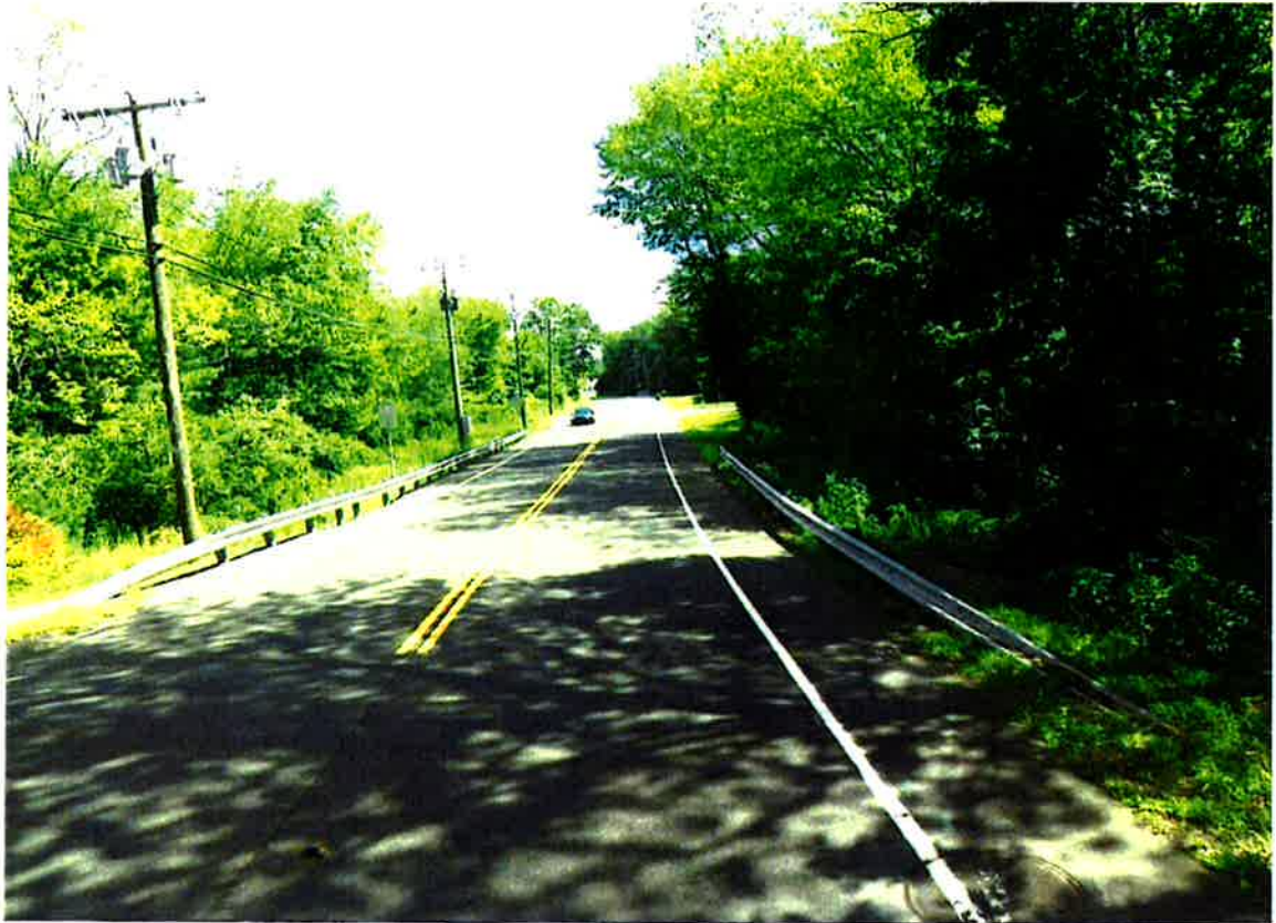
Image 2: View of Route 1 looking northward. The location of Structure #06676 is highlighted. Note the manhole on the shoulder, indicating a storm/sewer utility line.
