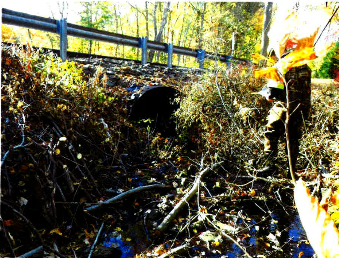
4. Downstream Elevation of Bridge No. 06676
