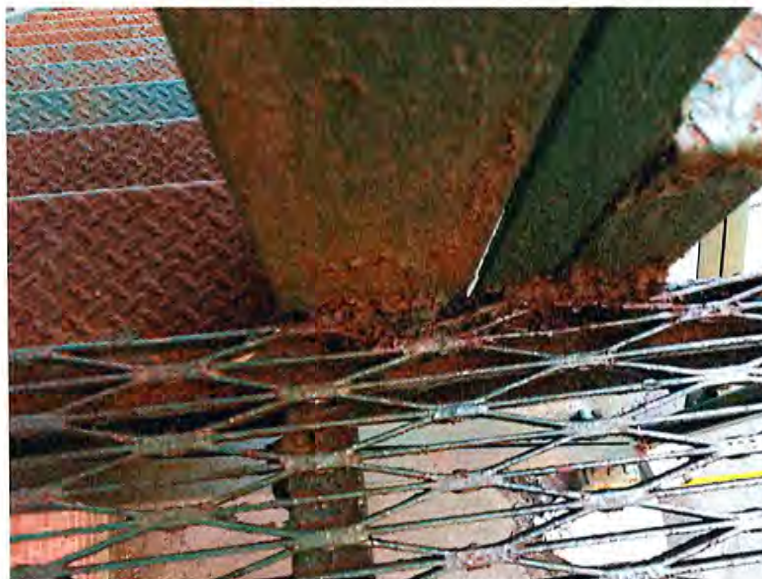
Figure 5: Connections at center of 1 st Floor Landing
