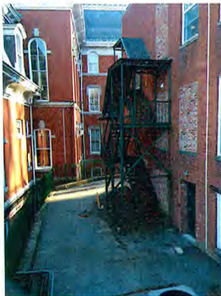
Figure 1: Overall View of Stairs and Landing
