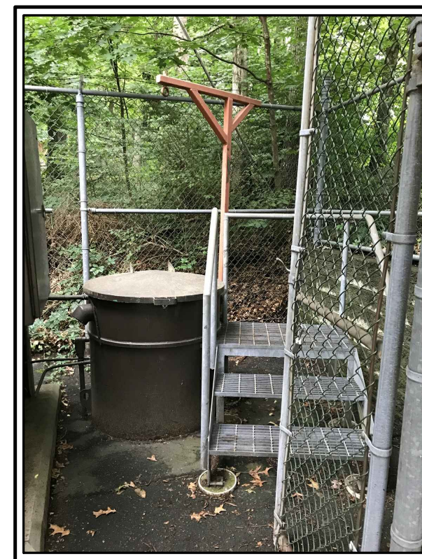
PHOTO ACCESS HATCH
