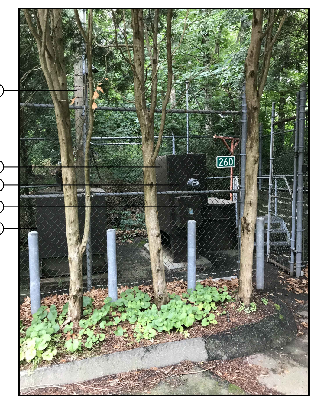
PHOTOGRAPH #2 PUMP STATION
