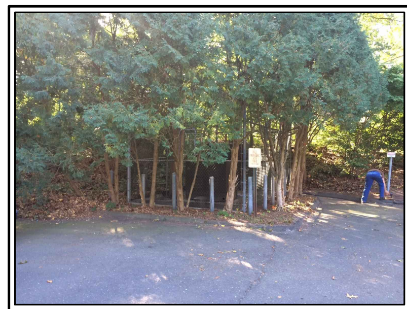
PHOTO PUMP STATION
