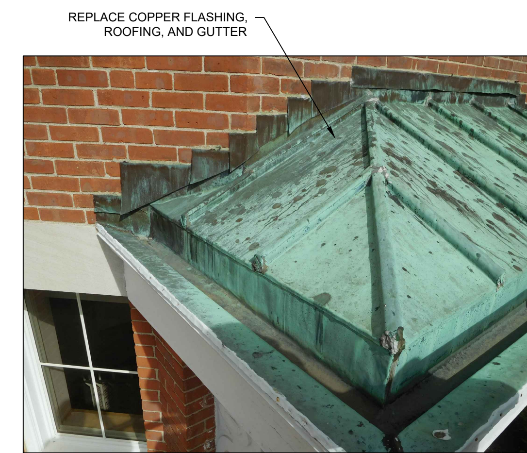
9 COPPER ROOF AT 1912 SOUTH ELEVATION SCALE: N.T.S.
