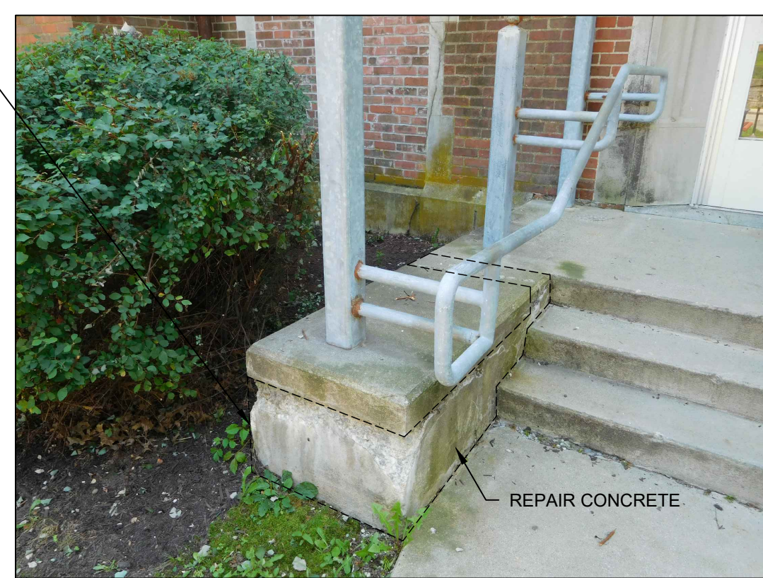
5 CONCRETE REPAIRS AT NORTH ELEVATION SUPPLEMENTAL BID #3 SCALE: N.T.S.
