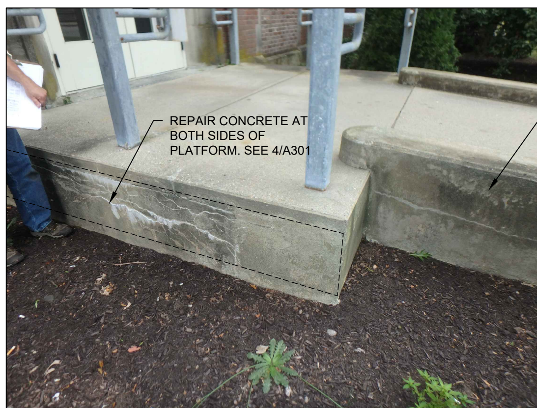
7 CONCRETE REPAIRS AT NORTH ELEVATION SUPPLEMENTAL BID #3 SCALE: N.T.S.
