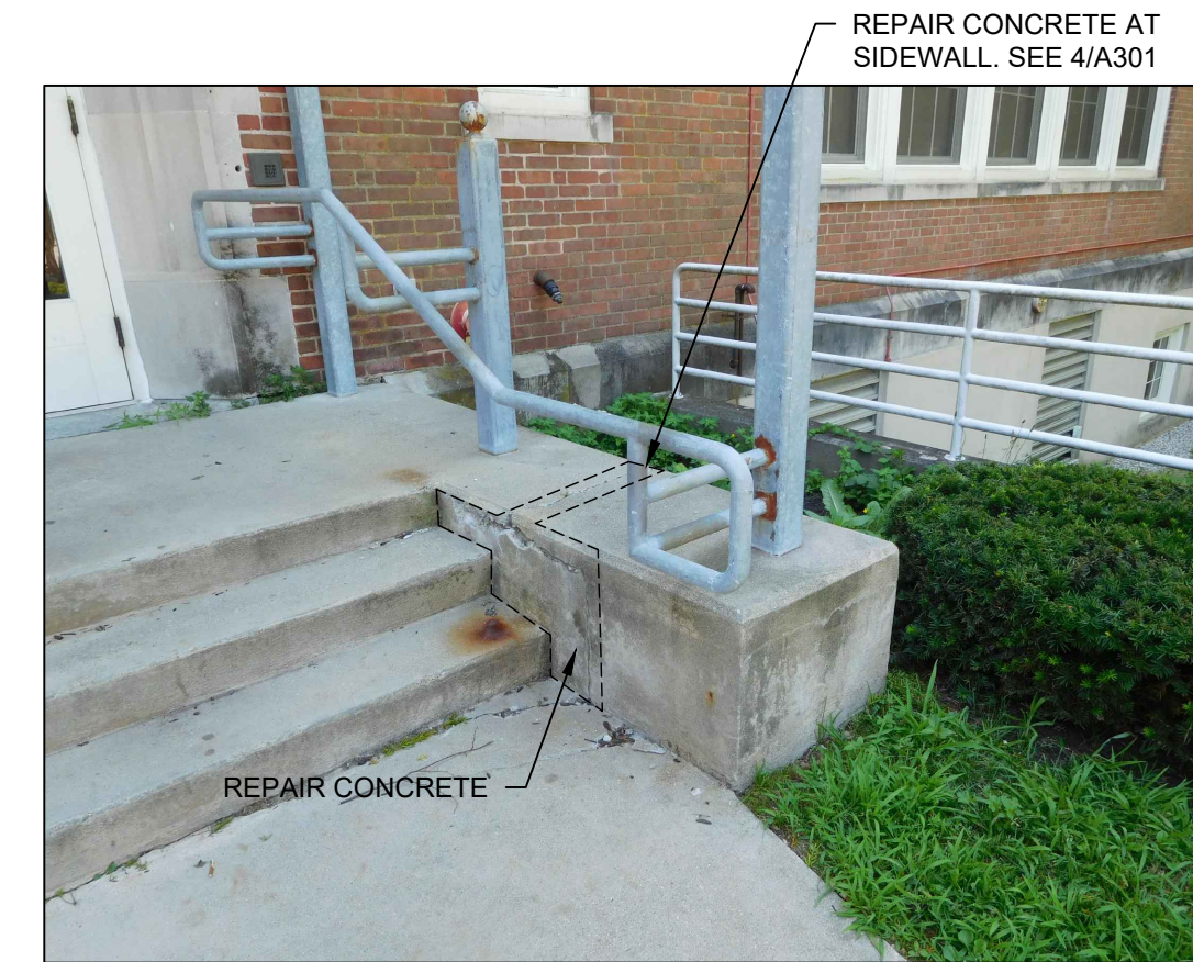
6 CONCRETE REPAIRS AT NORTH ELEVATION SUPPLEMENTAL BID #3 SCALE: N.T.S.
