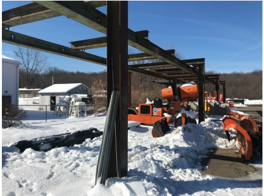
Jet Hanger Structure
