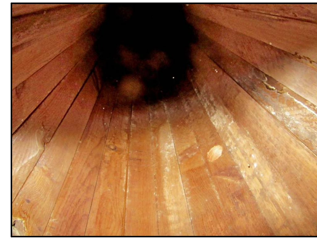
INTERIOR VIEW OF COLUMN LOOKING UPWARDS ALONG WOOD STAVES. PHOTO C02
