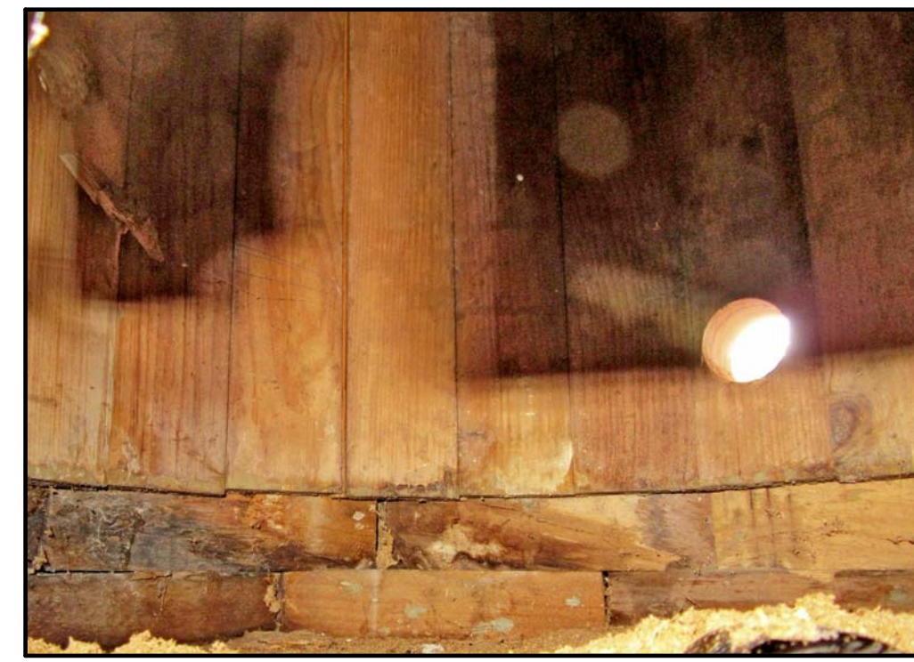
INTERIOR OF COLUMN BASE WITH VERTICAL STAVES AND 2 PART BULLNOSE BASE. NOTE VENTILATION HOLE IN SHAFT PHOTO C01
