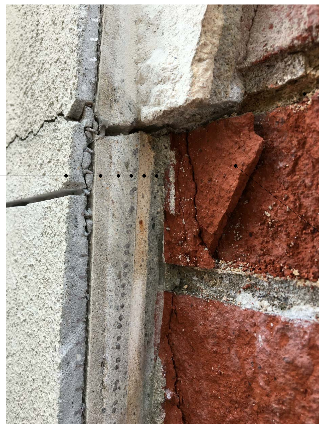
EXISTING STUCCO/PLASTER REMOVAL
