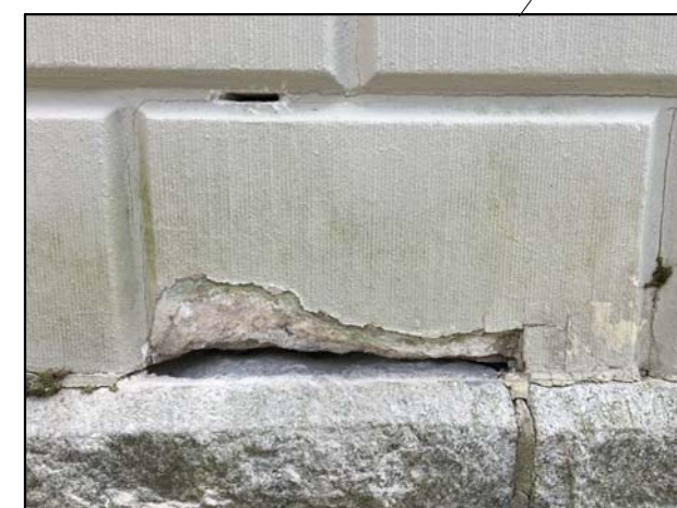
REMOVAL TEST PATCH OF DELAMINATED SURFACE/MORTAR JOINT OF PRECAST CONCRETE UNIT
