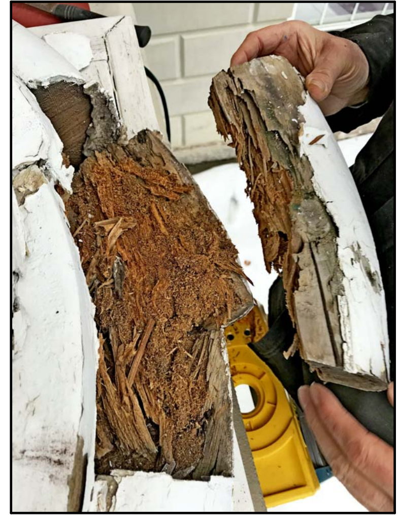
1/8 SEGMENT OF ROTTED BULLNOSE 2 PART BASE. ROTTED AND EASILY REMOVED BY HAND PHOTO C03
