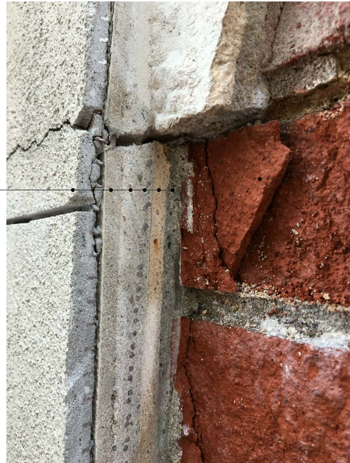
EXISTING STUCCO/PLASTER REMOVAL
