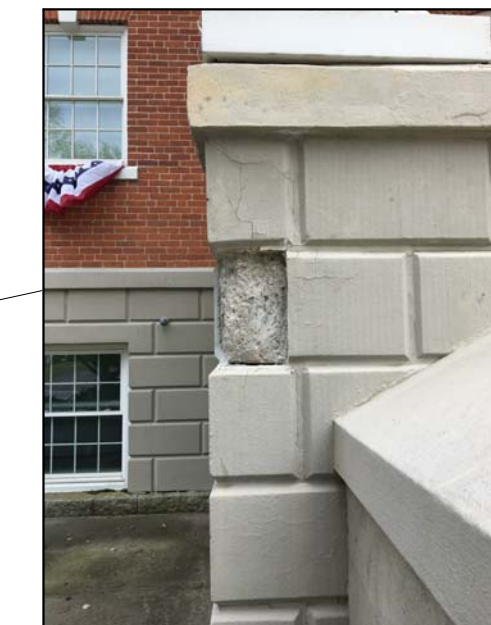
EXAMPLE OF REMOVAL OF DELAMINATED SURFACE OF PRECAST CONCRETE UNIT
