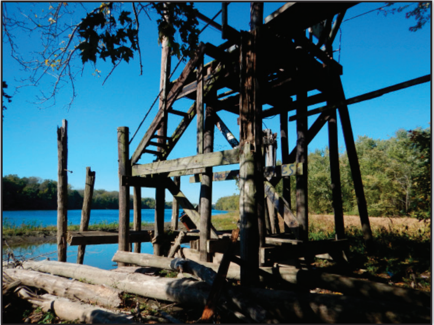
PHOTO 7. Looking north at piping support structure at edge of Connecticut River.
