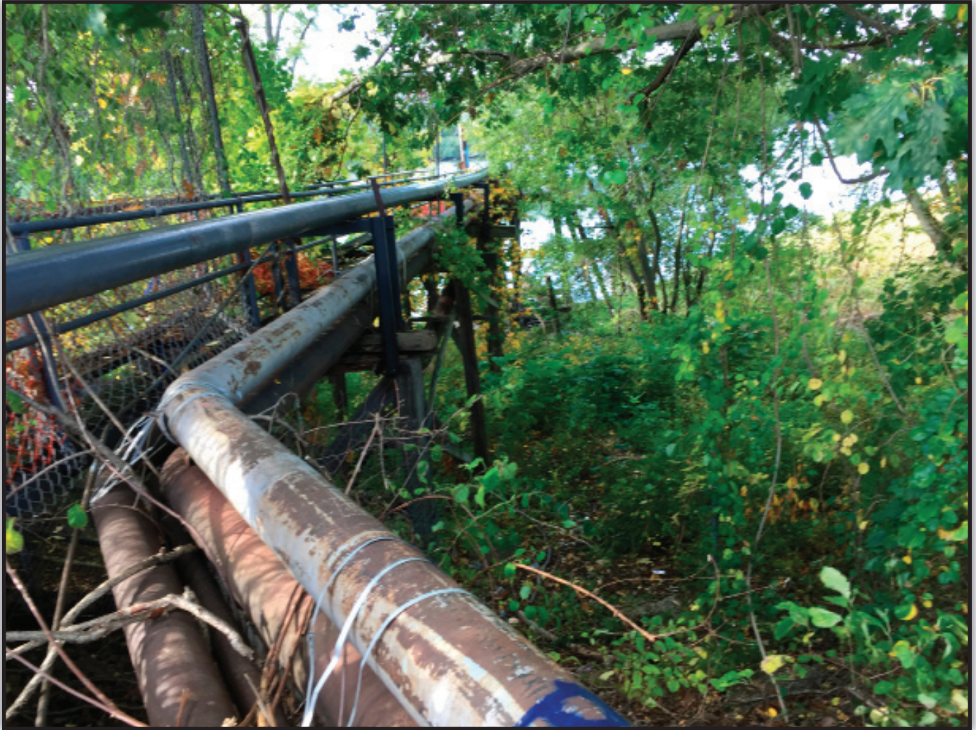
PHOTO 2. Looking west at historic terminal product transfer piping.
