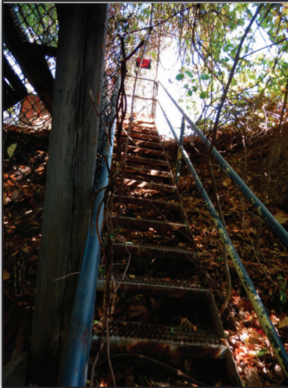
PHOTO 9. Steel staircase on southern side of piping support structure.
