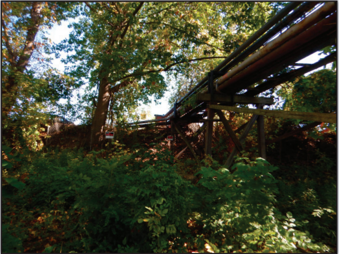
PHOTO 3. Looking east at piping and piping support structure.
