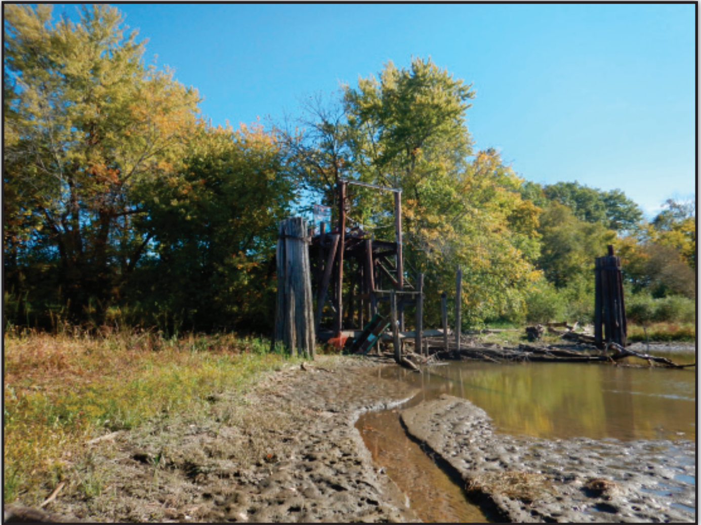
PHOTO 5. Looking southeast at piping and piping support from Connecticut River.
