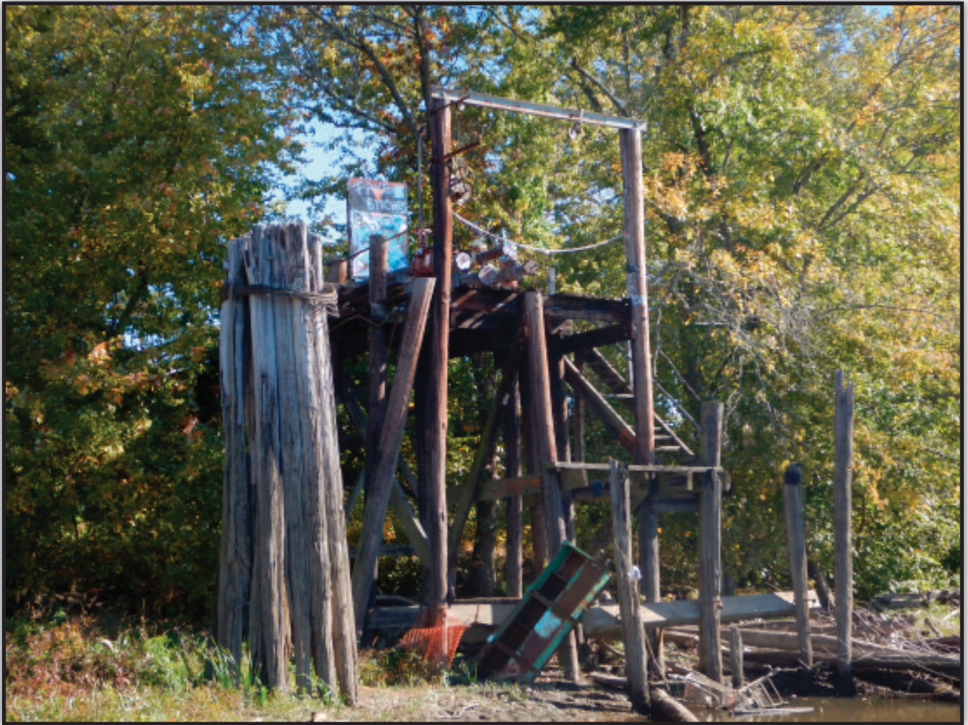
PHOTO 6. Looking southeast at piping and piping support from Connecticut River.
