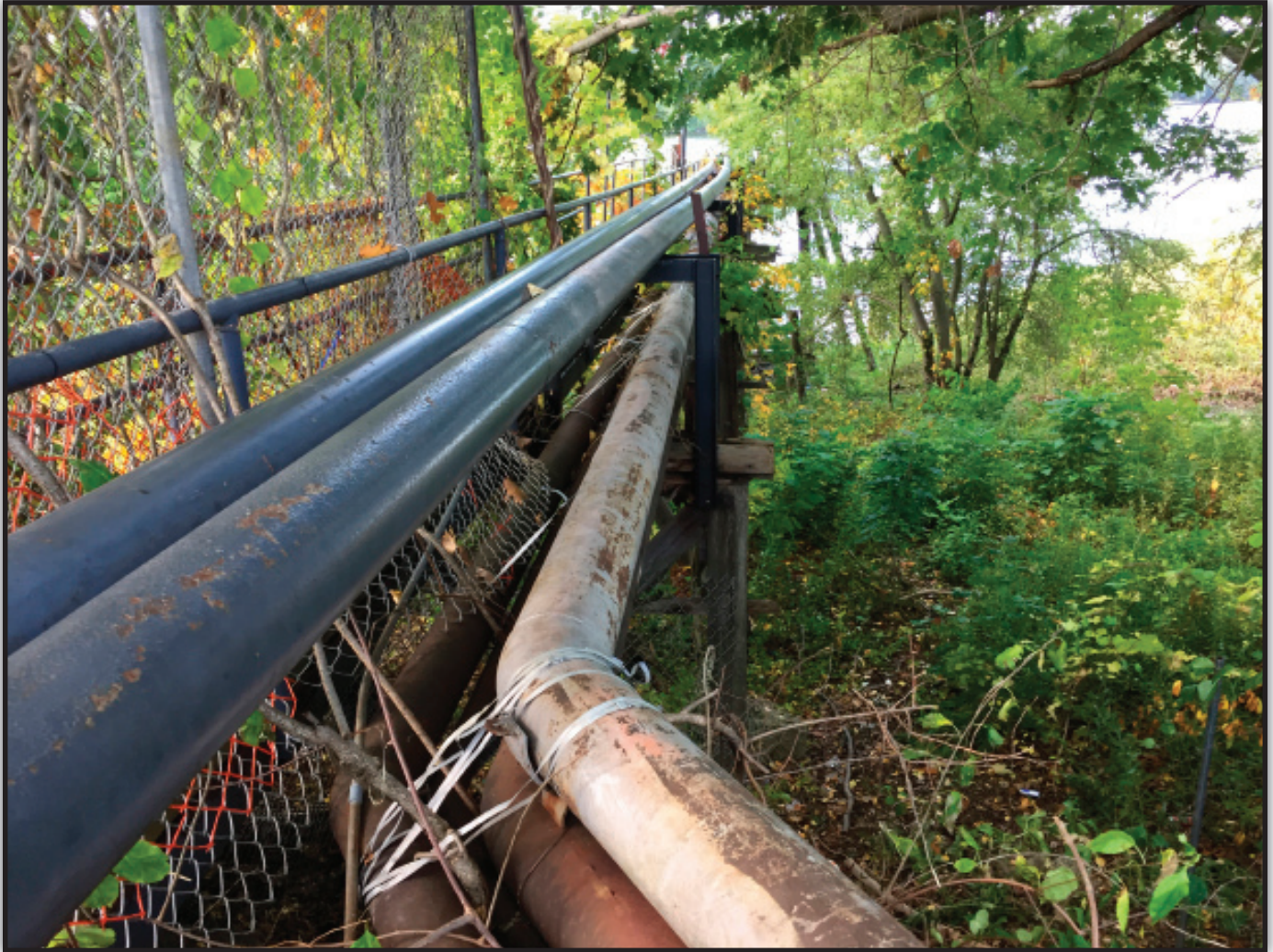
PHOTO 1. Looking west at historic terminal product transfer piping.
