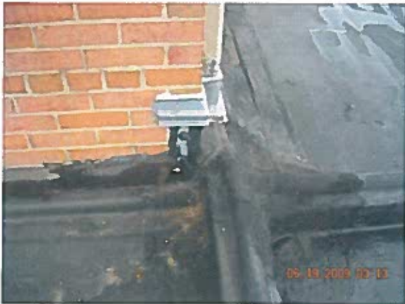
Area 1—Observation View of expansion joint termination at the wall
