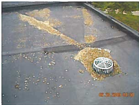
Area 5—Overview NOTE: Roof gravel was cleaned from roof surface
