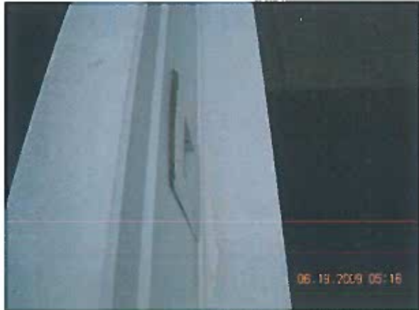
Area 9—Observation Outside view of roof scupper
