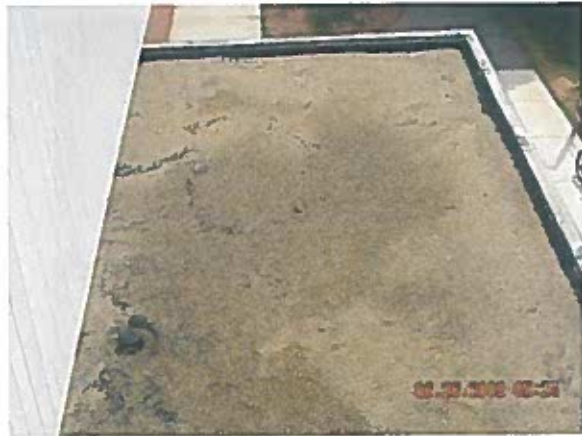
Gymnasium Area 3— Overview
