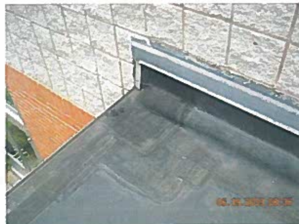
Area 8—Observations Terminations appear to be in satisfactory condition
