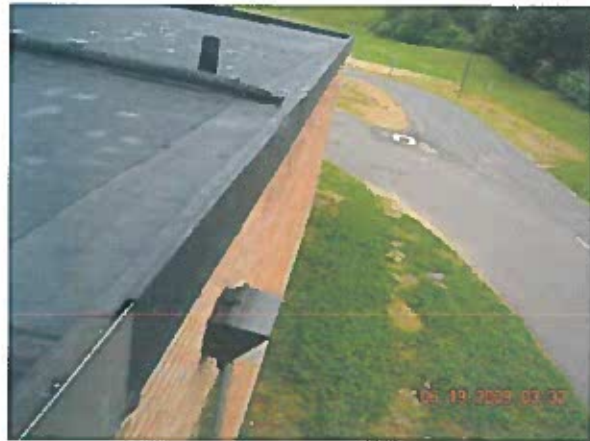
Area 2—Observation View of roof repair at roof modification
