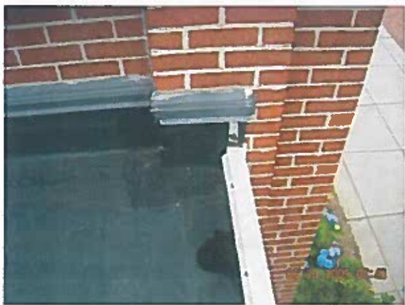
Area 6—Observation View of roof termination at wall
