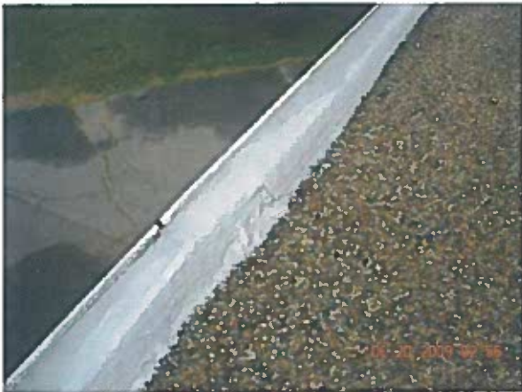
Area 1—Observation Outside perimeter edge repaired
