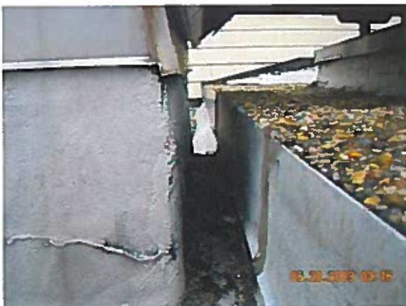
Area 2— Observation Limited flashing access
