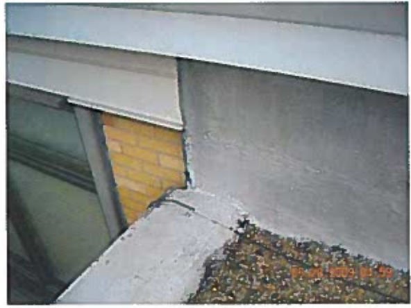
Area 10—Observation View of roof termination at wall flashing
