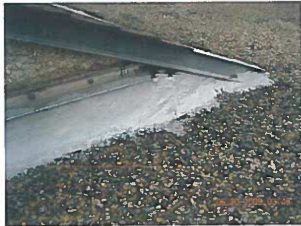
Area 4— Observation View of transition flashing
