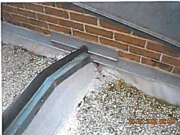
Area 3 — Observation Termination appears satisfactory
