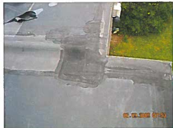
Area 2—Observation Terminations appear to be in satisfactory condition
