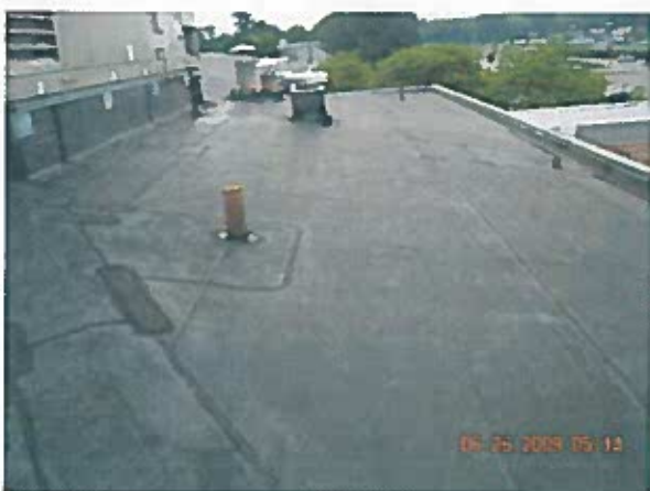
Gymnasium Area 1—Overview
