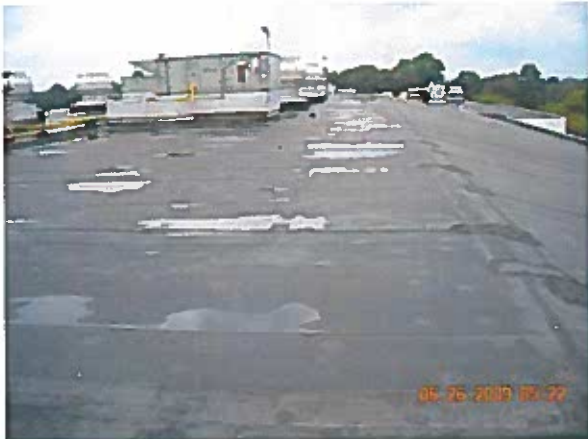
Gymnasium Area 2—Overview
