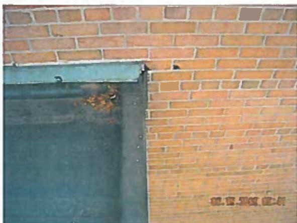
Area 11—Observation View of termination at wall
