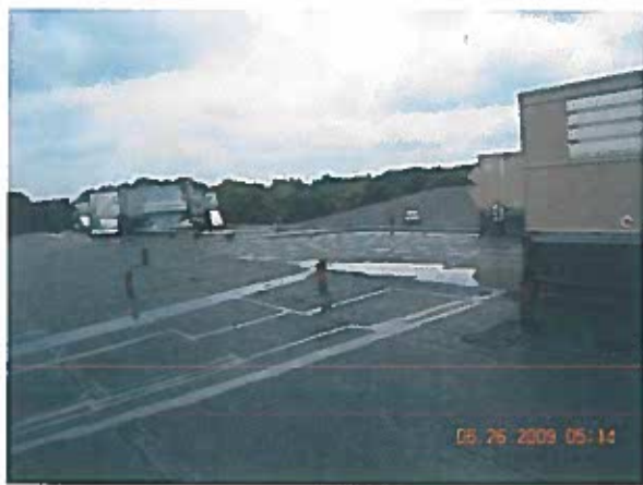
Gymnasium Area 1—Overview
