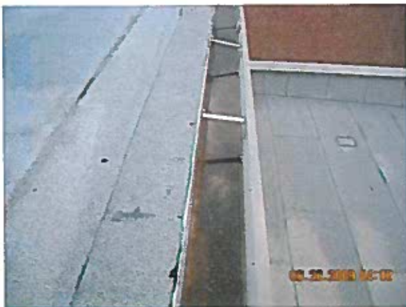
Area 9b — Overview Gutter detail on penthouse roof
