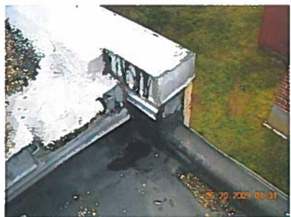
Area 5—Observation Roof termination
