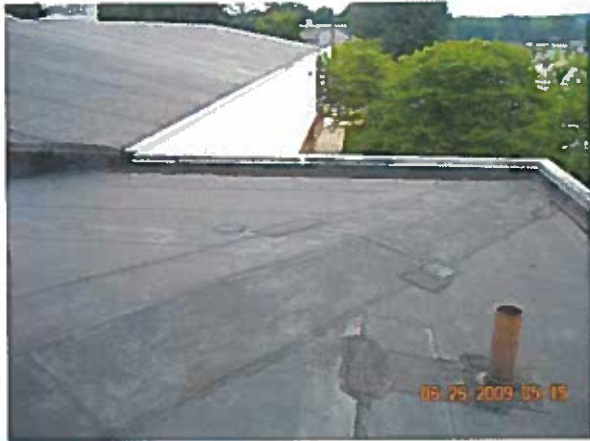
Gymnasium Area I—Overview
