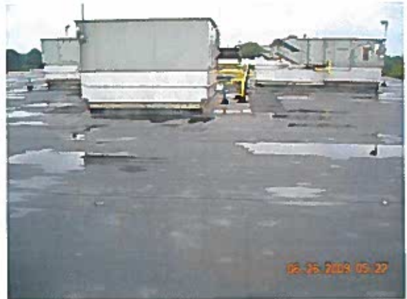
Gymnasium Area 2—Overview
