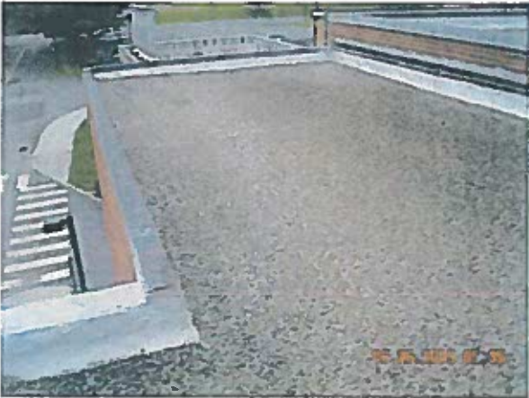
Gymnasium Area 6 — Overview
