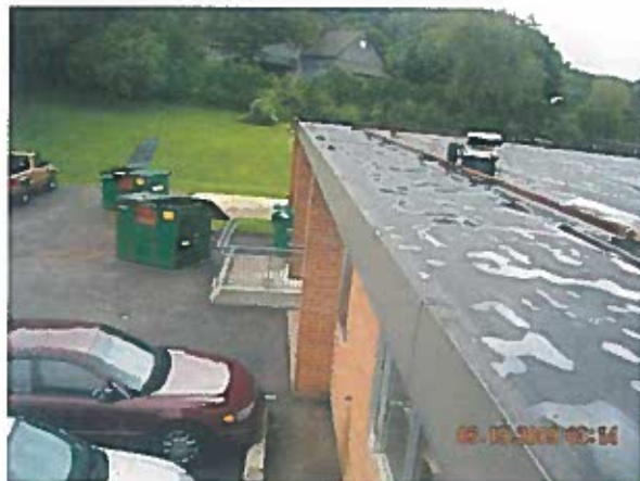
Area 1— Observation View of perimeter edge metal
