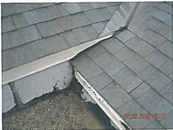
Area 2—Observation View of roof tie-in transition
