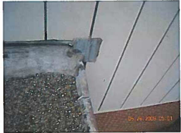
Area 24—Observation Base flashing terminations appear to be in satisfactory condition
