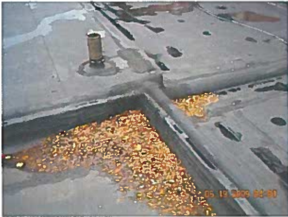
Area 4— Anomaly Debris was removed from the roof area
