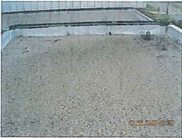
Gymnasium Area 6 — Overview
