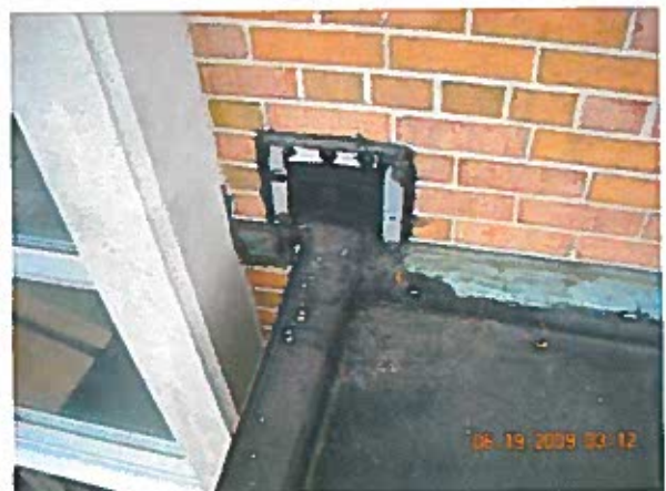
Area 1—Observation View of roof termination at wall
