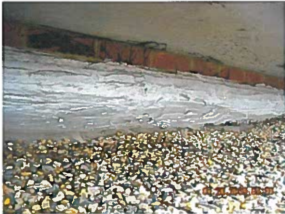
Gymnasium Area 4— Observation View of base flashings under cantilever
