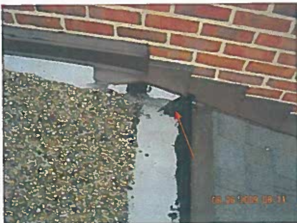
Area 3—Observation Built-up roof to shingle roof transition
