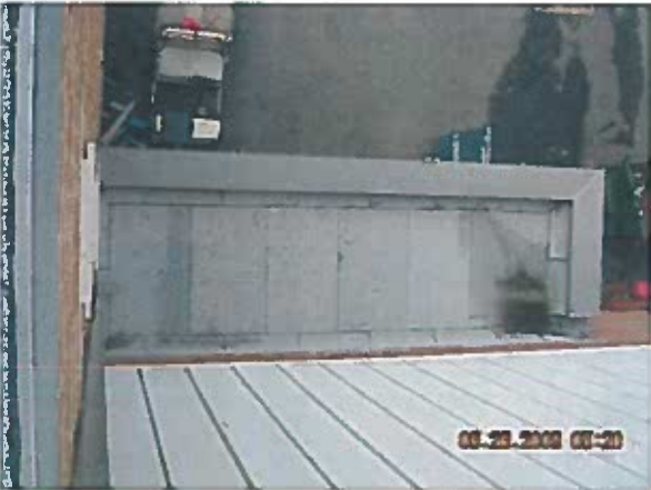
Gymnasium Area 1—Overview Lower roof area
