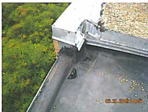
Area 5—Observation Roof termination
