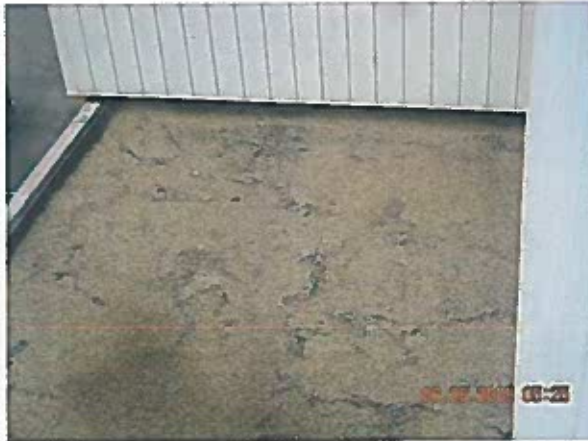
Gymnasium Area 3— Overview
