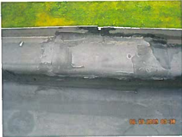
Area 2—Anomaly Splice patches repaired where applicable
