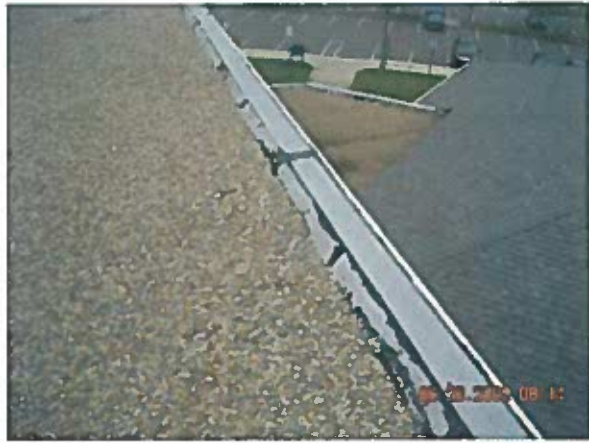
Area 6—Observation Built-up roof gravel edge detail
