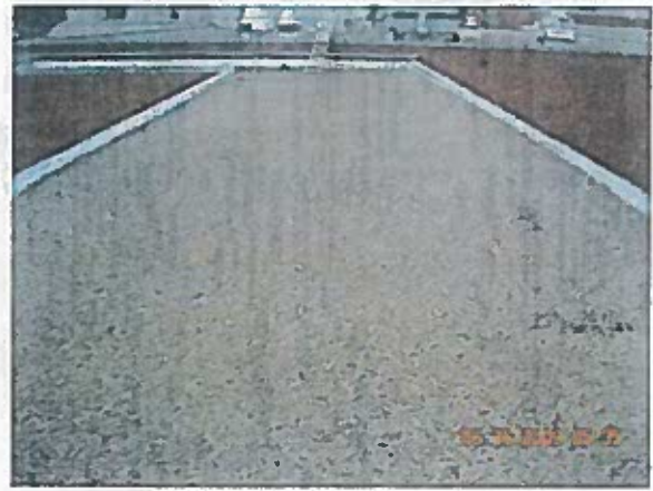
Gymnasium Area 6 — Overview
