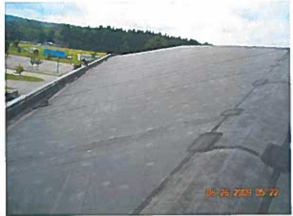
Gymnasium Area 2—Overview
