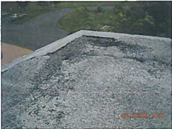
Area 16 — Overview View of edge metal detail
