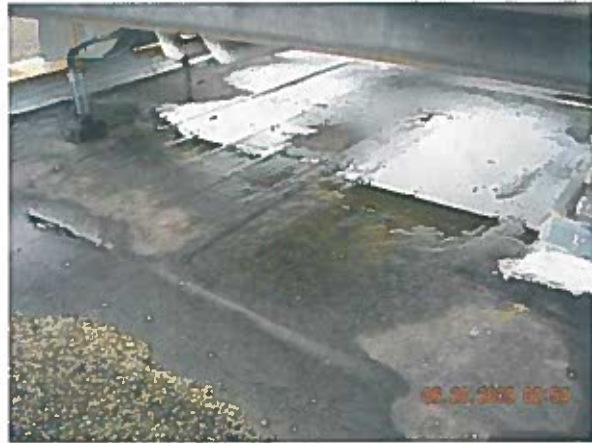
Area 1— Observation Repair patch installed beneath unit
