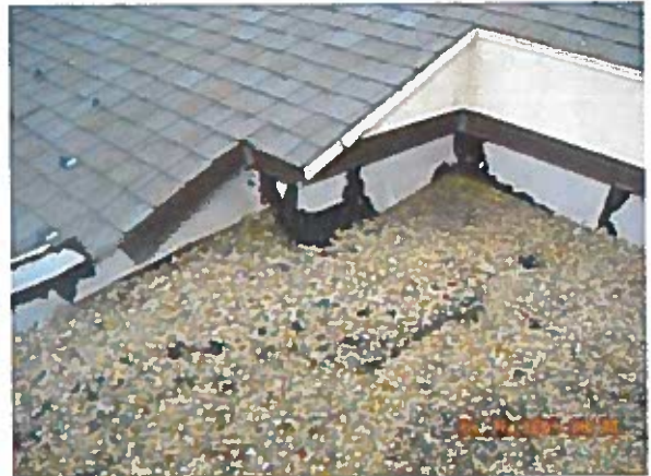
Area 8—Observation Built-up roof to asphalt shingle transition
