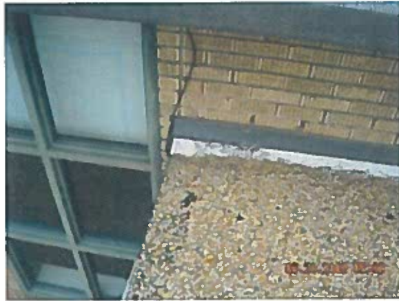
Area 11—Observation View of roof termination at wall
