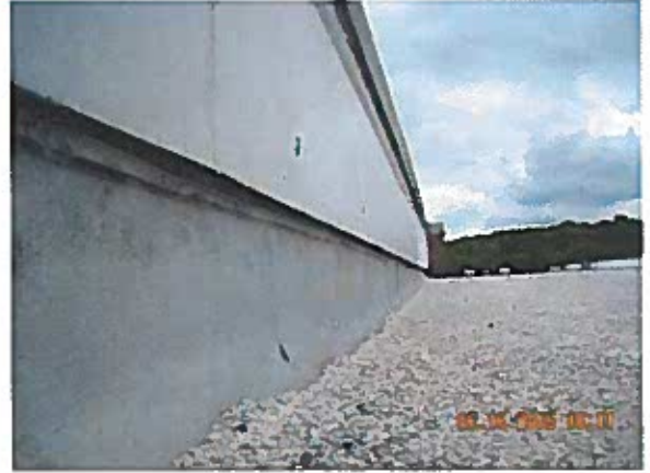
Area 17 — Observation Base flashings appear satisfactory
