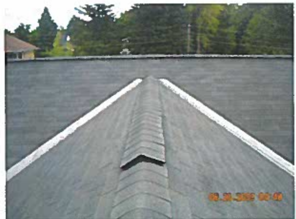
Area 6—Anomaly Ridge vent was resecured
