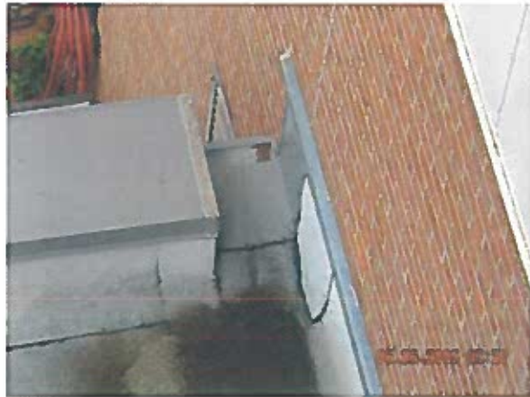
Gymnasium Area 1—Overview Scupper detail appears in satisfactory condition
