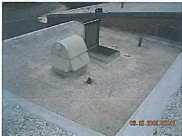
Area 2— Overview No apparent anomalies were observed at this roof area
