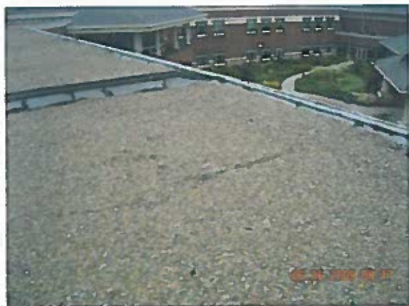
Area 7—Observation Built-up roof gravel edge to expansion joint detail
