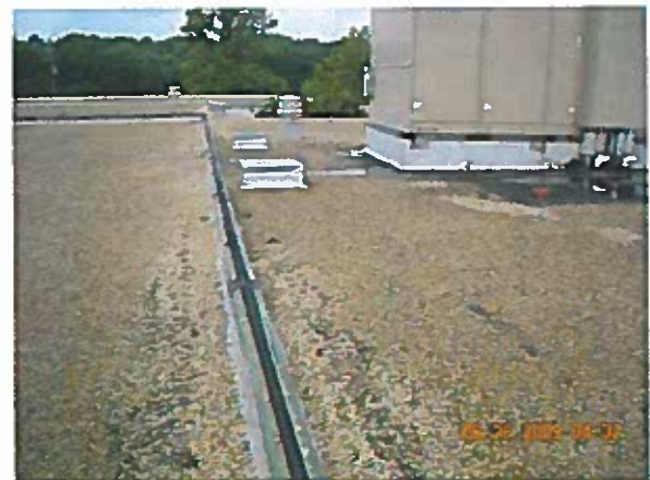
Area 15 — Observations Major repair was conducted around large A/C unit
