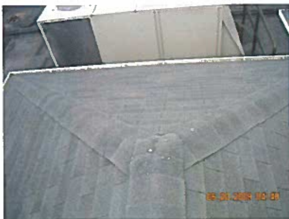
Area 6—Anomaly Hip to ridge shingle was resealed at both locations
