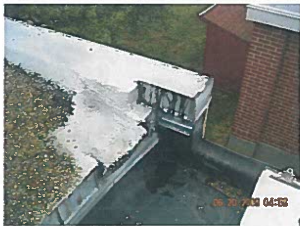
Area 10—Observation View of roof termination at drip edge
