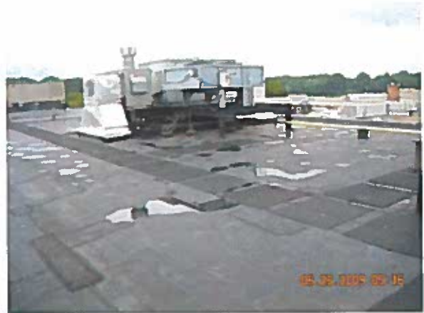
Gymnasium Area I—Overview
