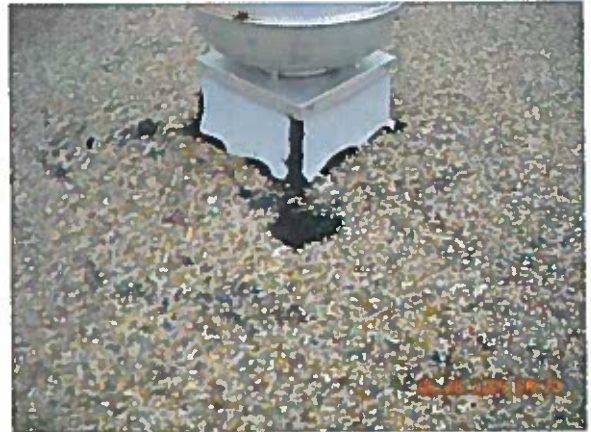
Area 8— Observation View of typical base flashing detail
