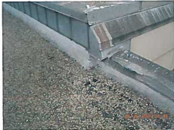
Area 11 — Overview of wall transitions
