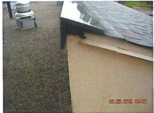
Area 5 —Observation Built-up roof to shingle roof transition
