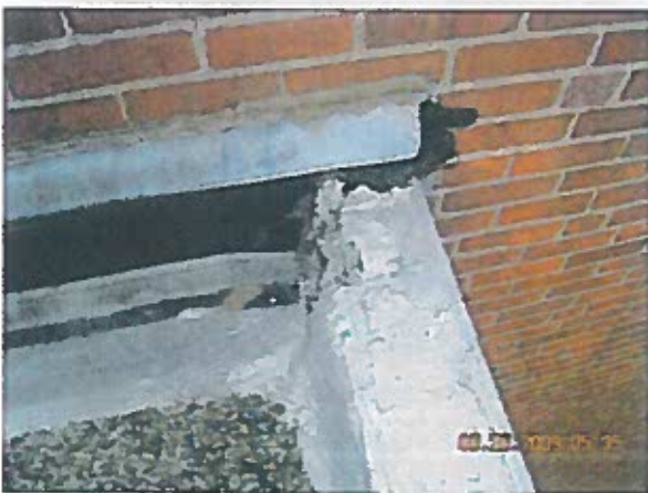
Gymnasium Area 5 — Observation View of expansion joint termination
