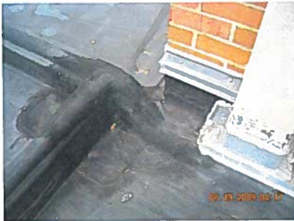
Area 5— Observation View of expansion joint at wall transition
