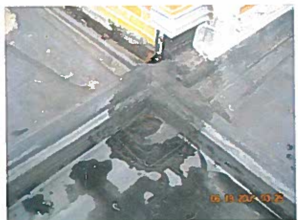
Area 2—Observation View of expansion joint at wall transition
