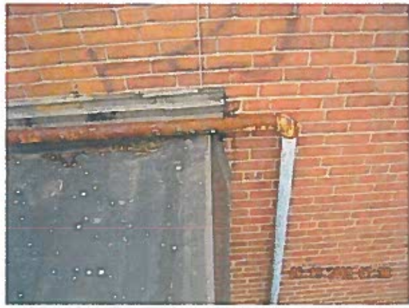
Area 1—Observation Terminations appear to be in satisfactory condition
