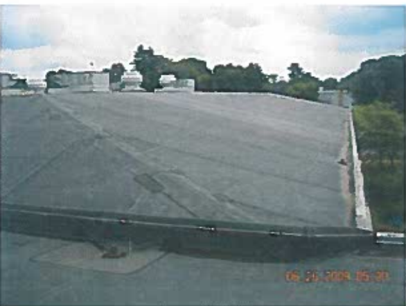
Gymnasium Area 2—Overview
