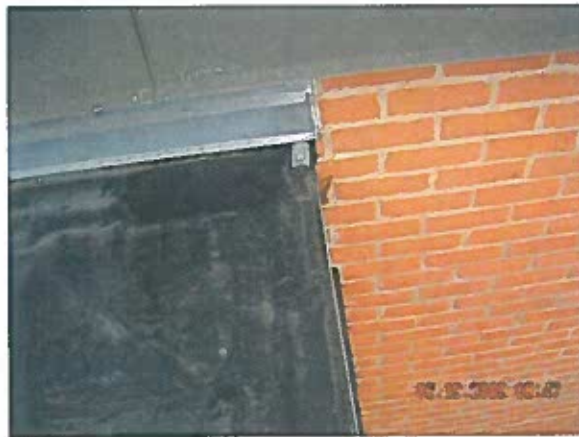
Area 10—Observations Terminations appear to be satisfactory
