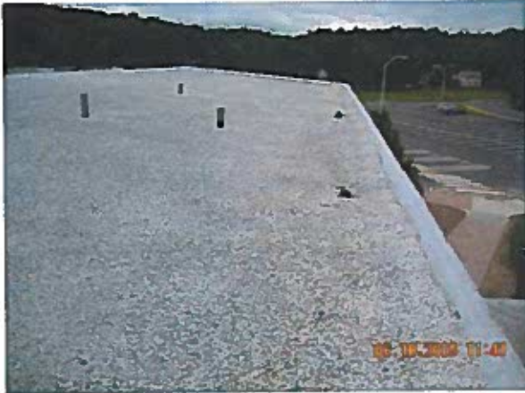
Area 9—Overview No apparent anomalies were observed
