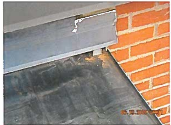
Area 7 — Observations Terminations appear satisfactory
