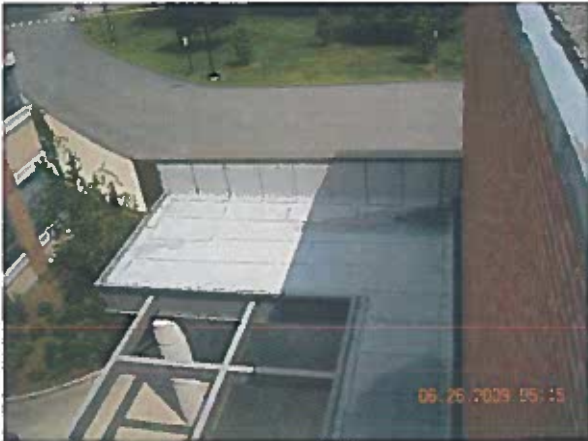
Area 9c & d — Overview
