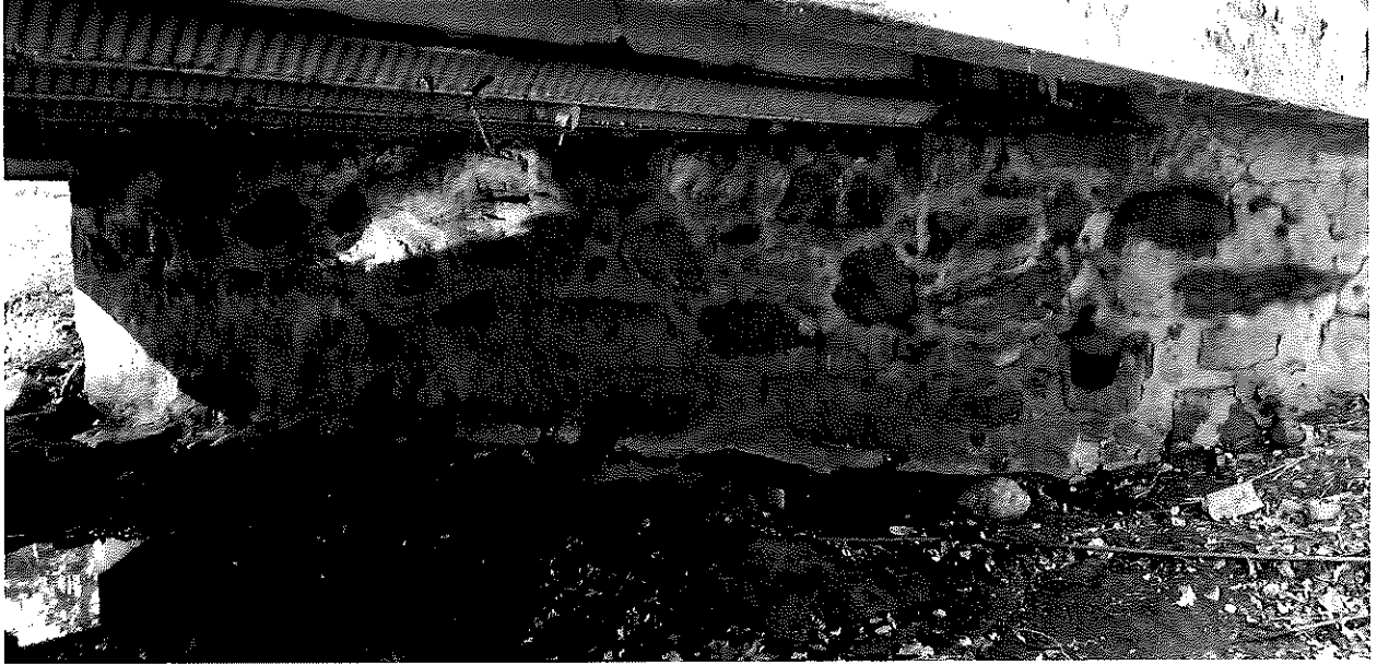
Deteriorating Bridge No. 02559 Superstructure
