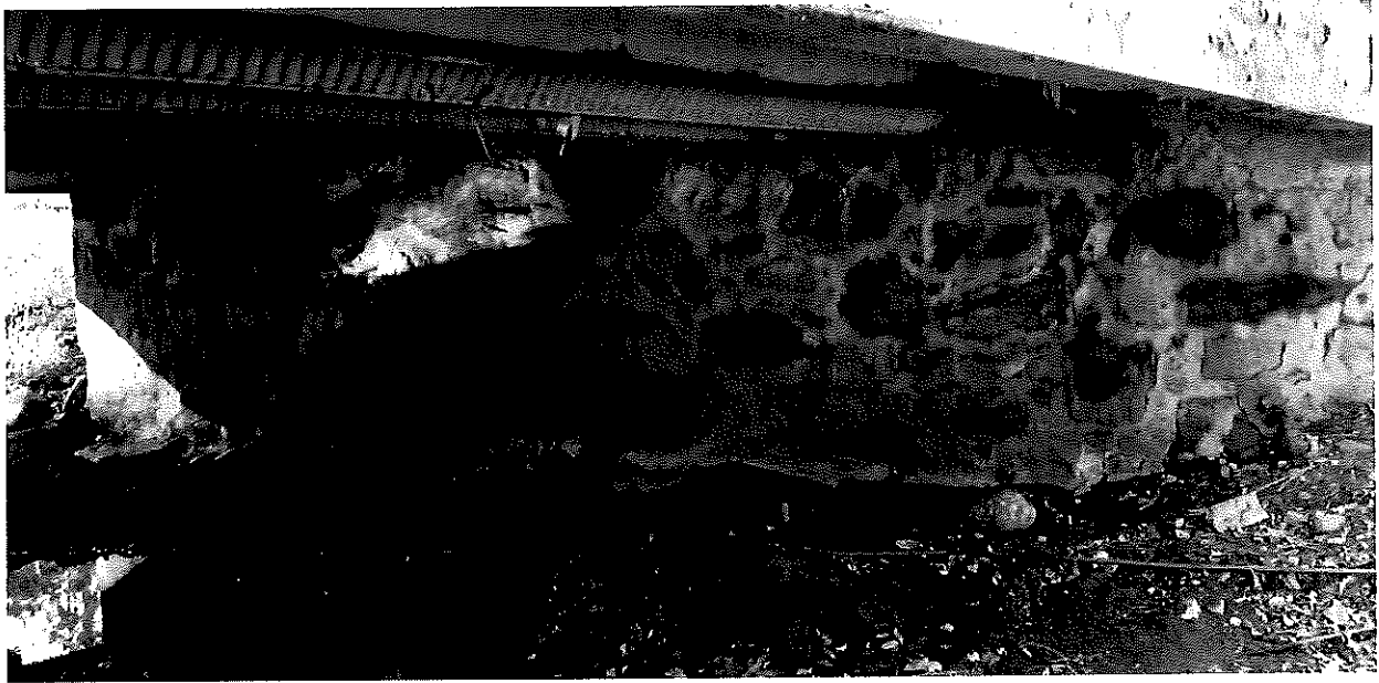
Deteriorating Bridge No. 02559 Superstructure
