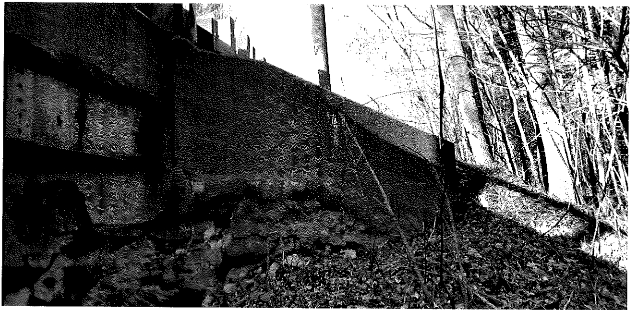
Southern Inlet Wingwall
