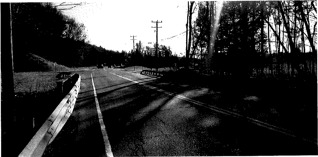
Area Overview Looking Southbound
