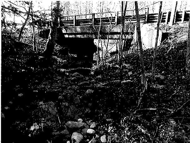
Looking downstream towards Bridge 02559
