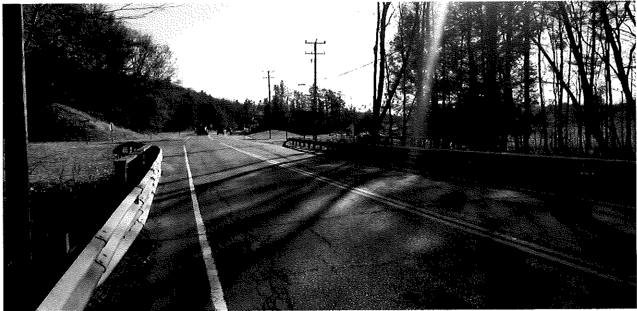
Area Overview Looking Southbound
