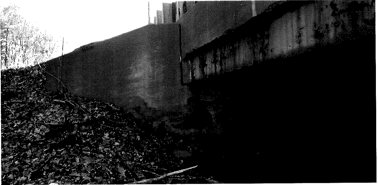
Northern Inlet Wingwall
