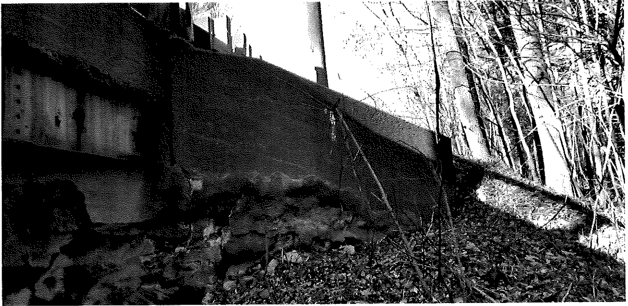
Southern Inlet Wingwall
