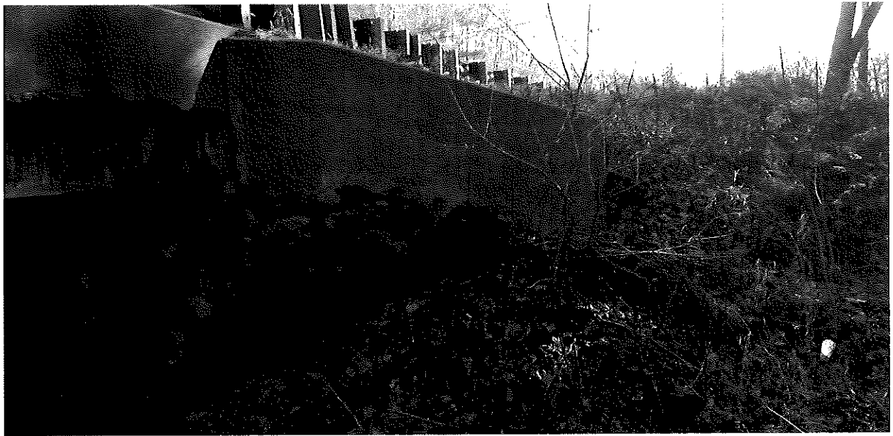
Northern Outlet Wingwall
