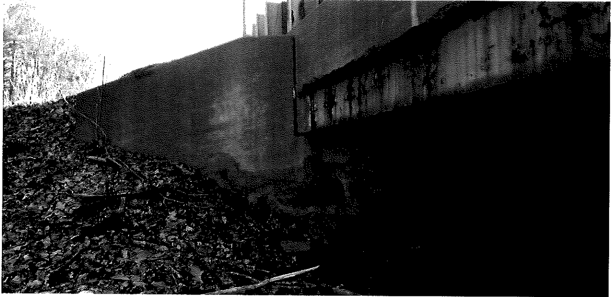
Northern Inlet Wingwall
