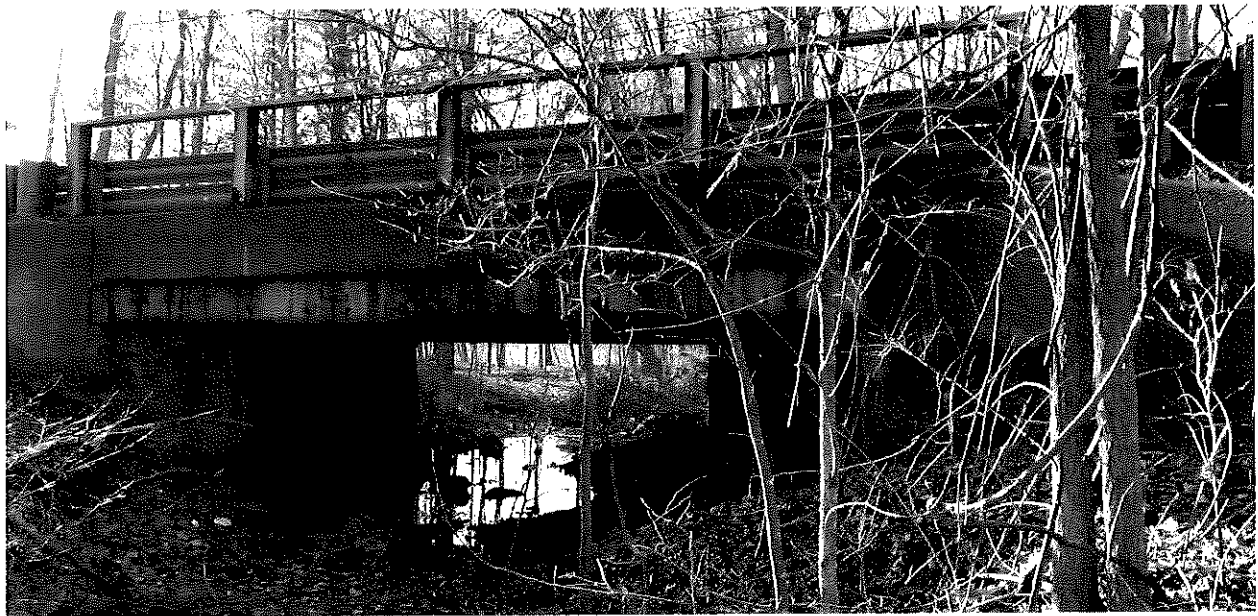
Bridge No. 02559 Inlet
