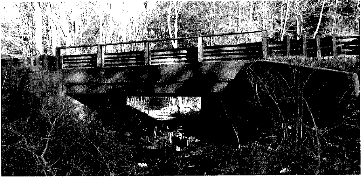
Bridge No. 02559 Outlet
