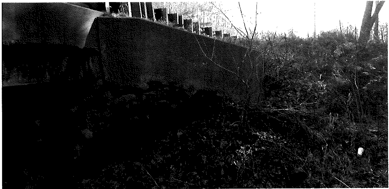
Northern Outlet Wingwall
