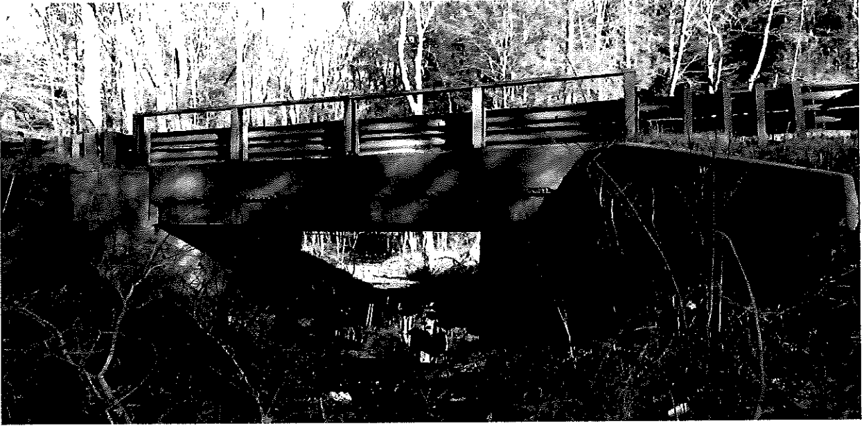
Bridge No. 02559 Outlet
