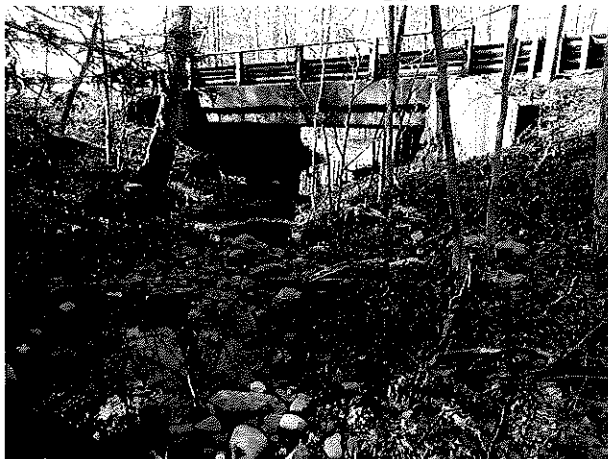
Looking downstream towards Bridge 02559
