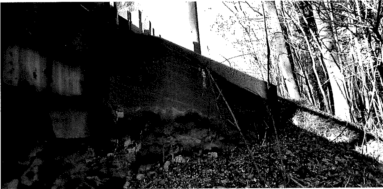
Southern Inlet Wingwall
