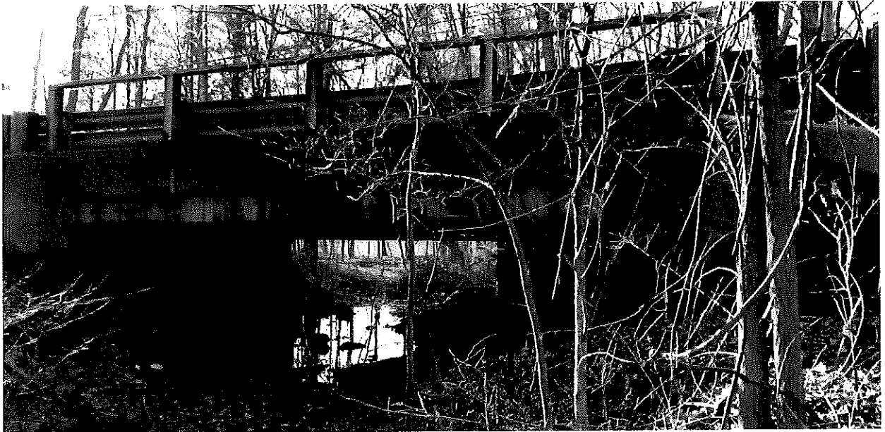
Bridge No. 02559 Inlet
