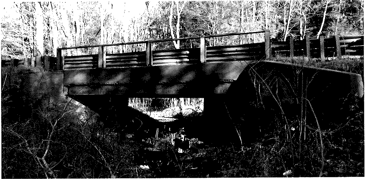
Bridge No. 02559 Outlet
