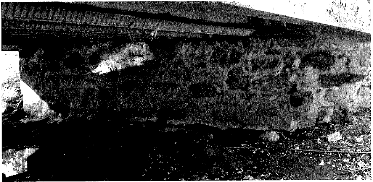
Deteriorating Bridge No. 02559 Superstructure
