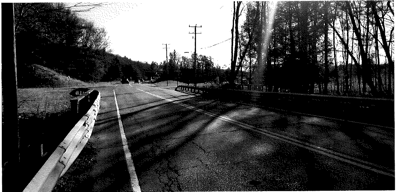
Area Overview Looking Southbound
