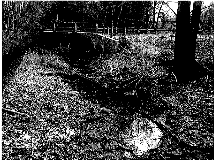
Looking upstream towards Bridge 02559
