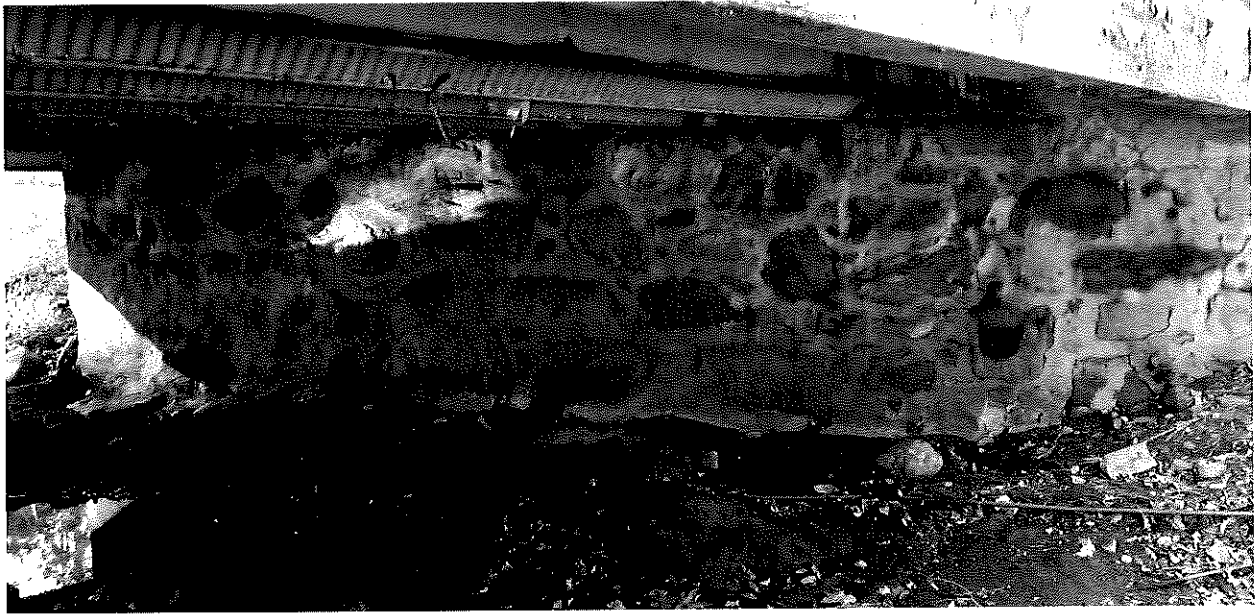
Deteriorating Bridge No. 02559 Superstructure
