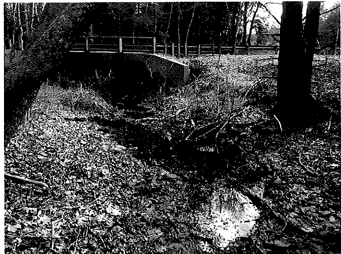
Looking upstream towards Bridge 02559
