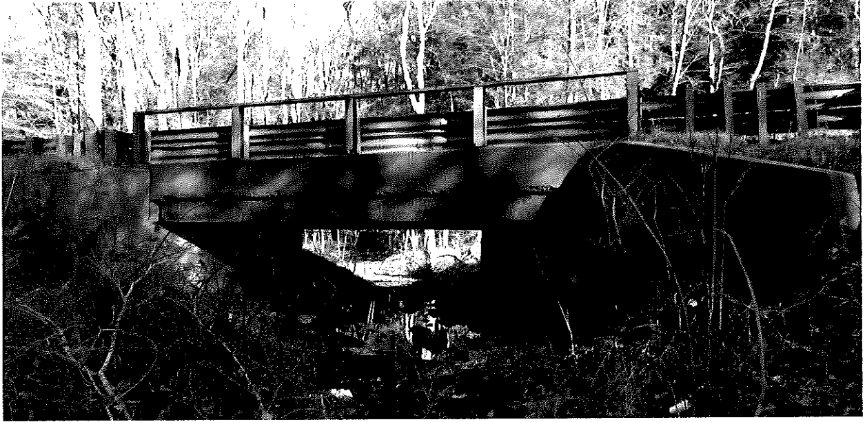
Bridge No. 02559 Inlet
