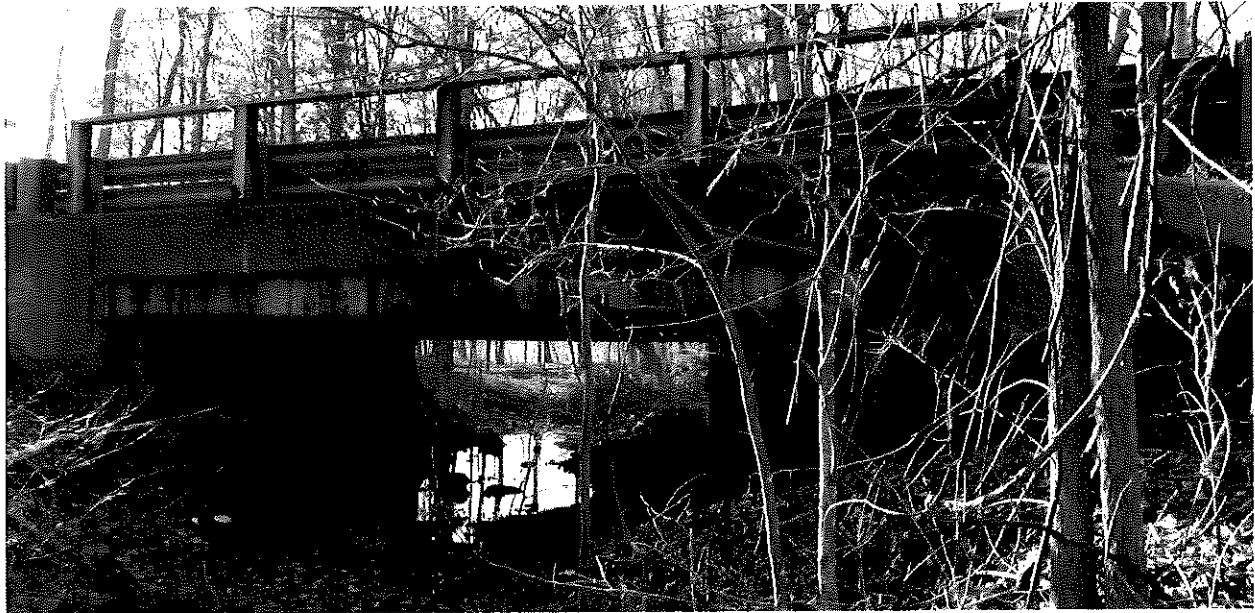
Bridge No. 02559 Outlet
