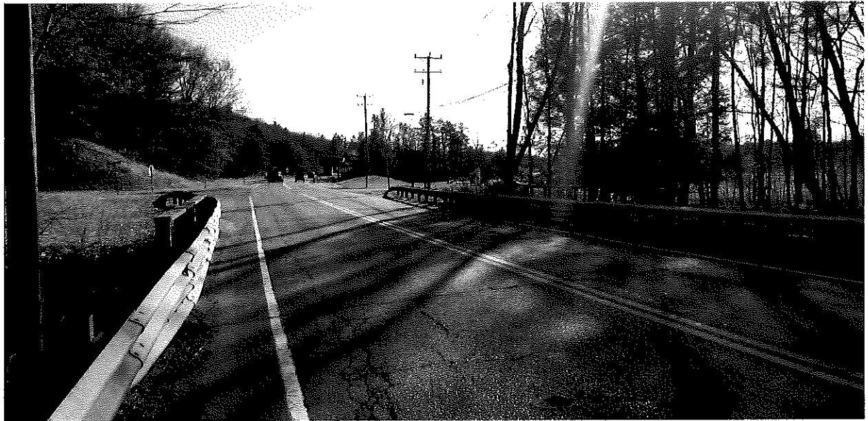
Area Overview Looking Southbound
