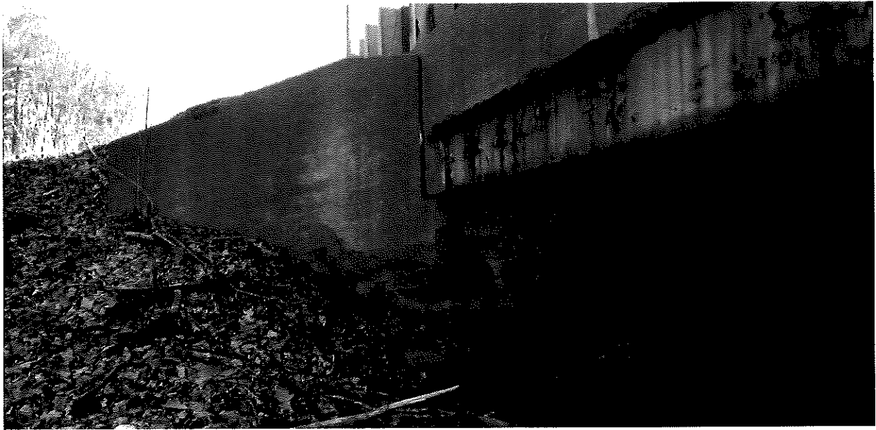
Northern Outlet Wingwall
