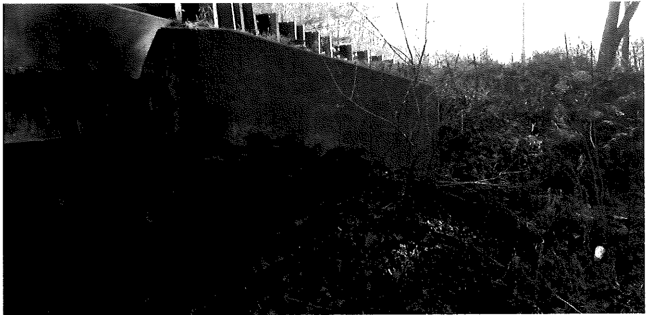
Northern Inlet Wingwall
