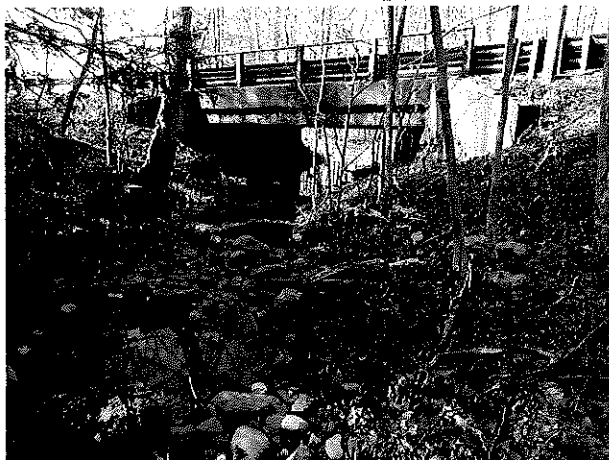
Looking downstream towards Bridge 02559
