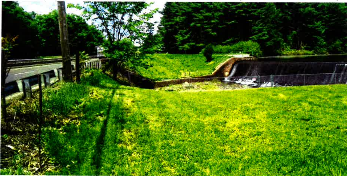
2. Dam upstream of Bridge No. 00948
