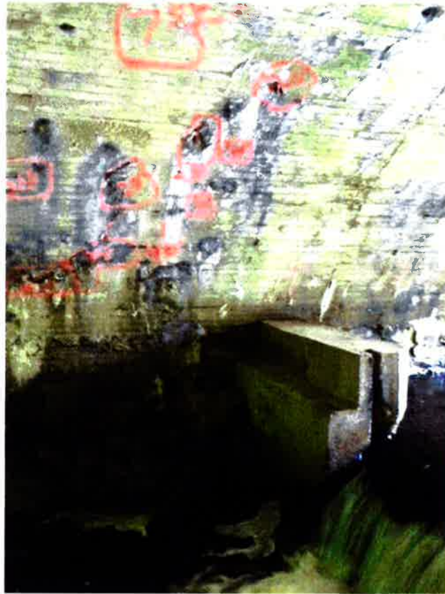
7. Typical condition of mortar veneer
