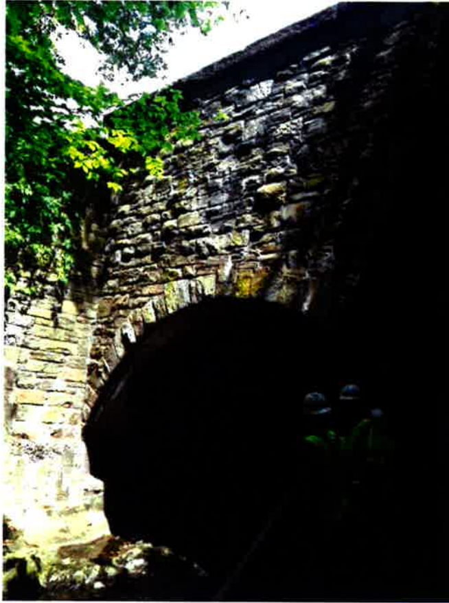
1. Downstream elevation of Bridge No. 00948
