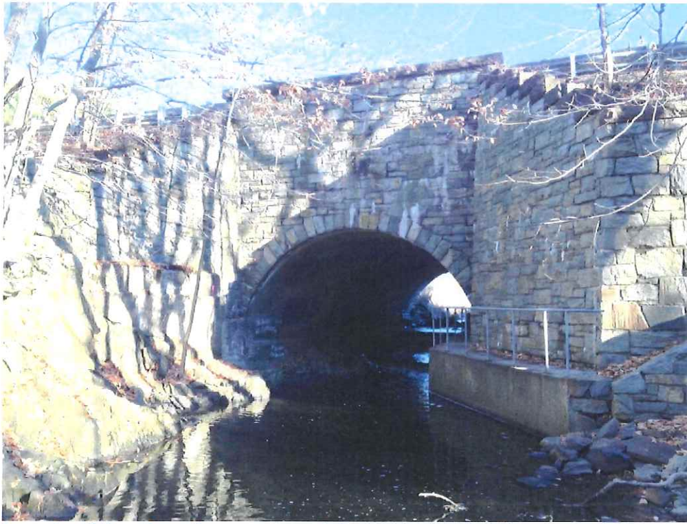
Image 1: 1940 southern (downstream) spandrel of Bridge #00948. The masonry clad concrete structure includes a staircase and walkway that provides access from the hiking trails to the underside of the bridge.
