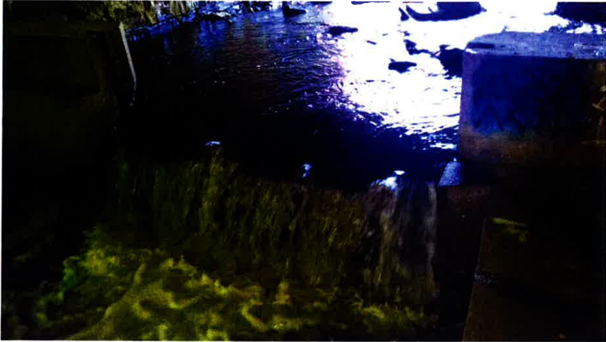
5. Weir under Bridge No. 00948
