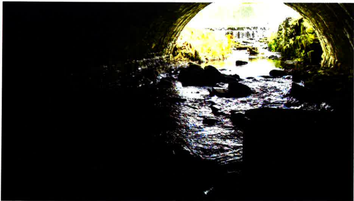
4. Looking upstream from Bridge No. 00948
