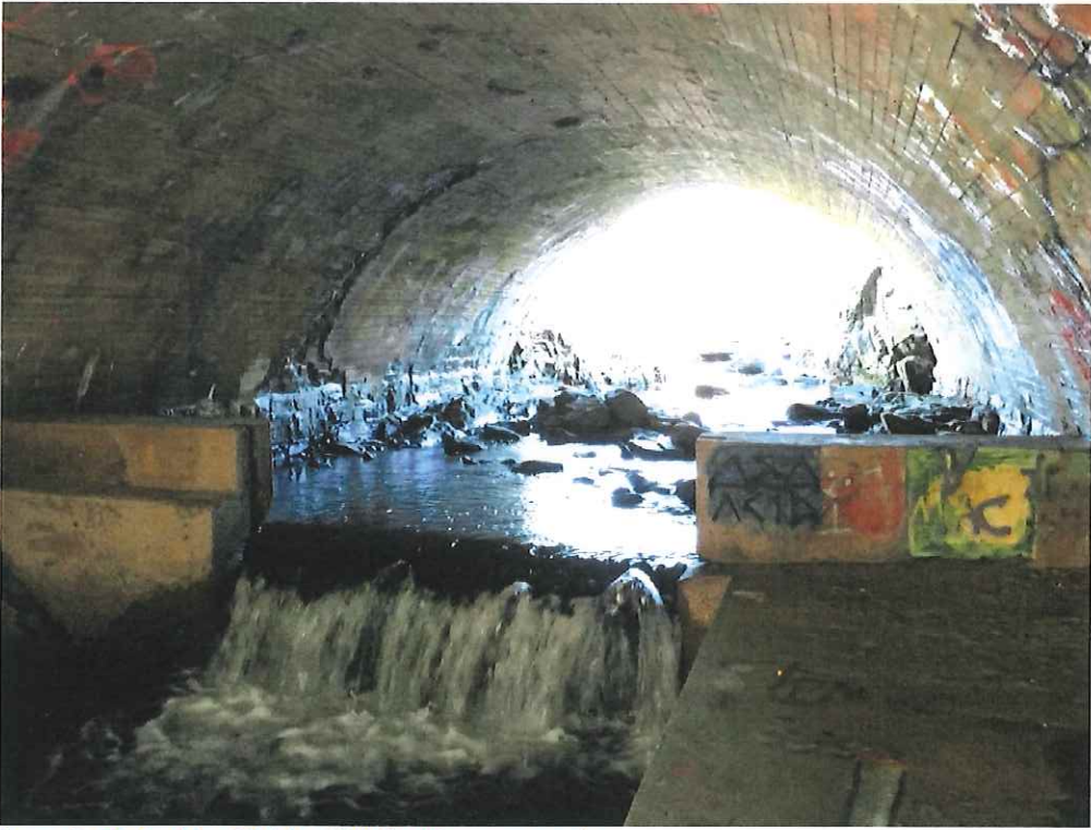
Image 2: Underside of Bridge #00948 with concrete weir.
