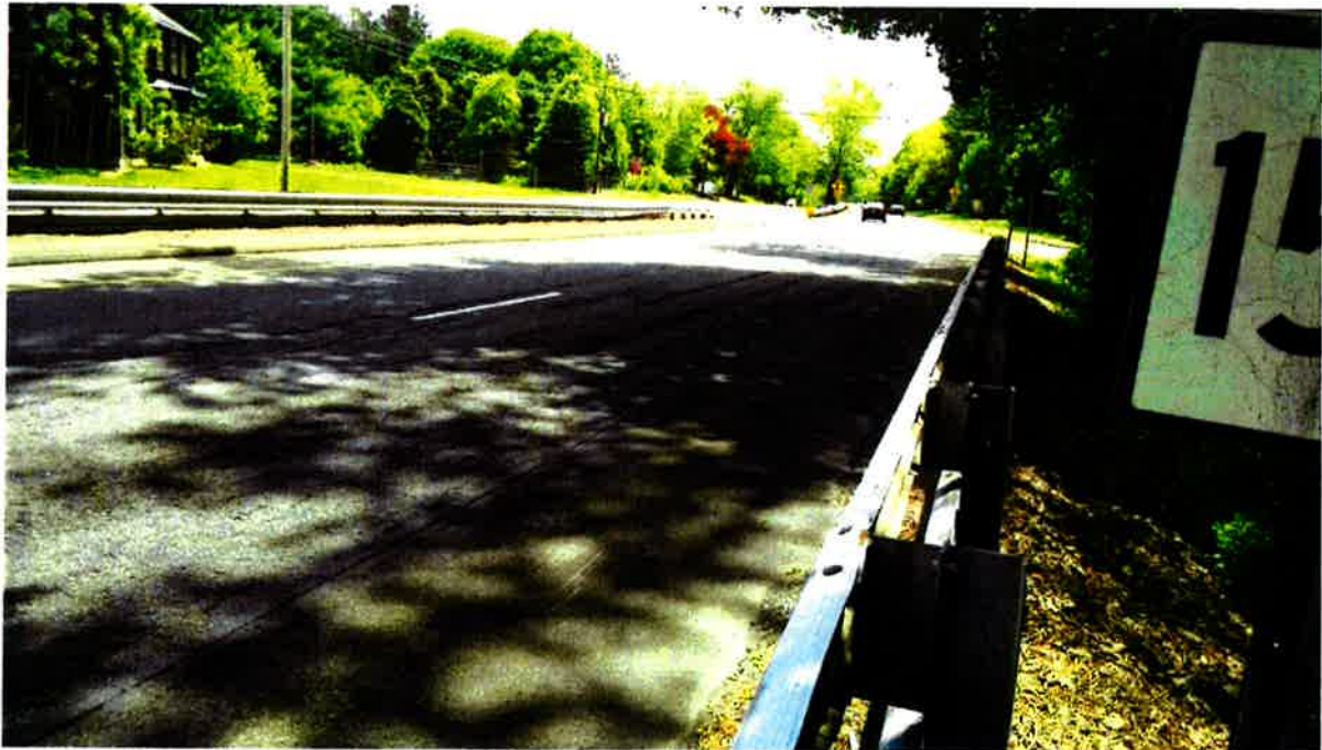
10. Looking west on top of Bridge No. 00948
