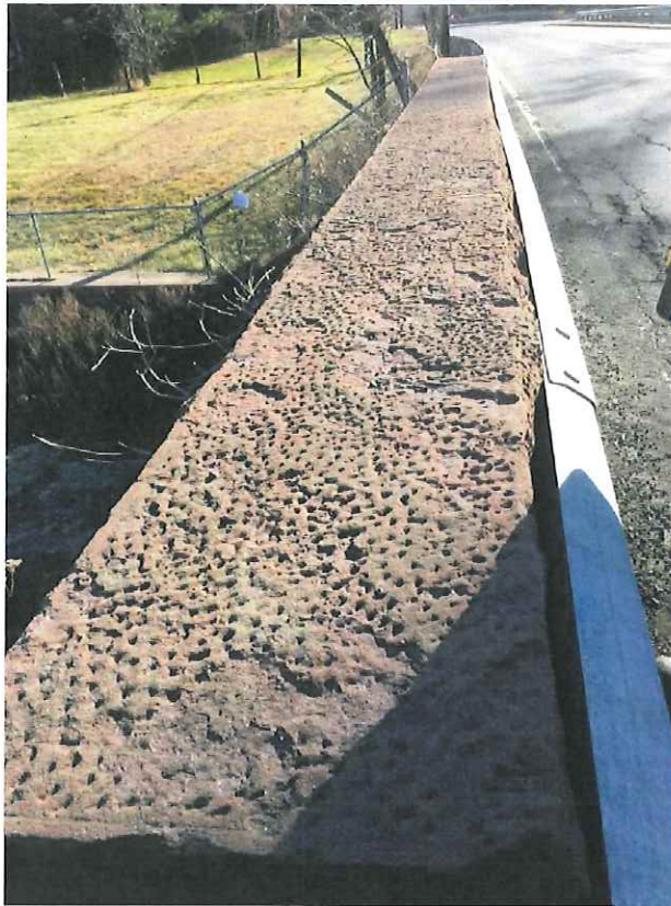
Image 3: Capstone on north parapet of bridge with pecked marked tool patterns.
