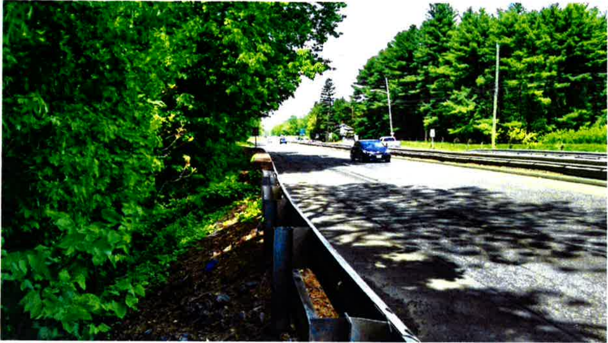
9. Looking east on top of Bridge No. 00948
