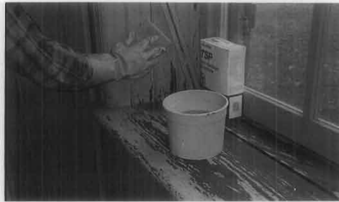
Figure 16. Washing windows and cleaning debris from window wells on a periodic basis can substantially reduce lead dust. Using water and tri-sodium phosphate (TSP or equivalent) will remove loose paint, and, after rinsing, the surface can be repainted with latex, oil/alkyd, or latex acrylic paints.
