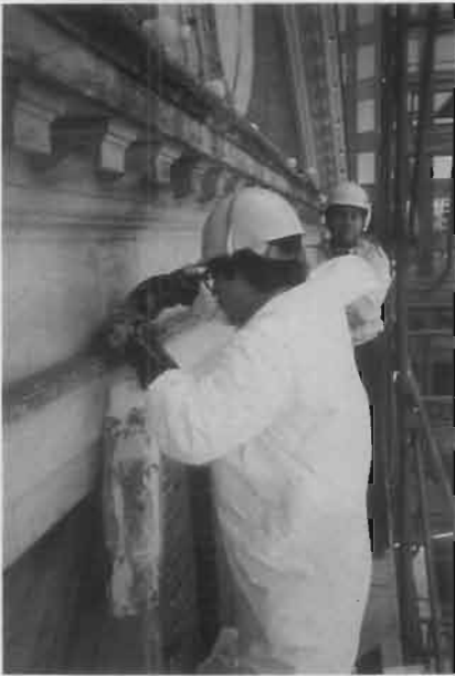
Figure 10. The choice of paint removal method will trigger various environmental controls and worker protection. The chemical poultice-type paint remover uses a paper backing that keeps the lead waste contained for proper disposal. The worker is adequately protected by a suit and gloves; for this work a respirator was not required. Local laws required containment and neutralization of any after-wash water run off. Photo: NPS Files.
