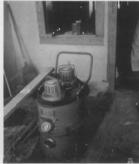
Figure 24. Historic baseboards are often bumped by brooms and vacuum cleaners, causing lead-based paint chips to fall on the floor. Shoe moldings can be added or replaced to increase protection to the baseboard itself. In this case, because the interior warranted substantial repair, simple historic board trim was replaced with new matching trim. Note the HEPA filter vacuum in the foreground. Photo: NPS file.
