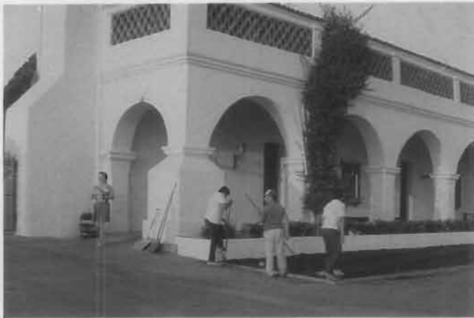
Figure 17. When historic sites are found to contain high levels of lead in bare soil — particularly around foundations — it is important to reduce the hazard without destroying significant landscapes. In many cases, contaminated soil can be removed from the foundation area and appropriate plantings or ground covers replanted in new soil. Photo: Charles A. Birnbaum, ASLA.
