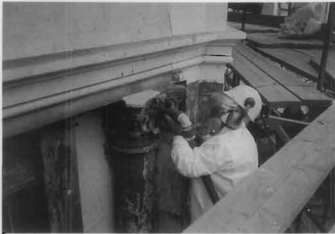
Figure 11. New methods are being developed or adapted to safely remove lead-based paint from various substrates. On this cast iron building undergoing rehabilitation for apartment units, multiple layers of lead-based paint were removed with pneumatic needle guns with vacuum attachments. Paint chips and waste containing lead-based paint were placed in 55 gallon drums for transport to a special waste site, and the workers were fully protected. The cleaned metal was primed and repainted. Photo: Building Conservation Associates, Inc.
